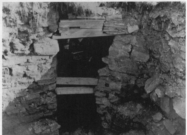
Figure 16: 'The Pap', Hillhead, broch. 'Entrance passage from inside'. Barry realised the need to photograph significant features which could not be recorded visually in any other way. This is one of several photographs which show the use of timber supports, a reminder of Barry's mining background. (C7591)
