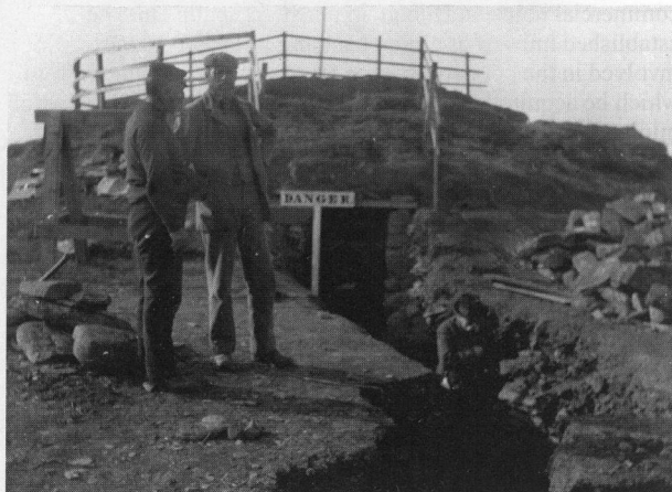
Figure 7: 'The Pap', Hillhead, broch, 1901. View towards entrance. Barry is standing in the passage to the right, with Mr Murdoch and John Nicolson to the left of the 'Danger' sign. (D5205)
