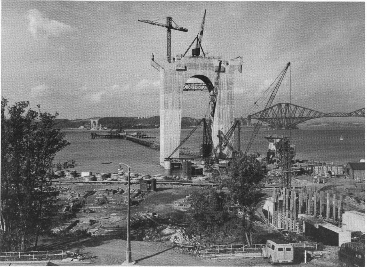
Plate 25: Forth Road Bridge: view from south overlooking the working site adjacent to South Queensferry, September 1960. The construction causeway can be seen clearly in the middle distance. The coils of temporary construction cable visible in the foreground were provided by Bruntons of Musselburgh, whose wire rope works closed in 1997 (W Ralston negative number 60/643/1) (C 87217 PO, item 122).
