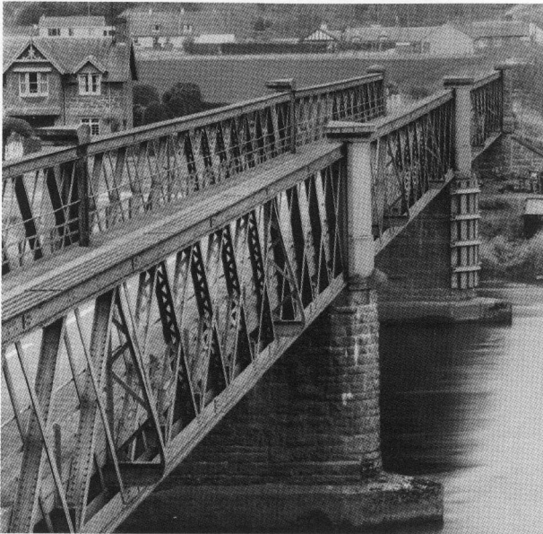
Plate 20: View from south-east of the old Victoria Bridge at Caputh (built in late 1880s), seen here prior to its replacement with a new bridge. Unconfirmed reports suggest that some of the members of this bridge were recycled from parts of the collapsed first Tay Bridge (A 80965, 1987, RCAHMS, item 94).
