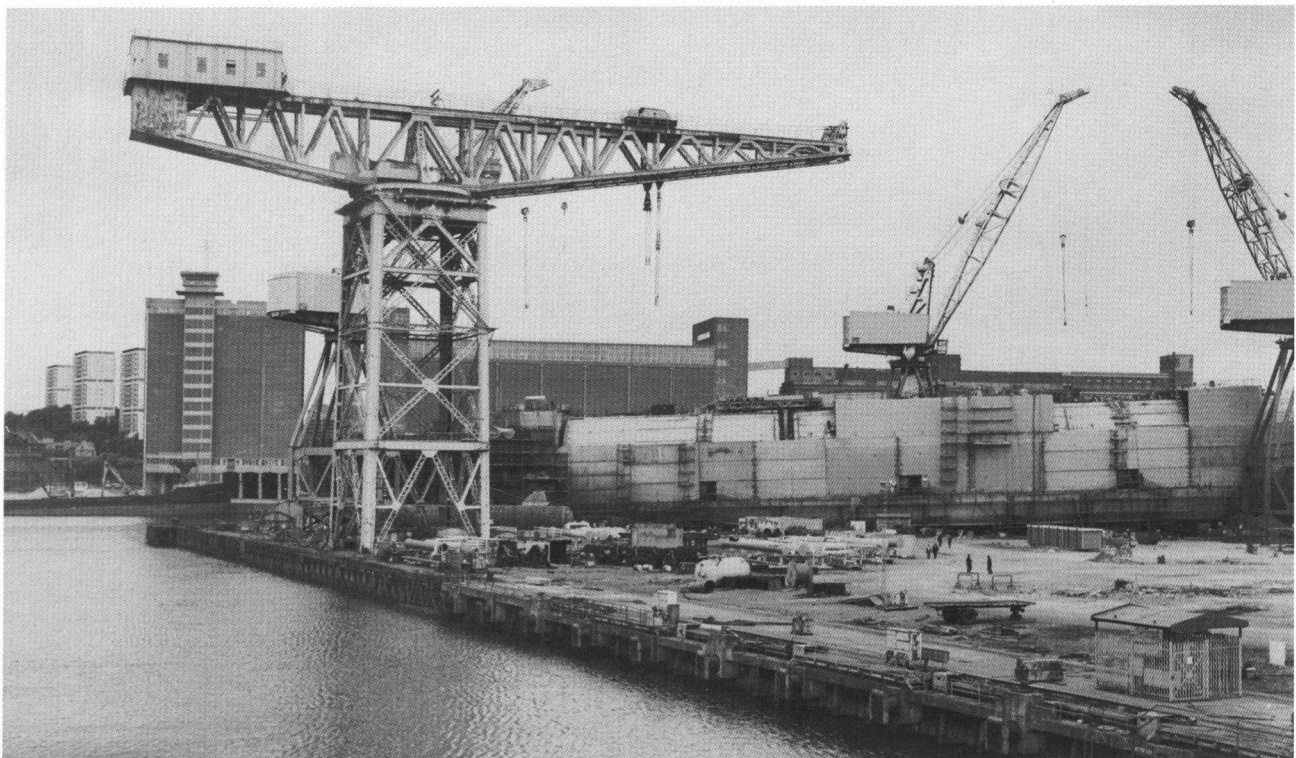
Plate 18: View from south-south-west across the fitting-out basin of the former Fairfield Shipyard in Glasgow (now Kvaerner Govan), showing the Arrol 220-ton Giant Cantilever crane (built in 1911) (B 41310, 1990, RCAHMS, item 74).
