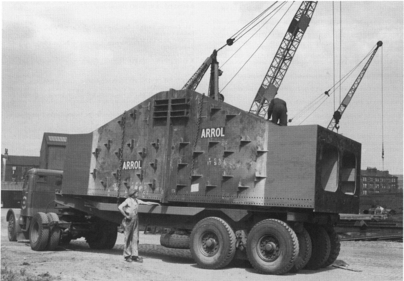
Plate 23: Forth Road Bridge: the base section of the upstream tower, North Pier, leaving Sir William Arrol and Company's works, Dalarnock, Glasgow, June 1960 (W Ralston negative number 60/355G) (C87198 PO, item 122).
