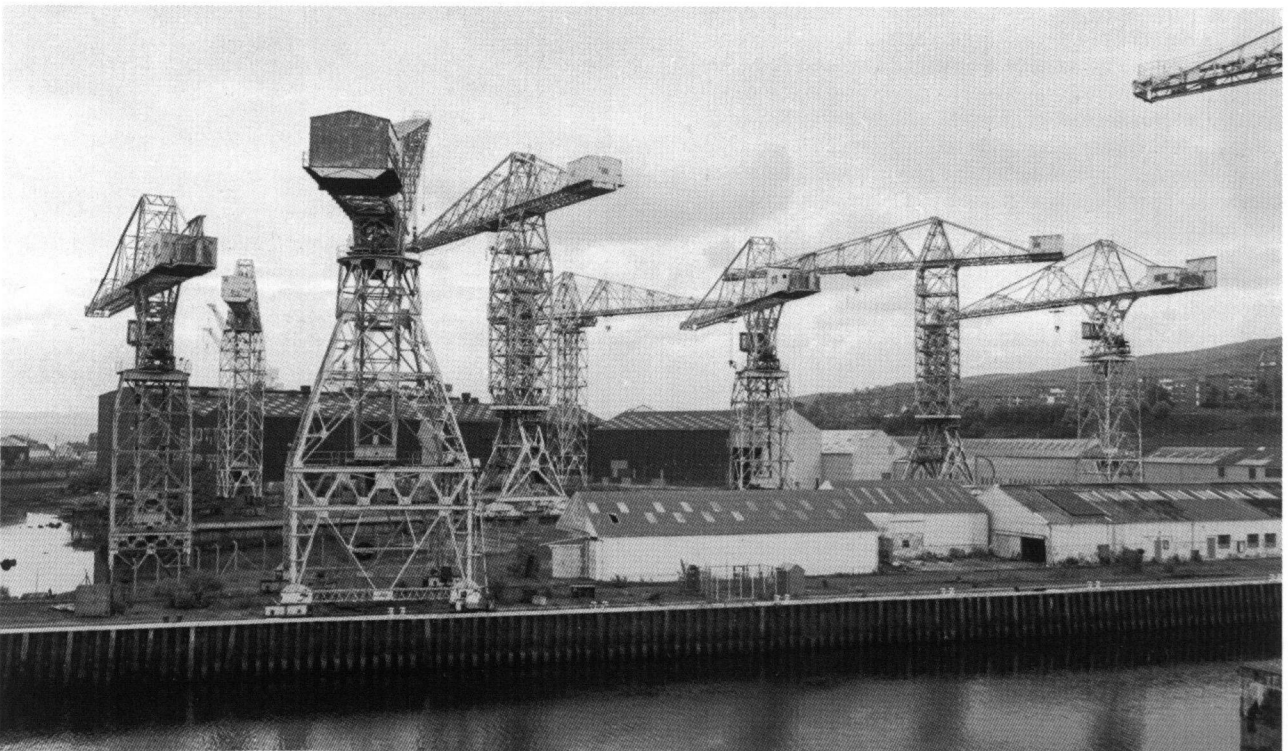
Plate 1: General view from west of the Cartburn Shipyard, Greenock, showing the large number of mostly Arrol-built cranes serving the slipways. The cranes were subsequently demolished (A 61945, 1987, RCAHMS).
