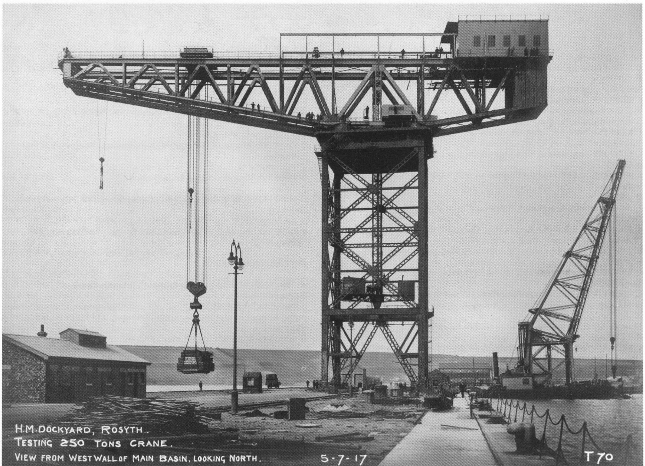
Plate 11: 'HM Dockyard, Rosyth Testing 250 Tons Crane... 5.7.17'. The acquisition of the Parkhead Crane Works in 1910 allowed Arrol not only to design and build such cranes, but also to provide the machinery (C 87838 PO, item 32).
