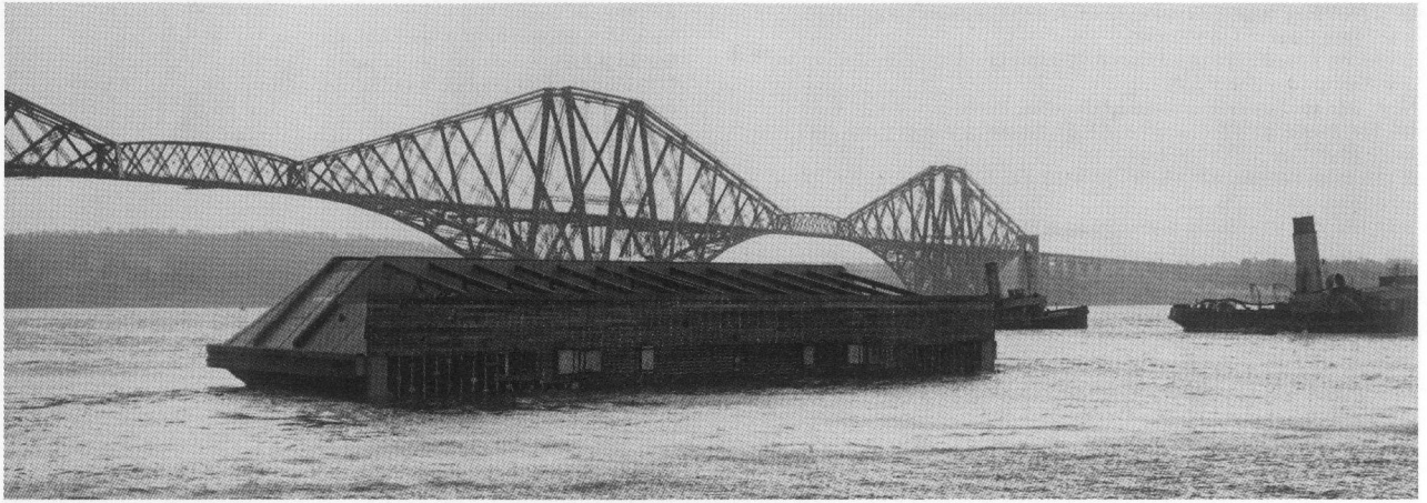
Plate 10: Rosyth Dockyard. Tugs taking charge after the launch of one of the seven sliding dock caissons designed and built by Arrol for the Admiralty, en route from the construction site at North Queensferry to Rosyth Dockyard, c. 1914. Latterly, the caissons were built at Rosyth because mooring in the River Forth caused obstruction to shipping as wartime river traffic increased (C87142 PO, item 32). In the background, the Forth Railway Bridge, Sir William Arrol and Company's most famous project (1882-1890).
