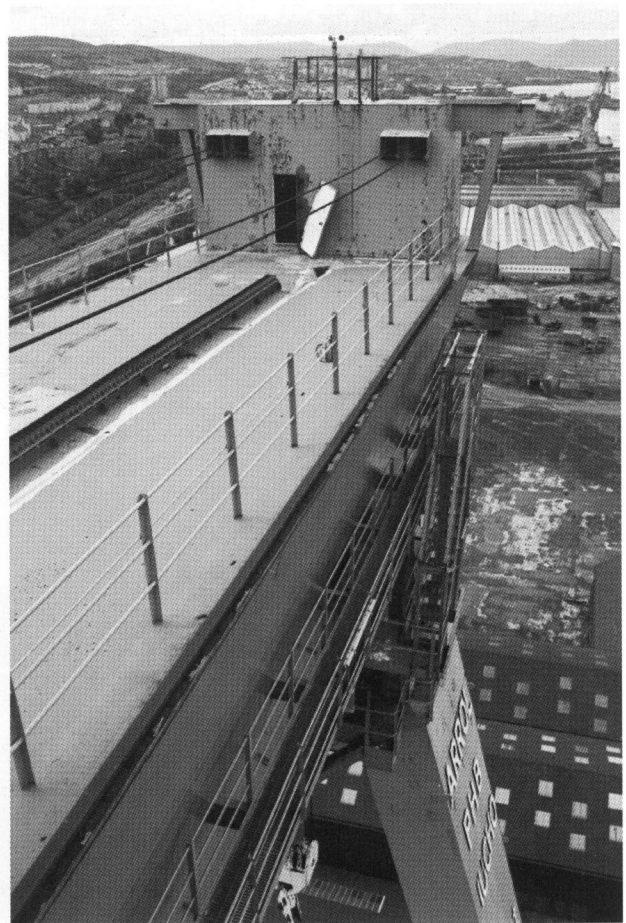
Plate 3: View from east on top of the north-west end of the 225-ton Goliath Crane at the Glen Shipyard, Port Glasgow, with Greenock shipyards visible below (B 45032, 1990, RCAHMS).
