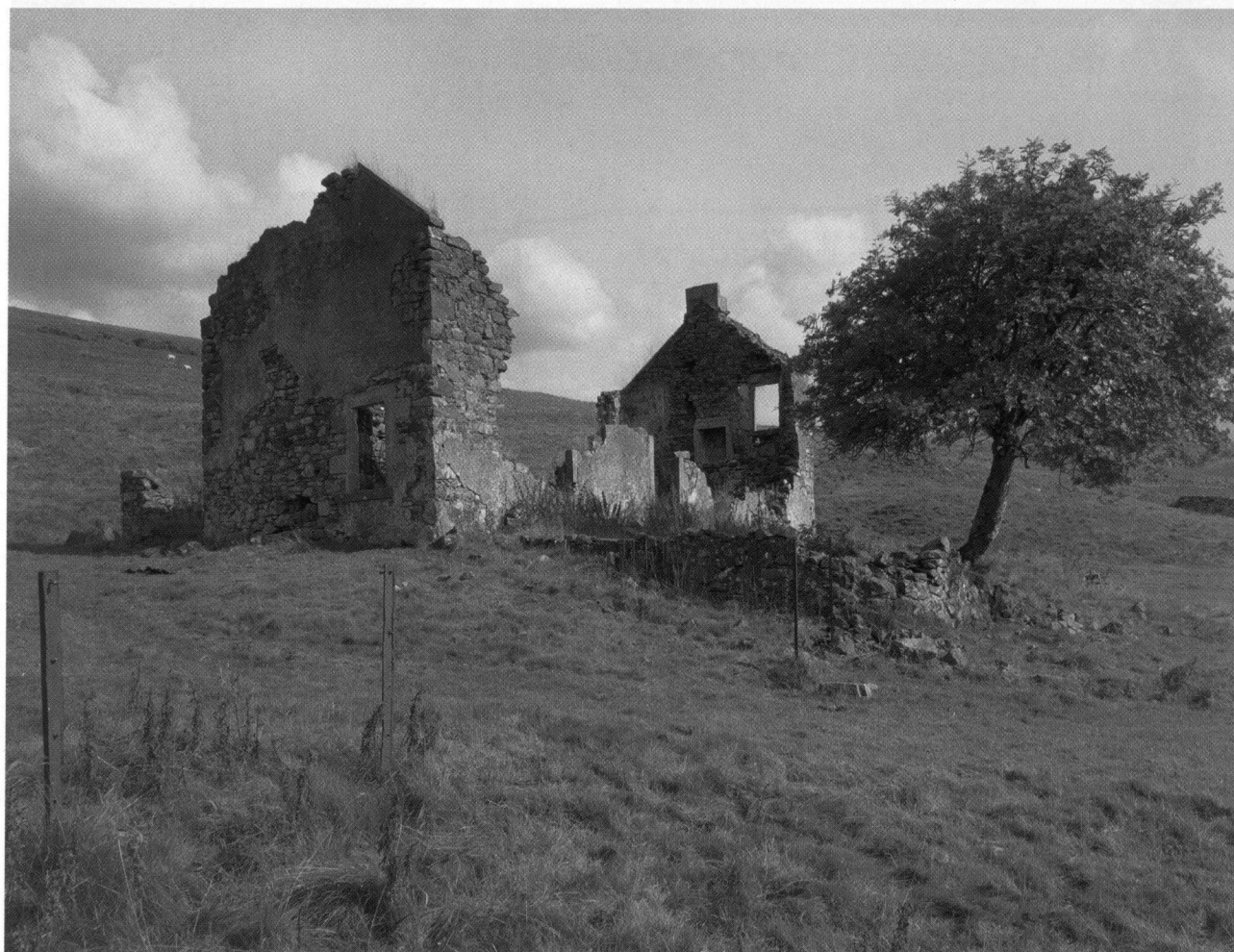
Fig.34 By the 1860s, Jerah was the only functioning farmstead left in the glen, and the ruined shell of its mid 19 th -century farmhouse, abandoned in the mid 20 th -century, can be seen in this ground view taken from the south-west. SC 579459
