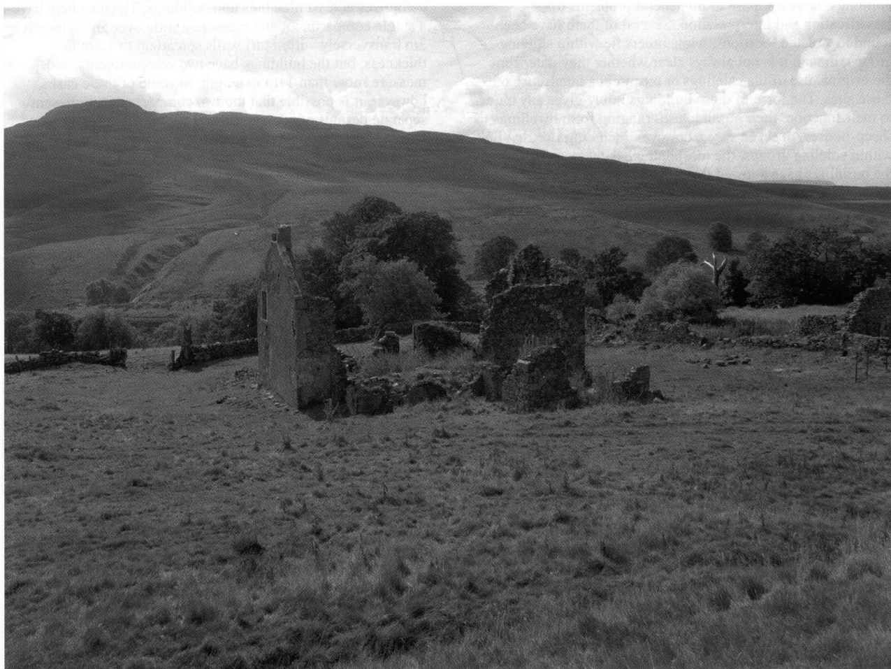
Fig.22 The shattered shell of the 19 th century farmhouse at Jerah, seen from the north and looking to Dumyat beyond. SC 585584
