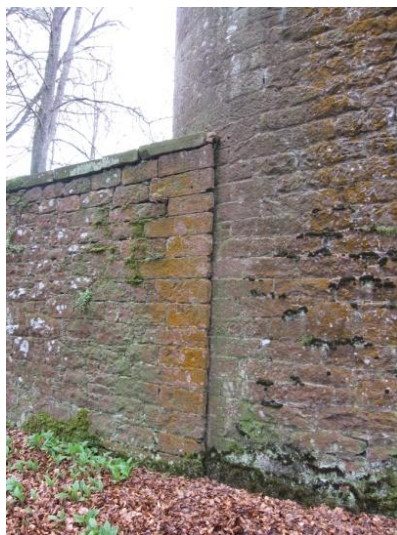
Spur wall join to observatory
