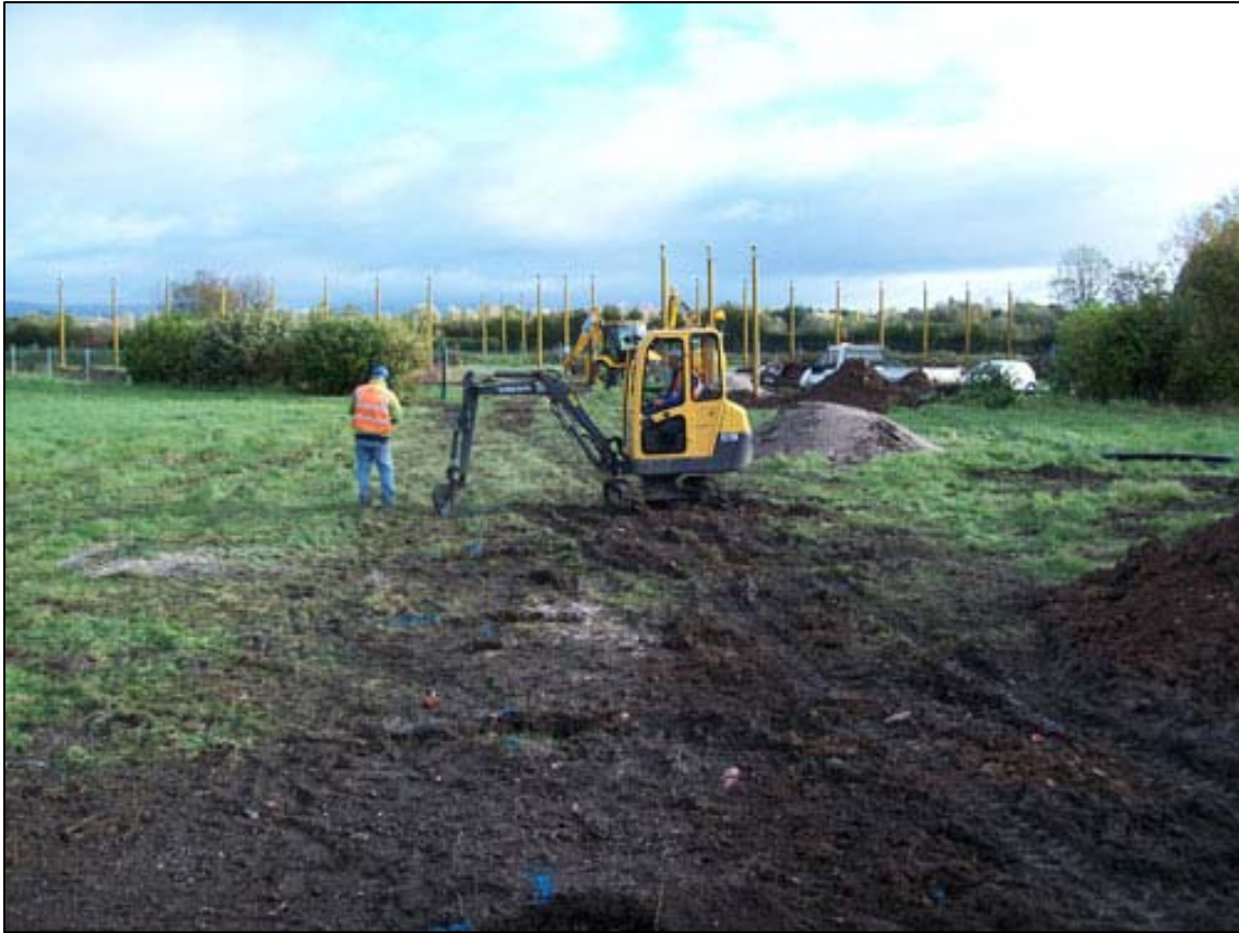
Figure 6a: Excavating for fence line
