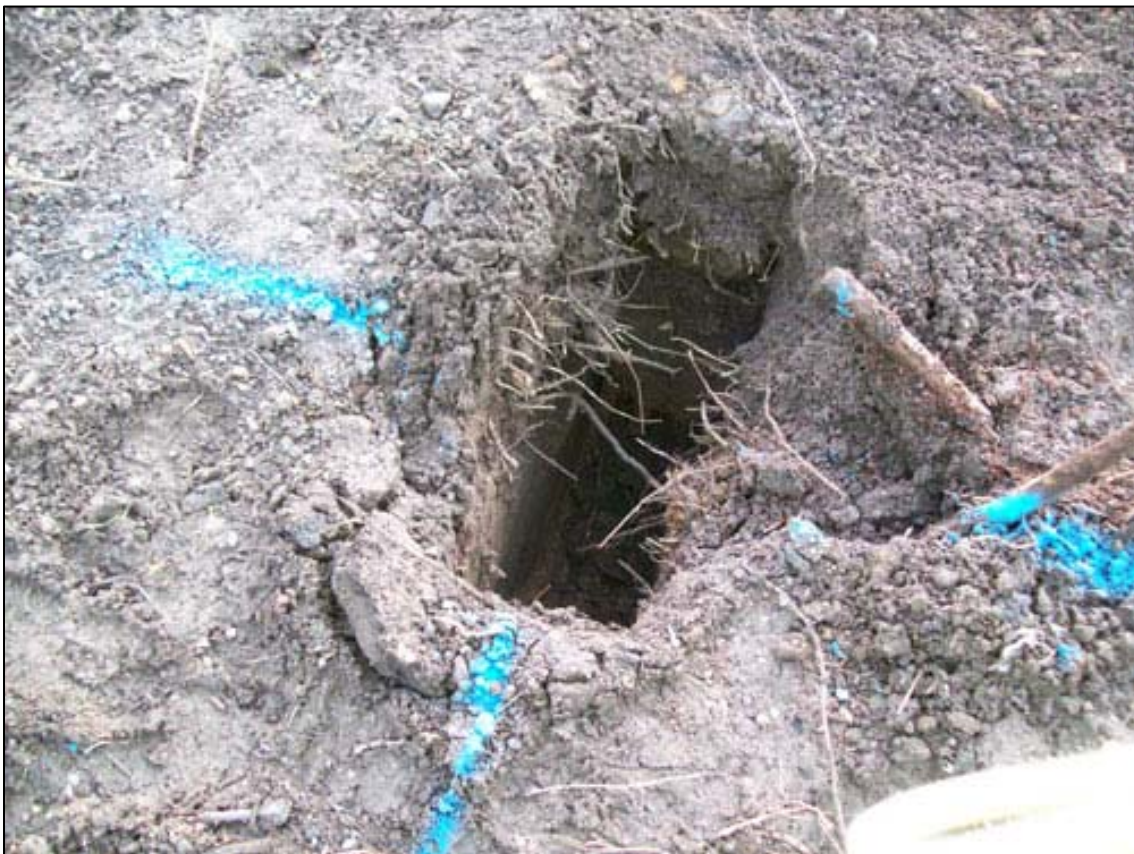
Figure 6b: Pit for fence line
