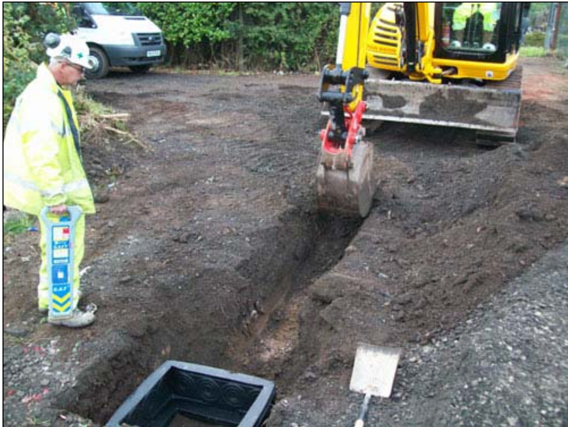
Figure 3a: Inspection hatch and track NE of graveyard
