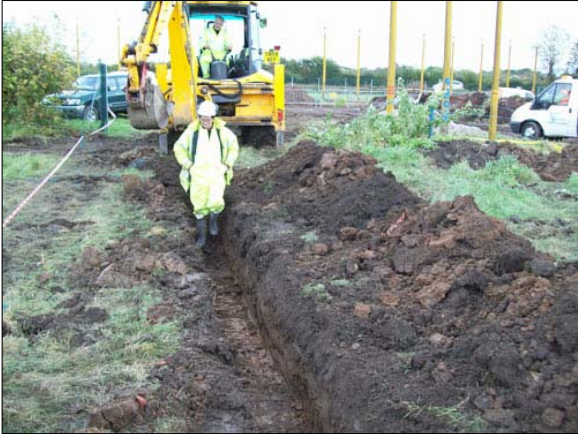
Figure 8a: Track at northern boundary of scheduled area
