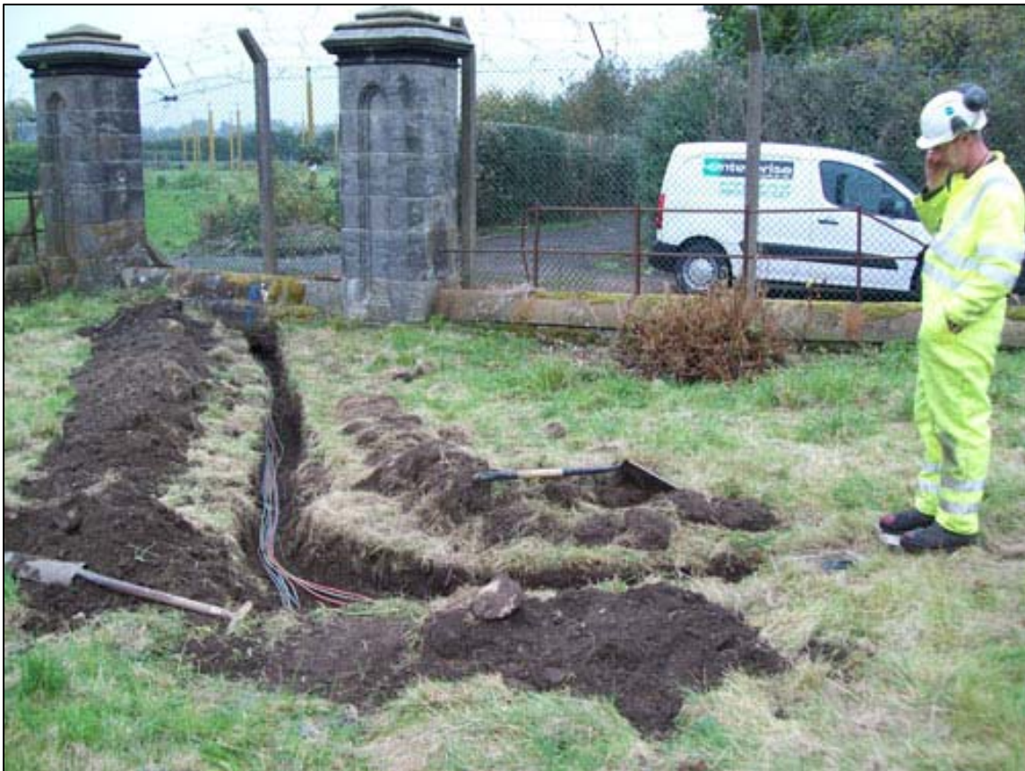
Figure 2b: Excavation in graveyard (looking north-east)
