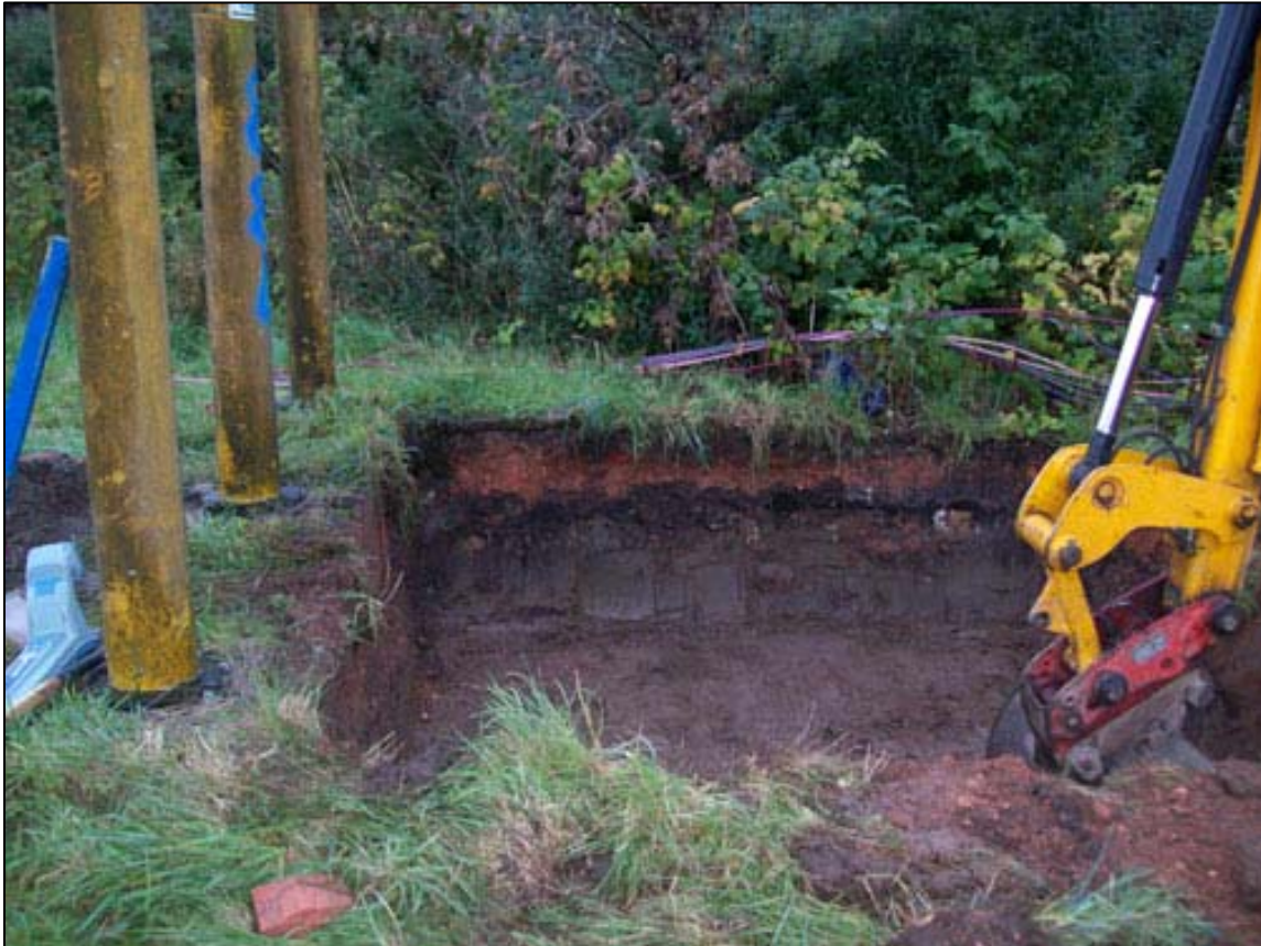
Figure 5b: Pit for new lighting base
