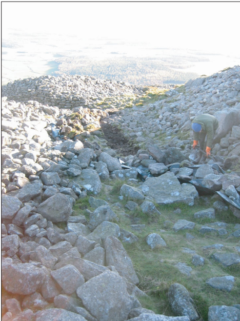
Plate 4: Section 3 of path. Looking E.
