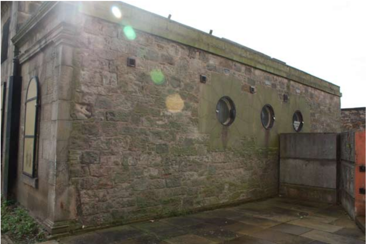
Illus 22 Western guardhouse, circular windows in west wall
