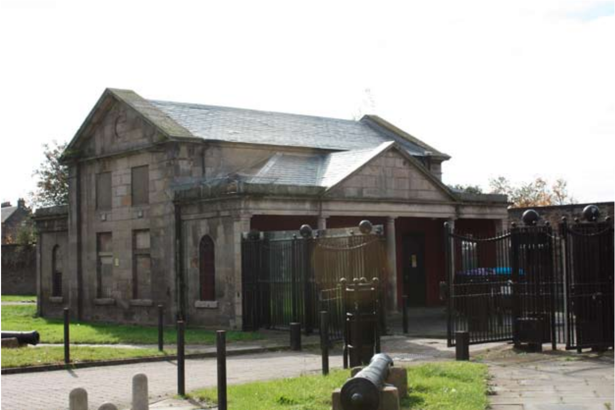
Illus 15 Eastern guardhouse looking SE
