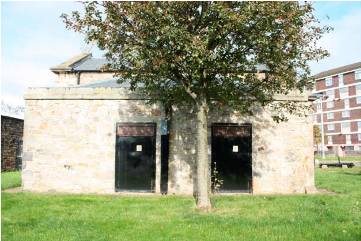
Illus 16 Eastern guardhouse, E elevation showing blocked doorways
