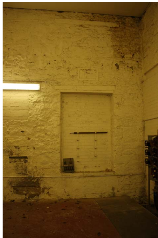
Illus 19: Eastern guardhouse, Room 1, blocked windows in north wall
