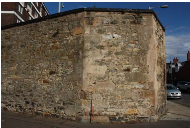
Illus 11: Boundary Wall , Portland Street
