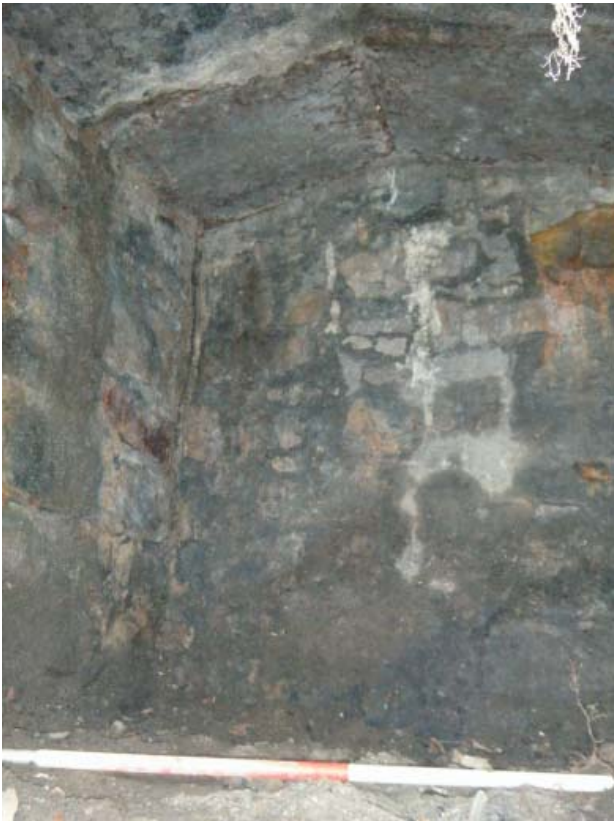
Illus 10 Cellar 20, internal view
