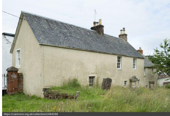
Fig. 1: The East elevation of the Smithy. Note the blind wall on the first floor above the Smithy. Kirk House is the north half of this range (right)
