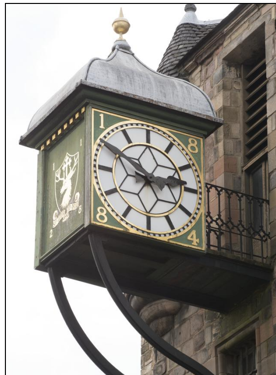
Figure 109: Detail of clock dated 1884, 2014 (DP190173 ©Crown copyright HES)
