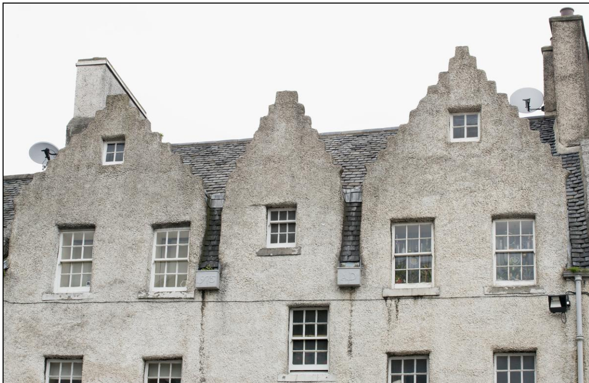
Figure 174: Detail of crowstepped gables on front elevation of 5 Canongate , 2014 (DP188699 ©Crown copyright HES)
