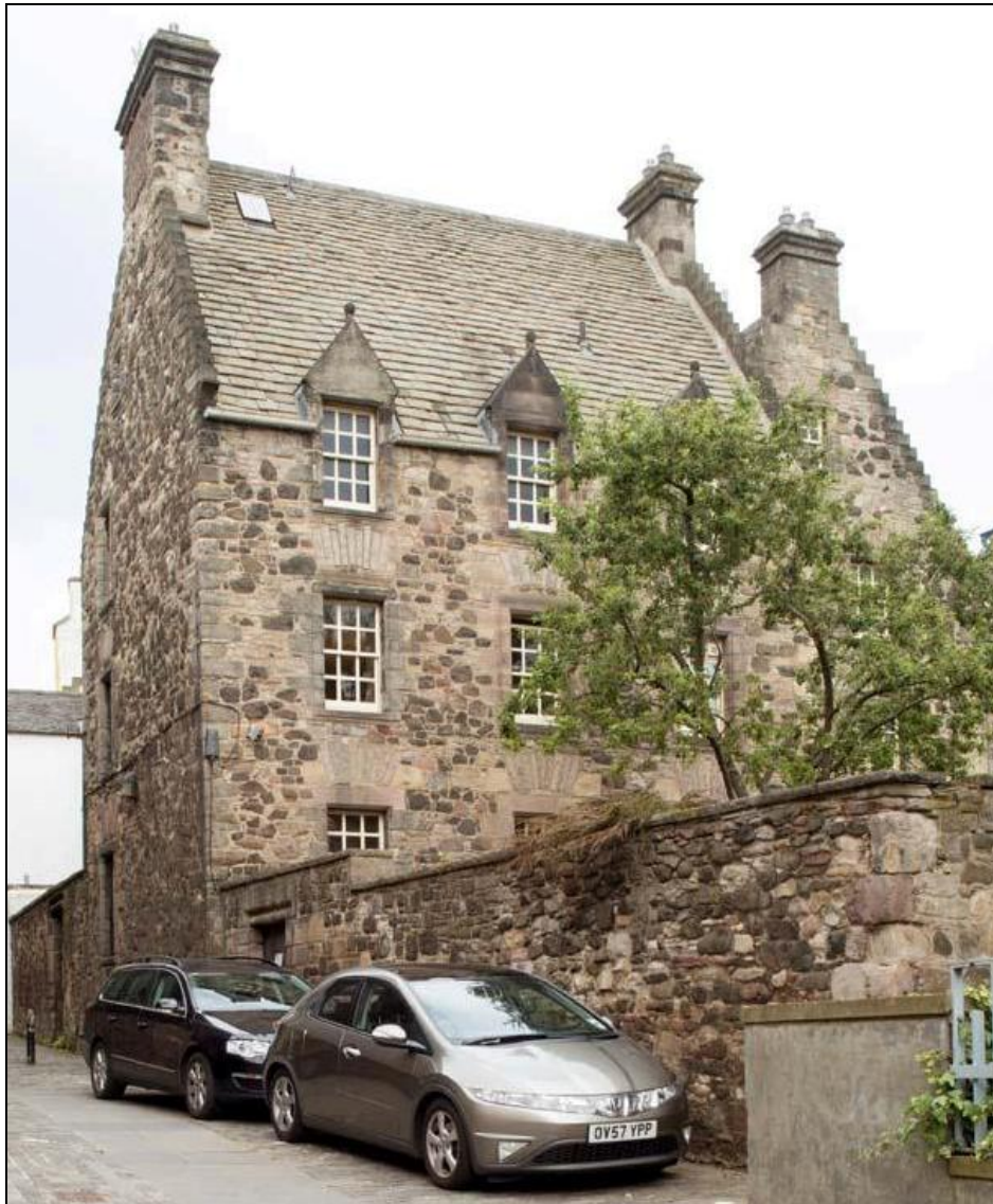
Figure 102: View of Acheson House , Bakehouse Close, from south-west, 2013 (DP158589 ©Crown copyright HES)
