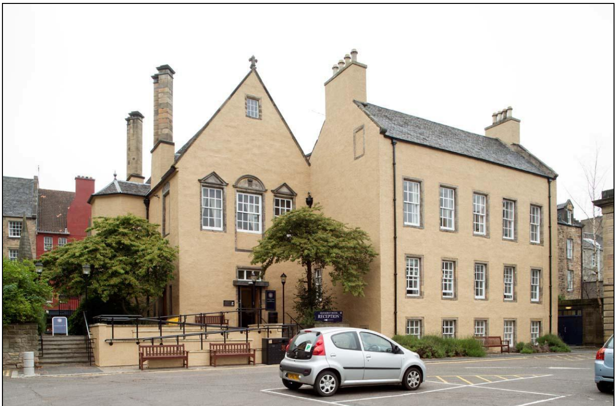
Figure 118: View of Moray House, from south, 2013 (DP160519 ©Crown copyright HES)
