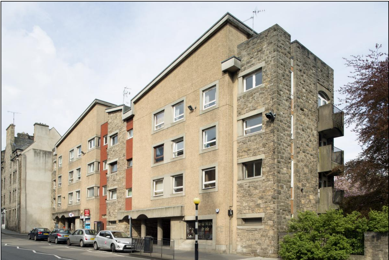
Figure 172: View of 97-103 Canongate , from south-east, 2014 (DP188670 ©Crown copyright HES)
