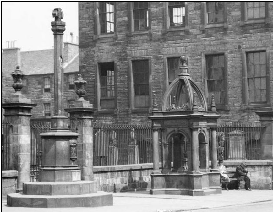
Figure 123: View of Burgh Cross and Home Fountain , 1948 (copied 1999) (SC487937 ©Crown copyright HES)
