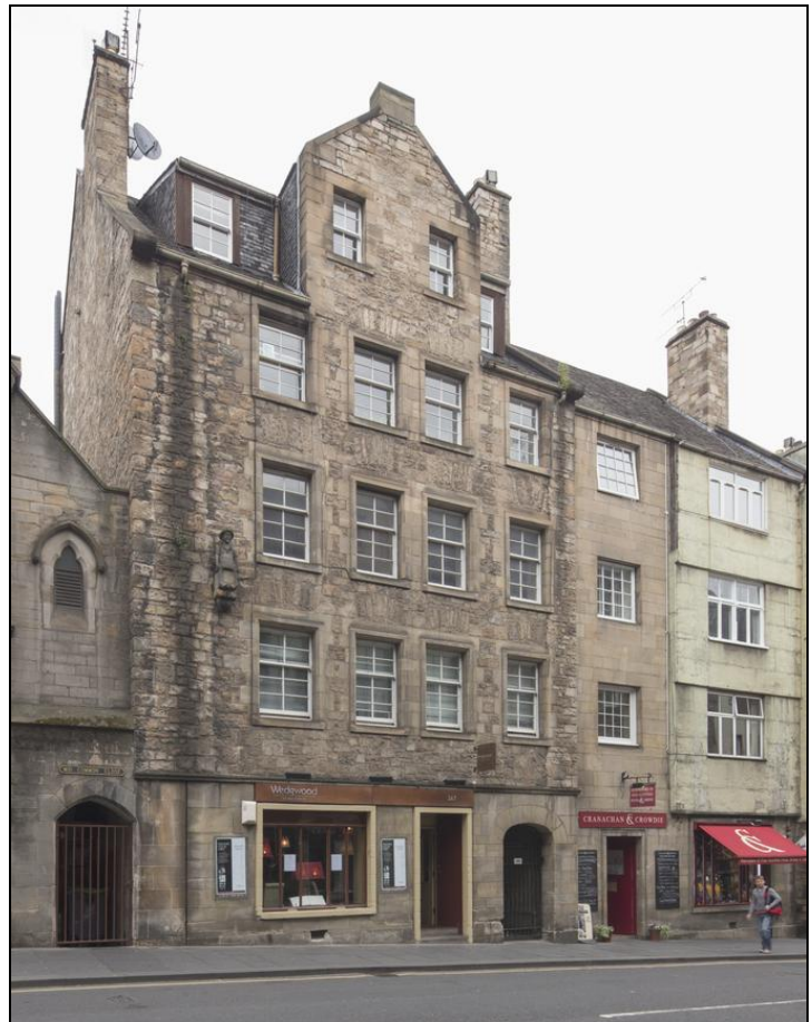
Figure 167: View of Morocco Land, 265-7 Canongate, from south-west, 2014 (DP190154 ©Crown copyright HES)
