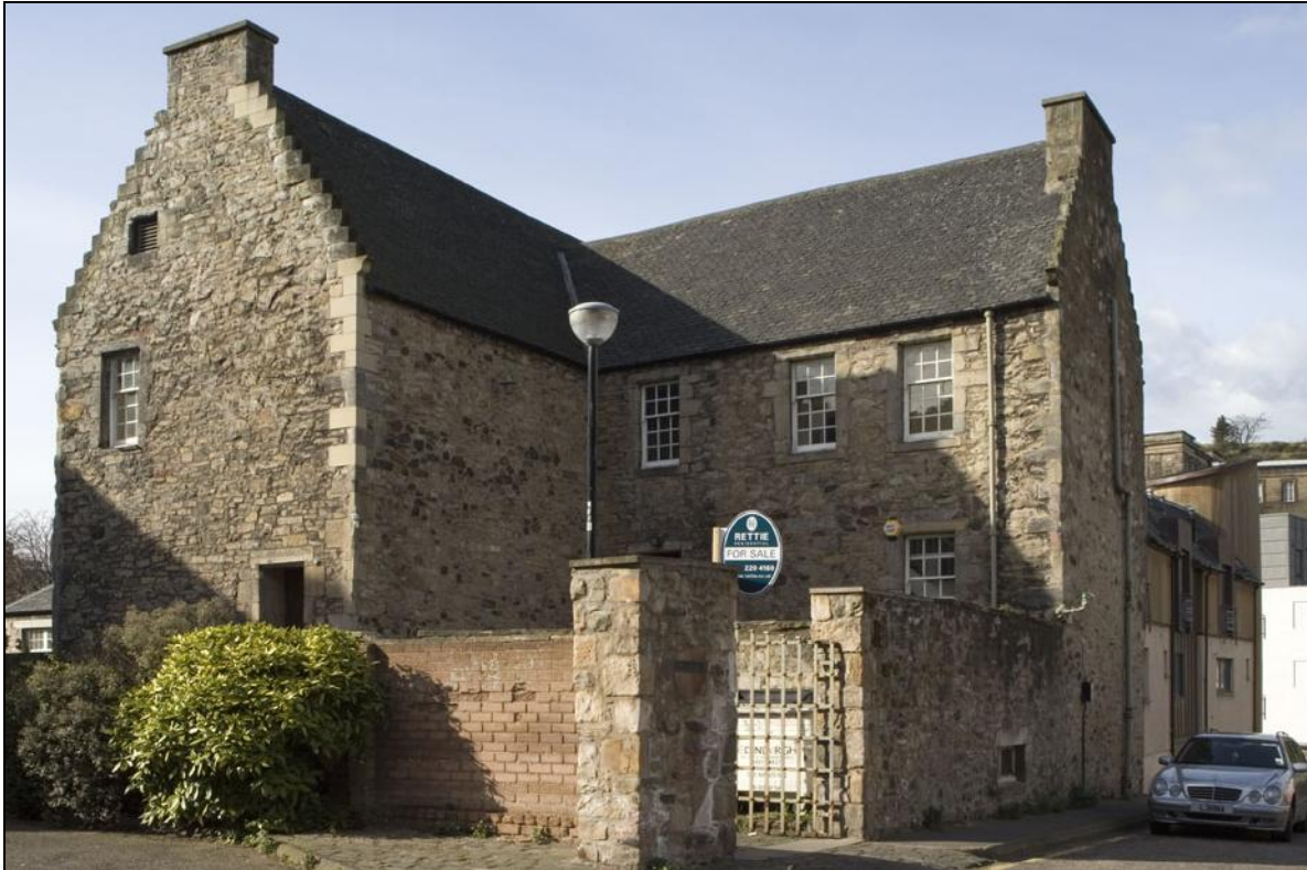
Figure 132: View of Panmure House, 129 Canongate , from south-east, 2008 (DP039169 ©Crown copyright HES)
