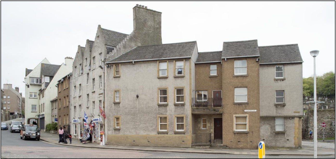
Figure 180: View of 5 and 11-15 Canongate/Robertson's Court, from east, 2014 (DP188702 ©Crown copyright HES)
