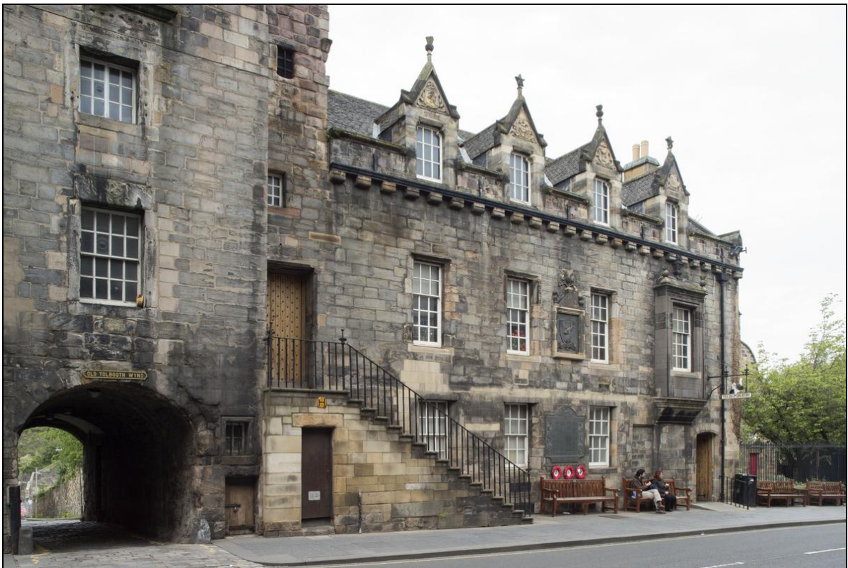
Figure 104: View of eastern section of Canongate Tolbooth with forestair, 2014 (DP190171 ©Crown copyright HES)
