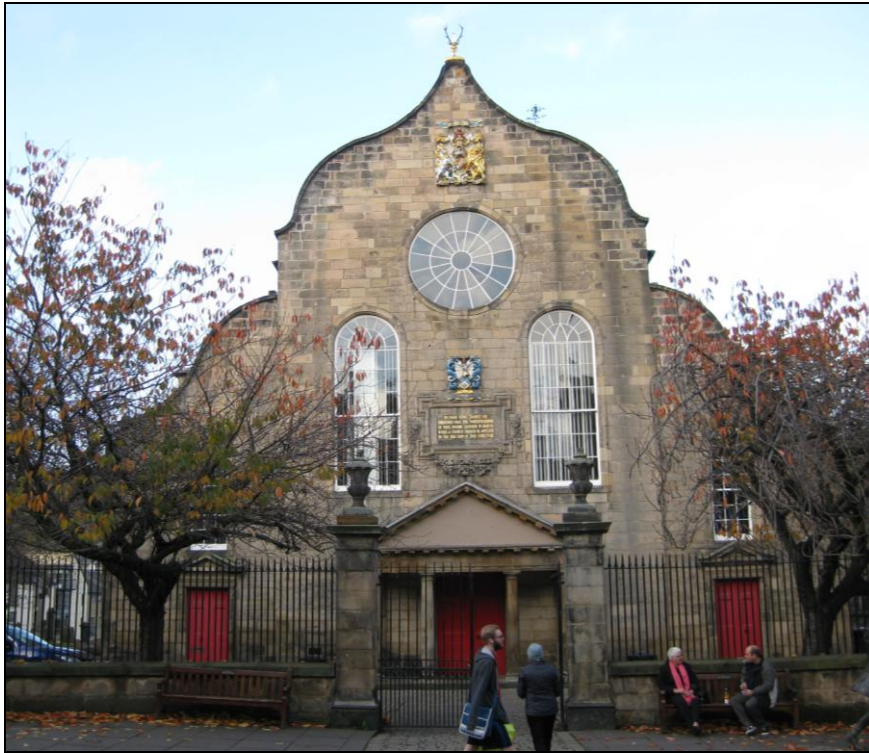
Figure 122: View of Canongate Kirk , from south, 2014 (DP207894 ©Crown copyright HS)
