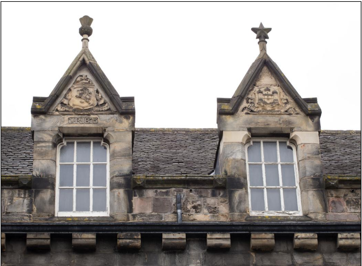
Figure 106: Detail of westernmost attic dormers at Tolbooth, 2014 (DP190175 ©Crown copyright HES)
