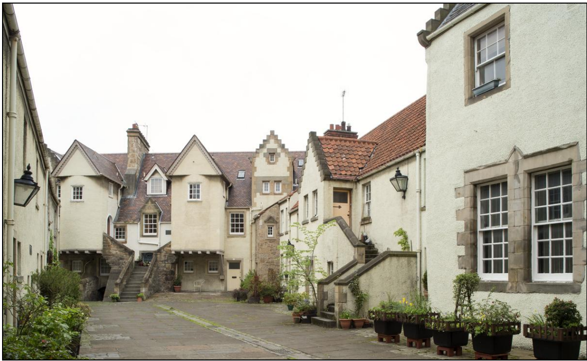
Figure 111: View of White Horse Close, 29 Canongate , from south, 2014 (DP188691 ©Crown copyright HES)
