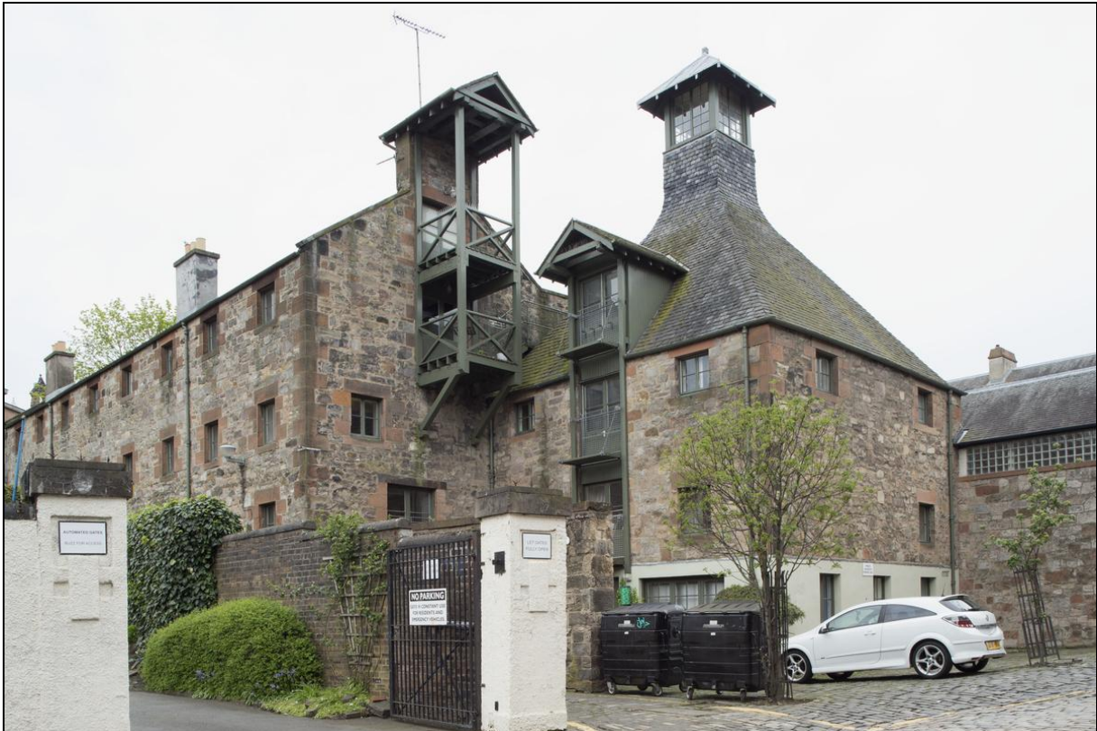
Figure 258: View of Balmoral Brewery malting, converted to housing, from north-east, 2013 (DP188706 ©Crown copyright HES)
