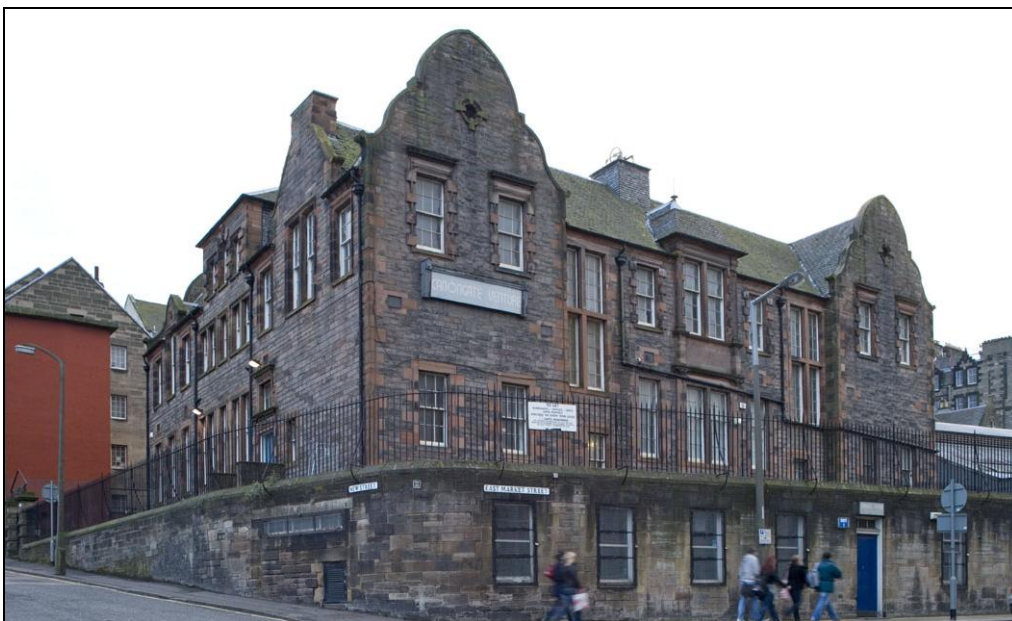
Figure 232: View of former North Canongate School on New Street/East Market Street, from north-east, 2008 (DP050335 ©Crown Copyright HES)
