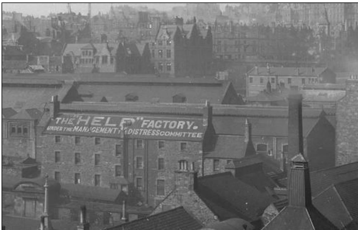
Figure 223: View of former workhouse and hospital operating as 'The HELP Factory', c.1906 (copied 2014), with the roofline of part of Calton Hill Brewery in the foreground and the gasworks in background (Scottish Gas Collection, SC1432909 ©Crown copyright HES)
