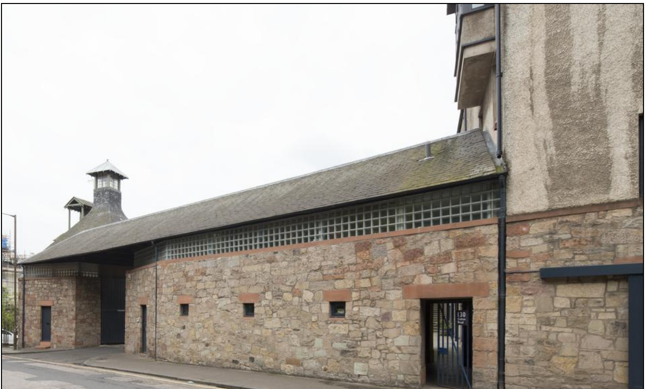
Figure 255: View of Calton Road elevation of former maltings, 136-8 Calton Road , from north-west, 2013 (DP188708 ©Crown Copyright HES)
