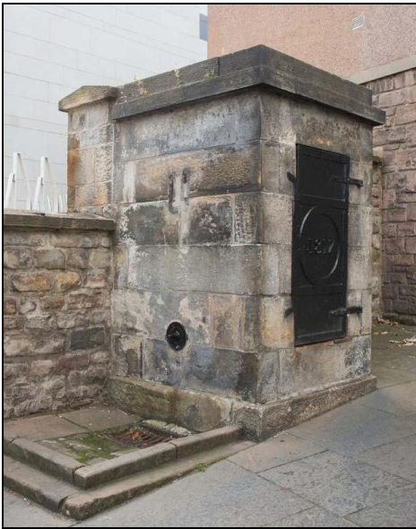
Figure 69: View of Wellhead, Queensberry House, 64 Canongate , from north, 2013 (DP161337 ©Crown copyright HES)
