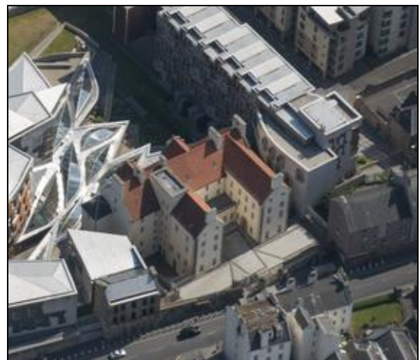
Figure 56: Aerial view of Scottish Parliament , showing roofing materials, 2014 (DP193138 ©Crown copyright HES)
