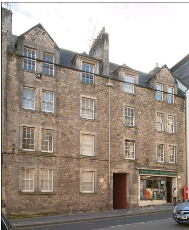
Figure 28: View of 106 Canongate , from north, 2013 (DP161398 ©Crown copyright HES)
