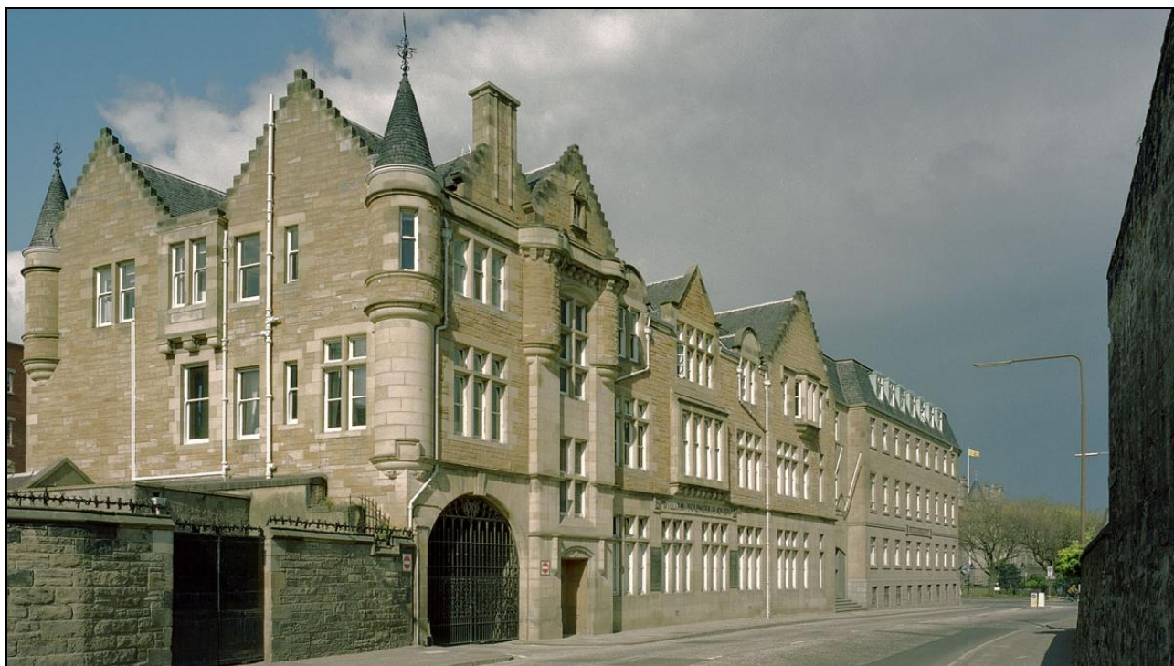
Figure 77: View of Holyrood Road elevation of Abbey Brewery , 1998 (copied 2003) (SC801757 ©Crown copyright HES)
