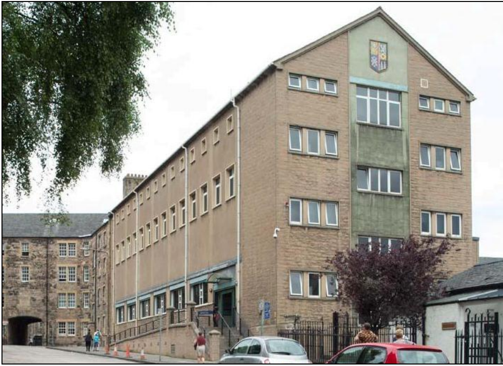
Figure 35: View of Dalhousie Land , St John Street, from south, 2013 (DP160516 ©Crown copyright HES)
