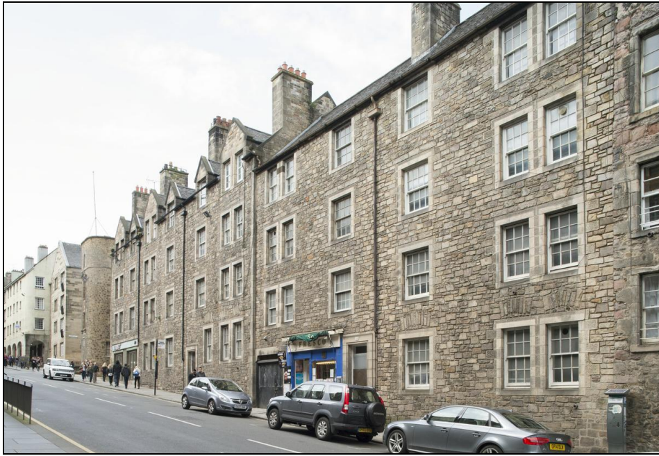
Figure 30: View of 221-9 Canongate , from south-east, 2014 (DP190164 ©Crown copyright HES)
