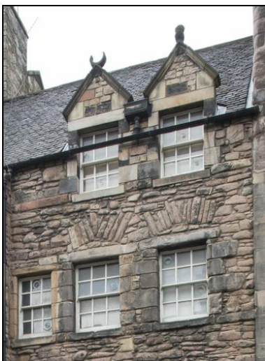
Figure 55: Detail of windows at 167-9 Canongate , 2014 (DP190170 ©Crown copyright HES)
