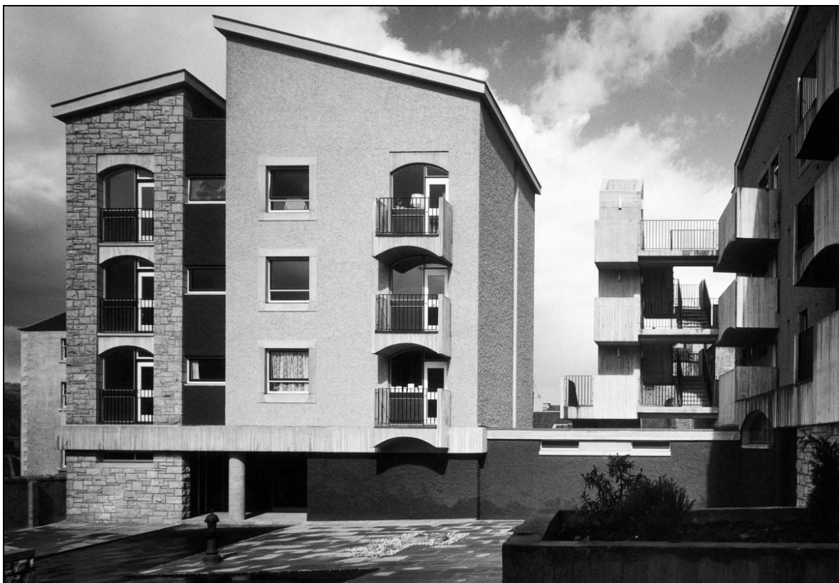
Figure 40: View of courtyard at 3 Brown's Close , from south-west, 1969 (copied 2006) (Sir Basil Spence Archive, SC1031107 ©Crown copyright HES)
