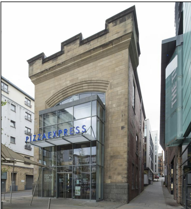
Figure 81: View of former clock tower from Holyrood Brewery at 111 Holyrood Road , 2014 (DP188516 ©Crown copyright HES)
