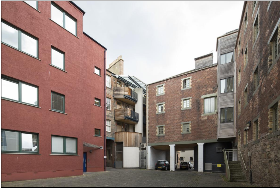
Figure 46: View of Cooper's Close, 114-120 Canongate , showing mixture of harling, stone, brick and timber cladding in backlands, 2014 (DP188649 ©Crown copyright HES)
