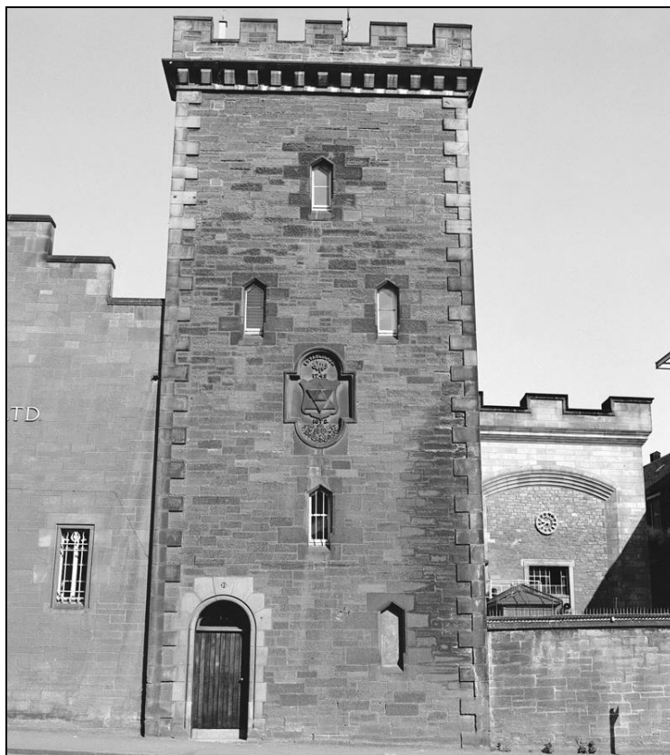
Figure 76: View of tun room and clock tower of Holyrood Brewery , Holyrood Road, 1977 (copied 2000) (John R Hume Collection, SC510189 ©Crown copyright HES)
