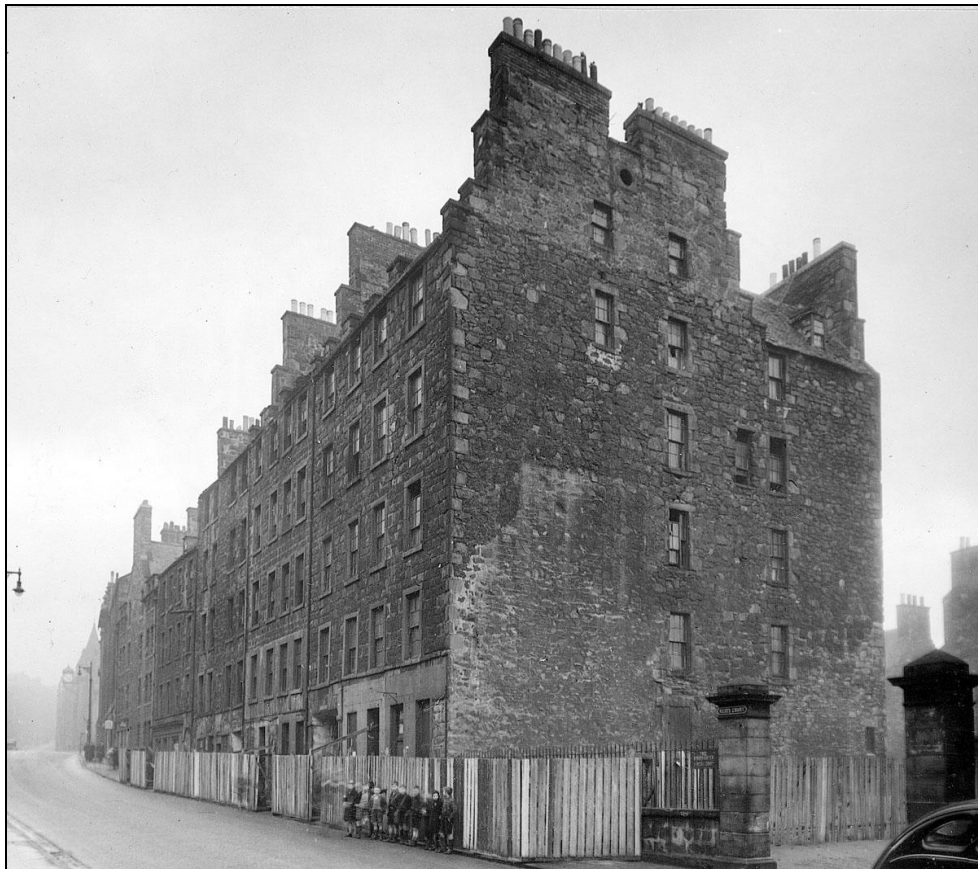
Figure 38: View of 101-21 Canongate , from east, 1948 (copied 2003) (SC801736 ©Crown copyright HES)
