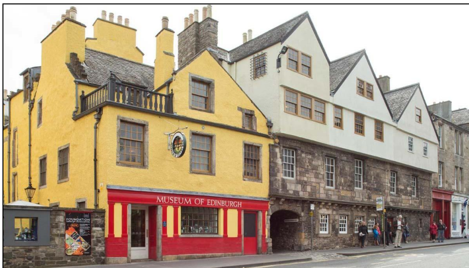
Figure 33: View of Huntly House, from north-east, 2013 (DP158595 ©Crown copyright HES)
