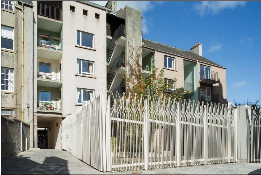
Figure 37: View of Ian G Lindsay's 1962 block of flats at 70-80 Canongate, Reid's Close, from south, 2013 (DP161359 ©Crown copyright HES)
