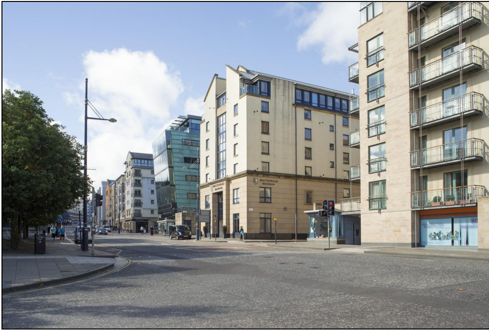
Figure 44: General view of developments along north side of Holyrood Road , looking west, 2014 (DP188504 ©Crown copyright HES)
