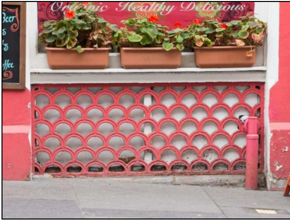
Figure 49: Detail of decorative grille below shop window at 6-8 St Mary's Street , 2013 (DP161645 ©Crown copyright HES)
