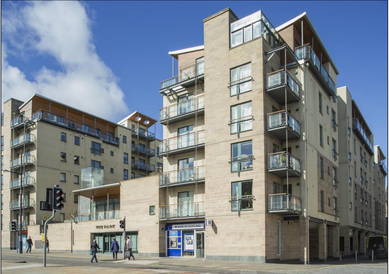
Figure 209: View of The Park, 85-91 Holyrood Road, from east, 2014 (DP188502 ©Crown copyright HES)
