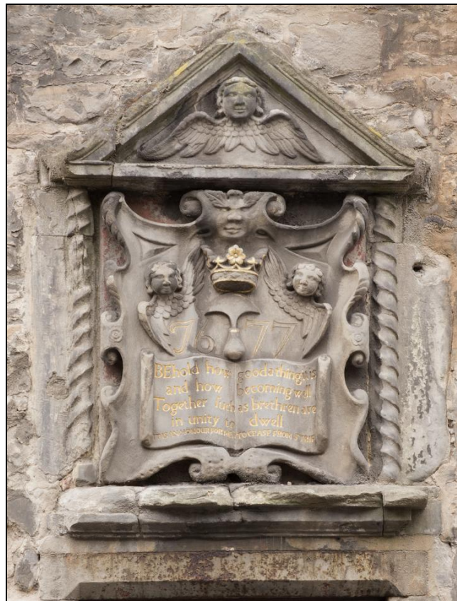
Figure 165: Detail of decorative panel above doorway at Bible Land, 185-7 Canongate, 2014 (DP190122 ©Crown copyright HES)
