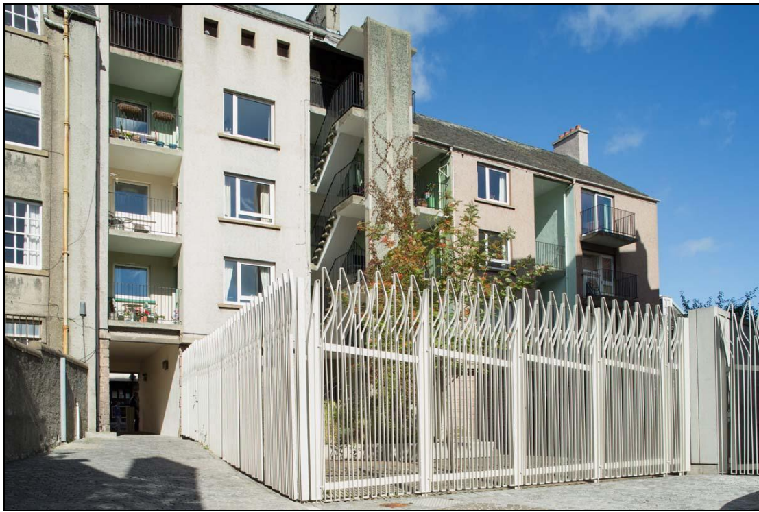
Figure 37: View of Ian G Lindsay's 1962 block of flats at 70-80 Canongate, Reid's Close, from south, 2013 (DP161359 ©Crown copyright HES)
