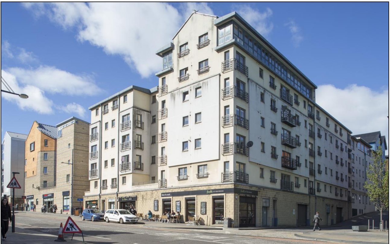
Figure 207: View of Parkgate, 63-7 Holyrood Road, from south-east, 2014 (DP188508 ©Crown copyright HES)
