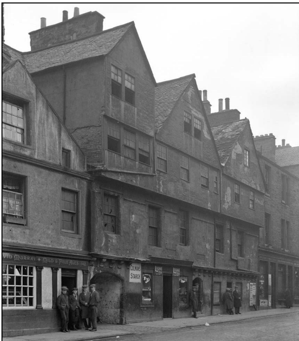
Figure 31: View of Huntly House , prior to restoration, c.1930 (copied 2008) (B C Clayton Collection, SC1122000 ©Crown copyright HES)
