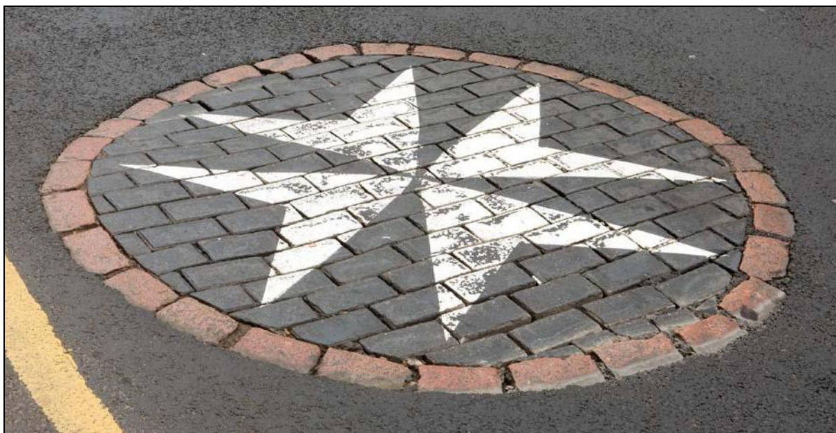
Figure 130: View of St John's Cross on the Canongate roadway, 2013 (DP160532 ©Crown copyright HES)
