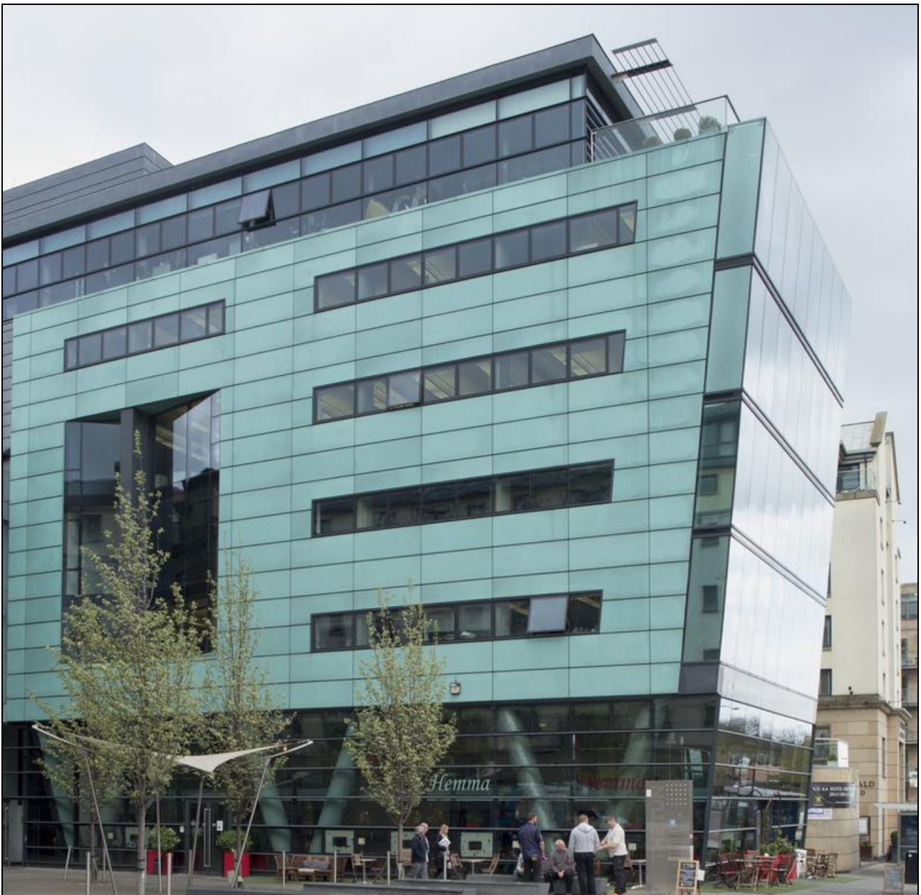
Figure 210: View of The Tun, Holyrood Road , from south-west, 2014 (DP188631 ©Crown copyright HES)
