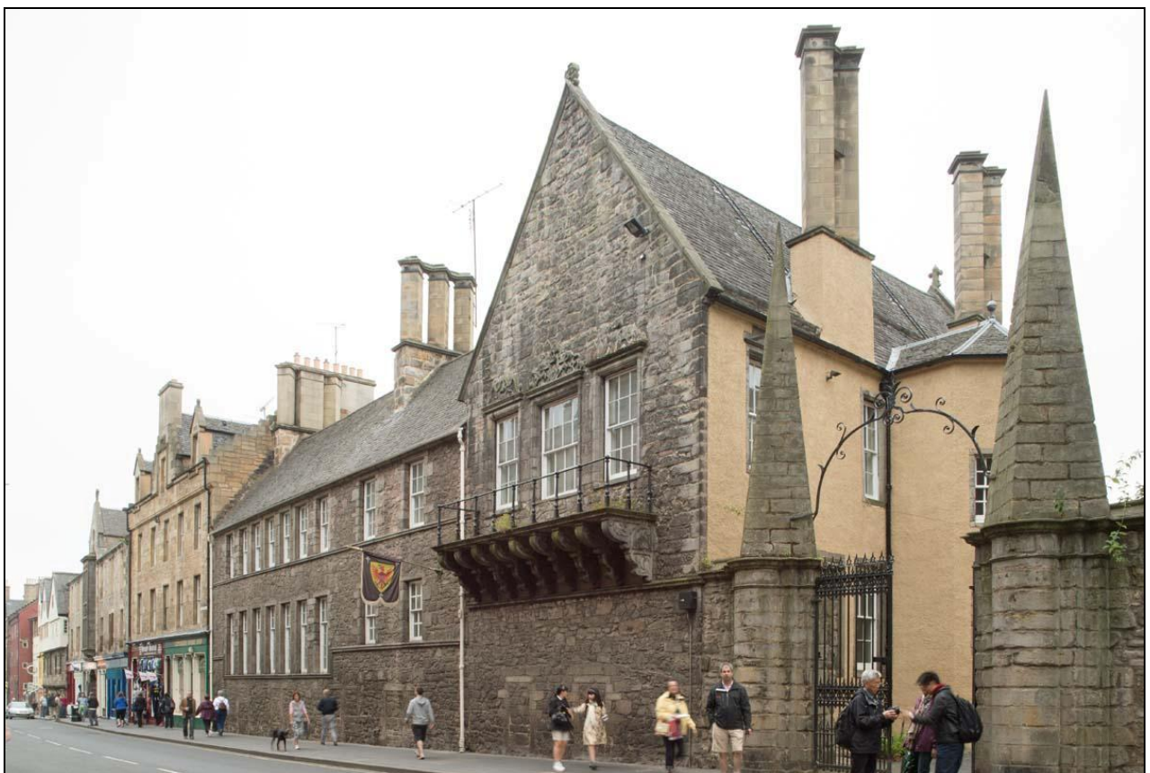
Figure 116: View of Moray House, from north-west, 2013 (DP160520 ©Crown copyright HES)
