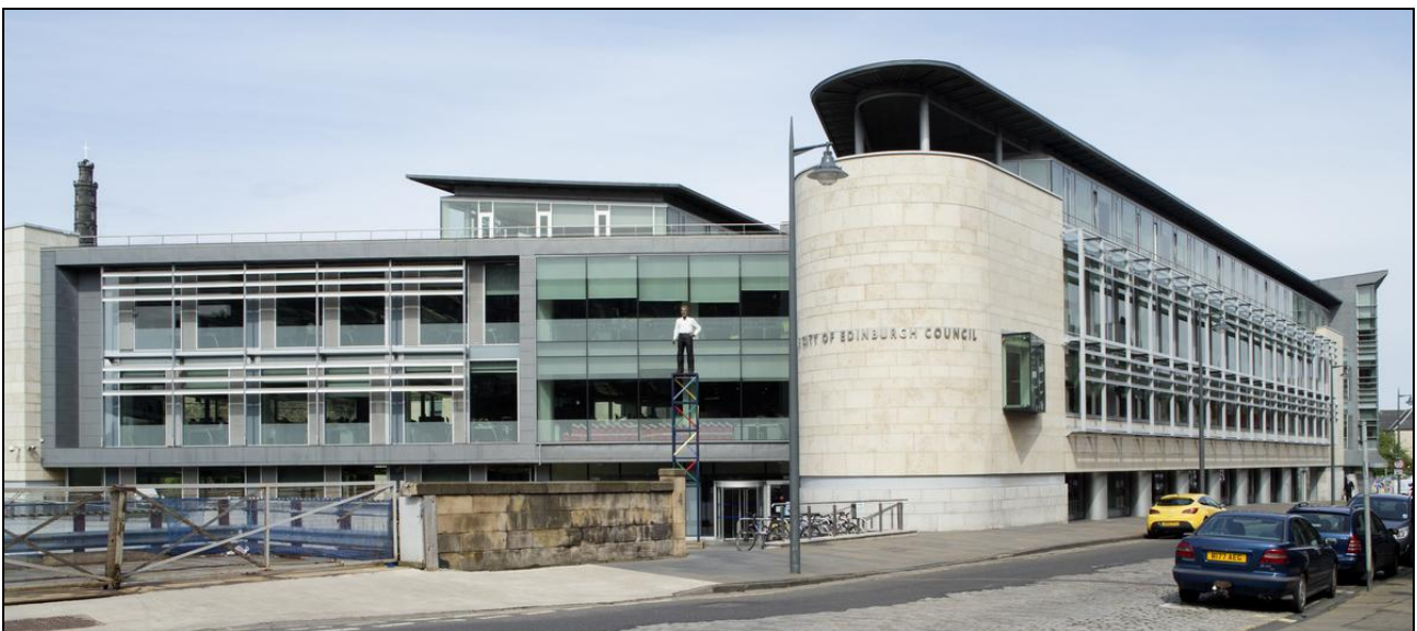
Figure 275: View of City of Edinburgh Council's HQ, Waverley Court, 4 East Market Street , from south-west, 2014 (DP190145 ©Crown copyright HES)
