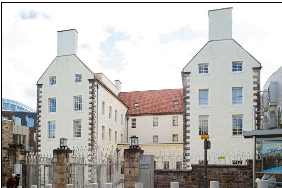
Figure 121: View of Queensberry House as part of the Scottish Parliament, 2013 (DP161330 ©Crown copyright HES)
