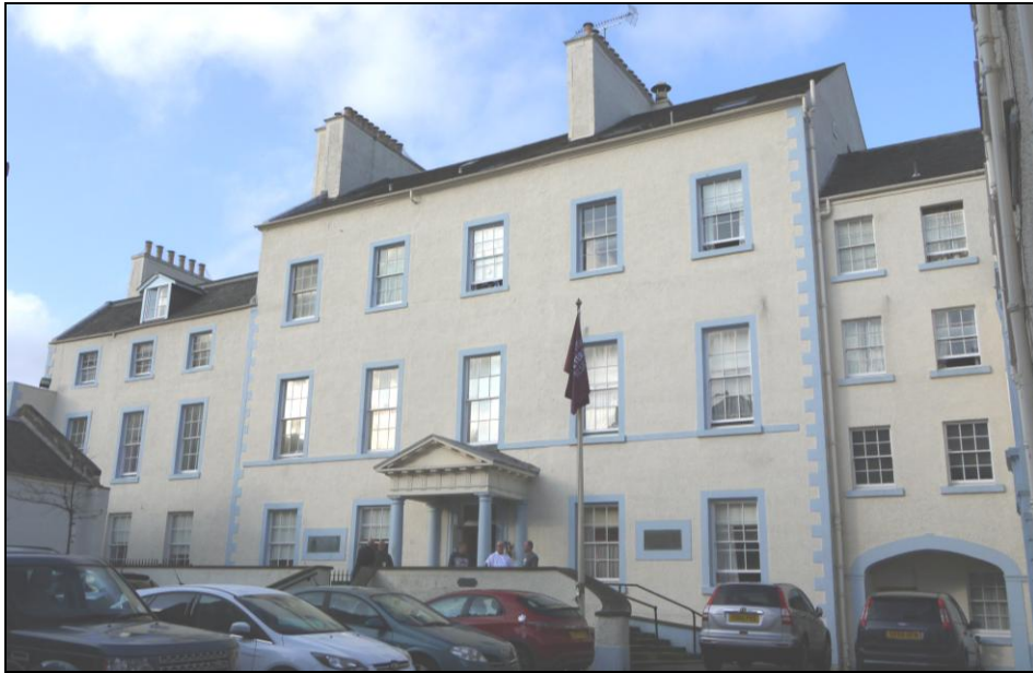
Figure 22: View of Whitefoord House and Callander House , from south, 2014 (DP207850 ©Crown copyright HES)
