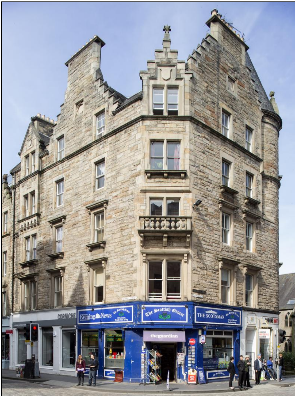
Figure 151: View of 2-18 Jeffrey Street , from south-west, 2014 (DP190127 ©Crown copyright HES)
