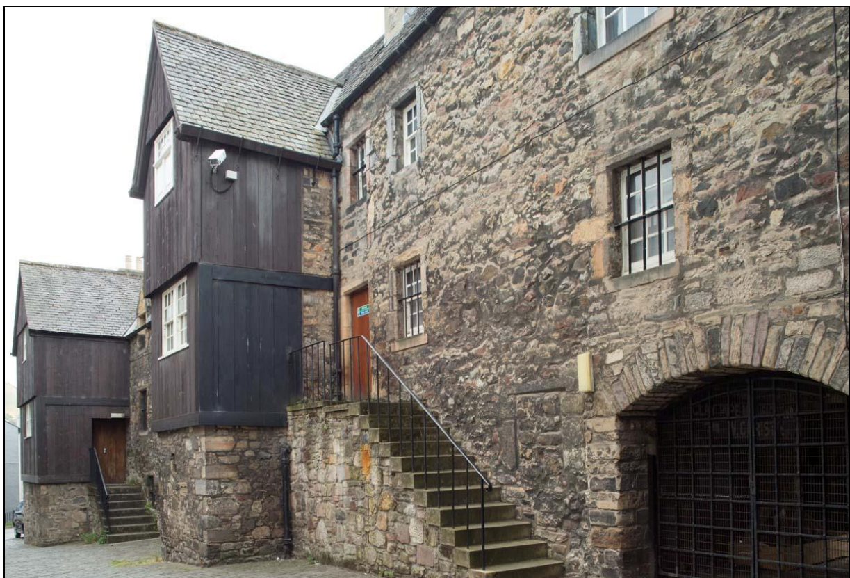
Figure 101: View of Bakehouse Close, from north, 2013 (DP158583 ©Crown copyright HES)
