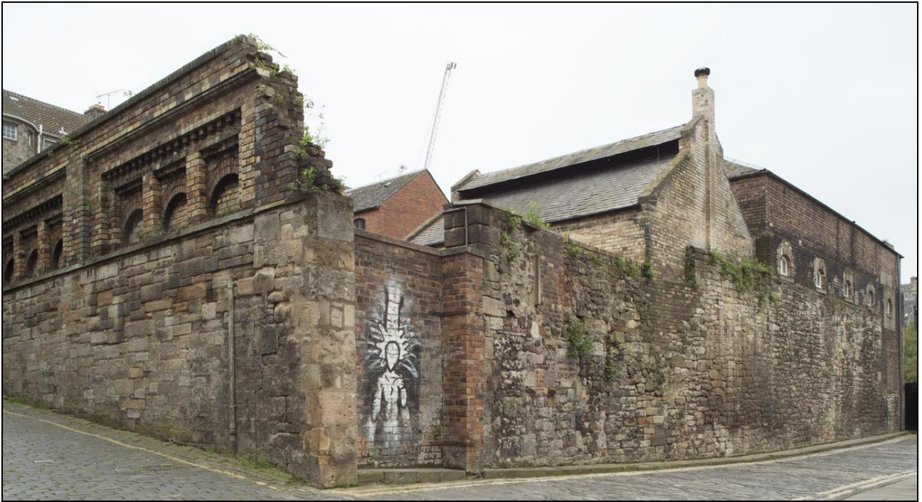
Figure 86: View of boundary wall and buildings of former Gasworks, Old Tolbooth Wynd, from north-east, 2014 (DP190184 ©Crown copyright HES)
