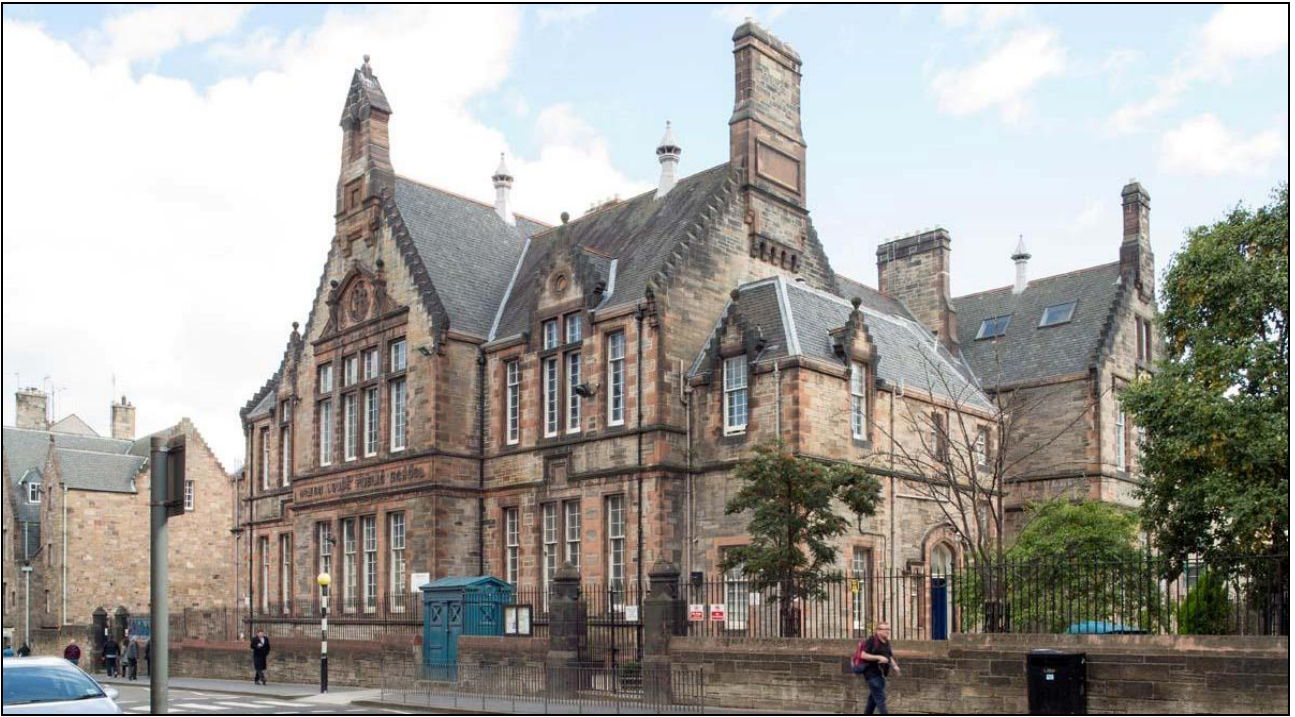
Figure 154: View of Royal Mile Primary School (Milton House Public School), from north-west, 2013 (DP161364 ©Crown copyright HES)
