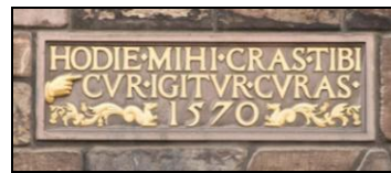
Figures 52, 53 and 54: Detail of plaques at Huntly House Museum, 142-6 Canongate, 2013 (DP158597 (top), DP158598 (centre) and DP158599 (bottom) ©Crown copyright HES)
