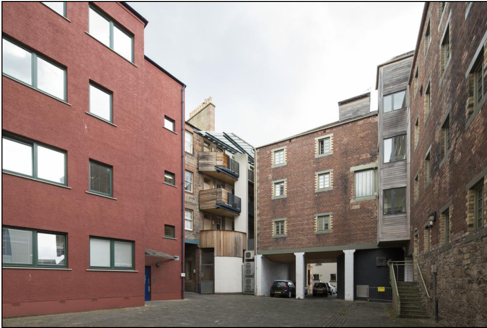
Figure 46: View of Cooper's Close, 114-120 Canongate , showing mixture of harling, stone, brick and timber cladding in backlands, 2014 (DP188649 ©Crown copyright HES)
