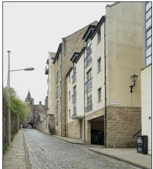
Figure 82: View of modern housing incorporating boundaries of Old Tolbooth Wynd, 2014 (DP190181 ©Crown copyright HES)
