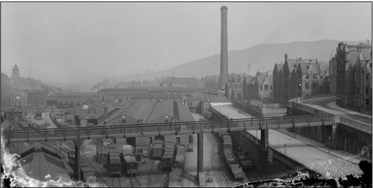
Figure 93: View of goods station at Waverley Station , from west, c.1900 (copied 2014) (SC1432916 ©Crown copyright HES)
