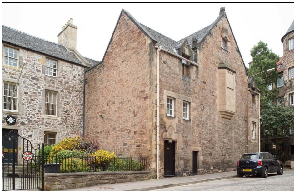
Figure 21: View of St John's Masonic Chapel , St John Street, from south-east, 2013 (DP158540 ©Crown copyright HES)
