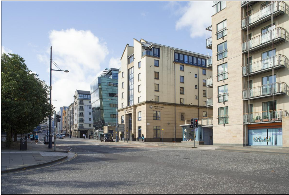
Figure 44: General view of developments along north side of Holyrood Road , looking west, 2014 (DP188504 ©Crown copyright HES)
