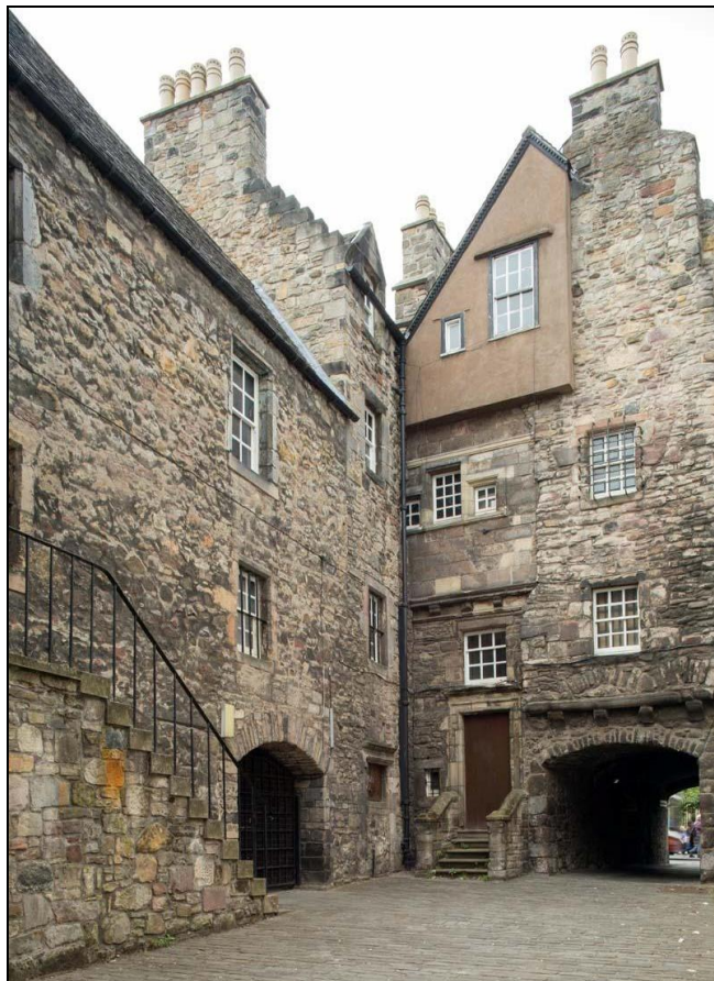
Figure 99: View of Bakehouse Close, from south, 2013 (DP158586 ©Crown copyright HES)
