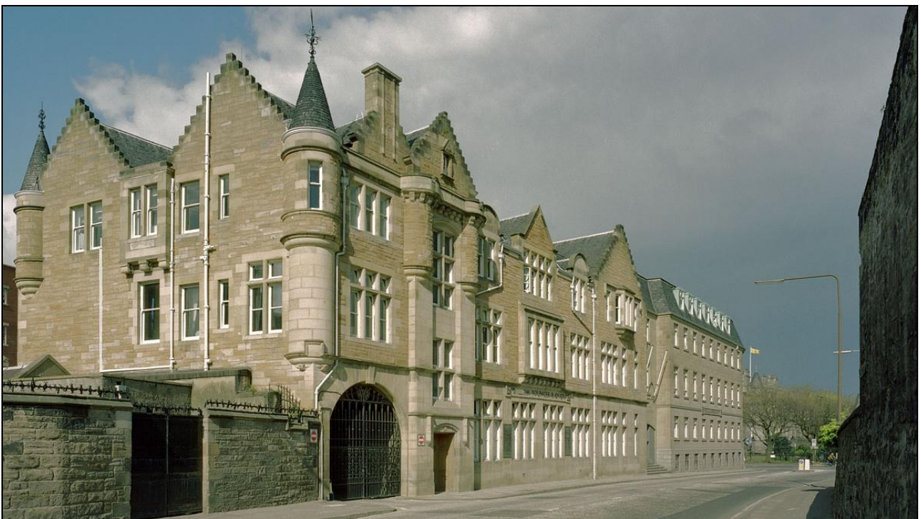
Figure 77: View of Holyrood Road elevation of Abbey Brewery , 1998 (copied 2003) (SC801757 ©Crown copyright HES)
