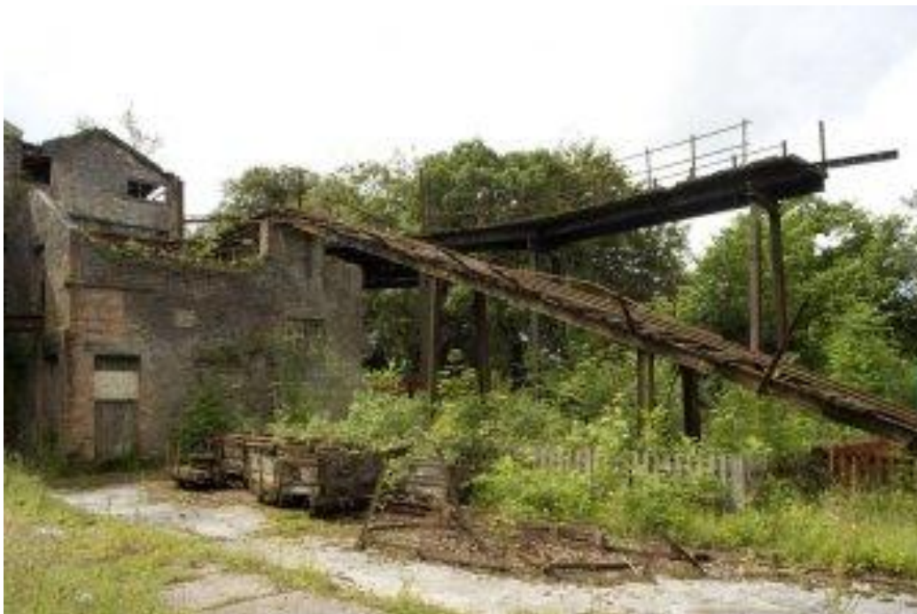
Birkhill Fireclay Mine, mine surface buildings. View of haulage gantry and 'run of mine' wagon rail gantry, from south. These structures have since been demolished. RCAHMS, 2007 [DP028368].
