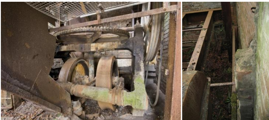
Above, left: Old Pan House with Incla Mill, from north. Chute on left from crusher on steel frame. The space was extremely cramped unlike the purpose-built New Pan House, RCAHMS, 2011 [DP11170]. Above centre: Old Pan House. The slapped through wall is clearly visible and the later steel structure carrying the crusher, which fed the Incla Mill, is to the left. Image: M McDonald, (2011).
