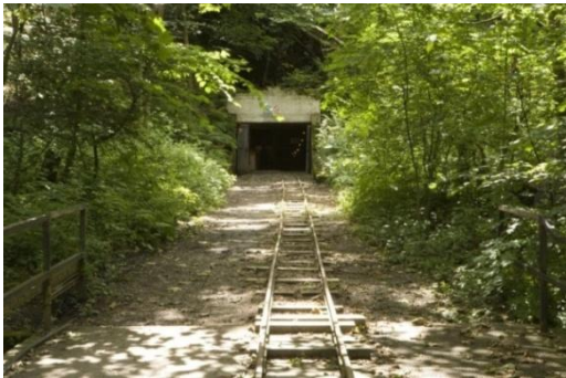
Above: View of reconstructed tramway as it enters Mine No 3, RCAHMS, 2007 [DP028338]
