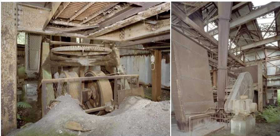
Far left: New Pan Mill House (post-1946), Pan Mill with the access mezzanine to the clay crusher above. RCAHMS, 2011 [SC1082490]. Left: View from south of New Pan Mill House. Bucket elevator and clay pit (left) return chute from screen sieve (centre) and drive motor (right). RCAHMS, 2011 [SC1082488]
