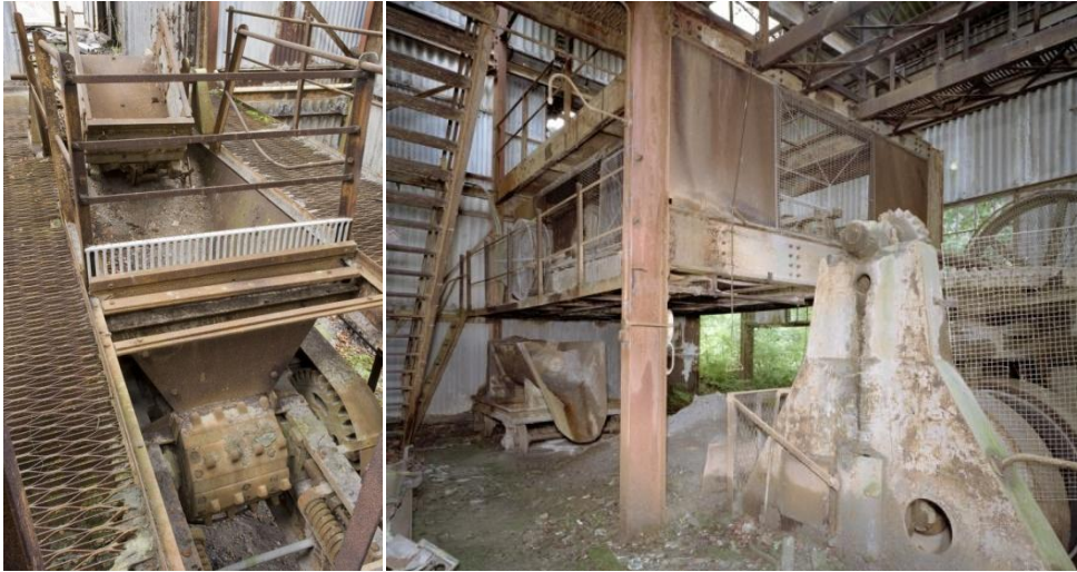
Above left: The tippler which tipped the clay wagon contents into the crusher below. RCAHMS, 2011 [SC1082489] Above right: View of the housing for the motors which drove the crusher and pan mill. The portable worm screw which pushed the crushed material from the crusher into the pan mill can be seen to the left. RCAHMS, 2011 [DP111671]
