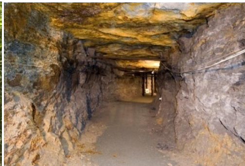
Above: Underground roadway or adit, RCAHMS, 2007 [DP028326]. Fireclay was mined using the 'stoop and room' or 'pillar and stall' method.
