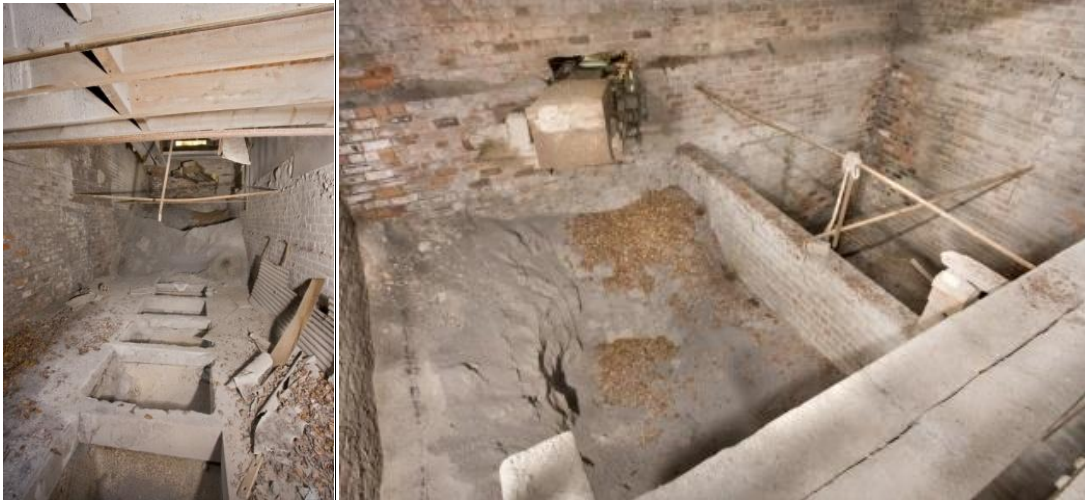
Above left: View of Hopper (SC1361816, D) above loading area from north, RCAHMS, 2011 [DP111695]. Above right: Hopper (SC1361816, D) above loading area, south end. The conveyor from the New Pan Mill House (post -1946) screens has been slapped through the south wall. RCAHMS, 2011 [DP111693]
