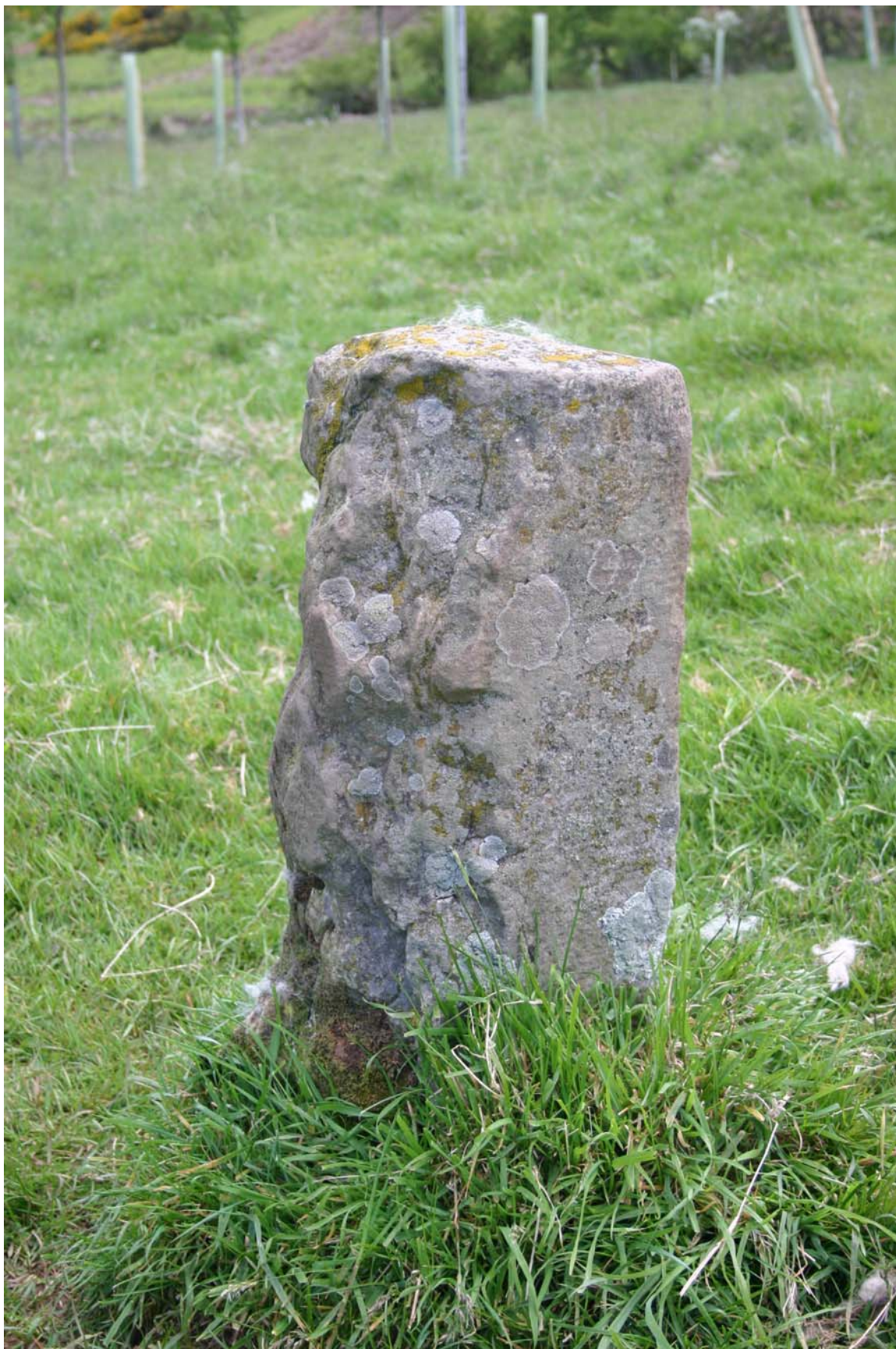
Illus 27. Dreghorn. View of one of the marker stones on the line of the Bonaly to Edinburgh water pipeline. Probably erected in the late 18 th or early 19 th century, this stone has been damaged by gunfire from the adjacent rifle-range (DP006704).
