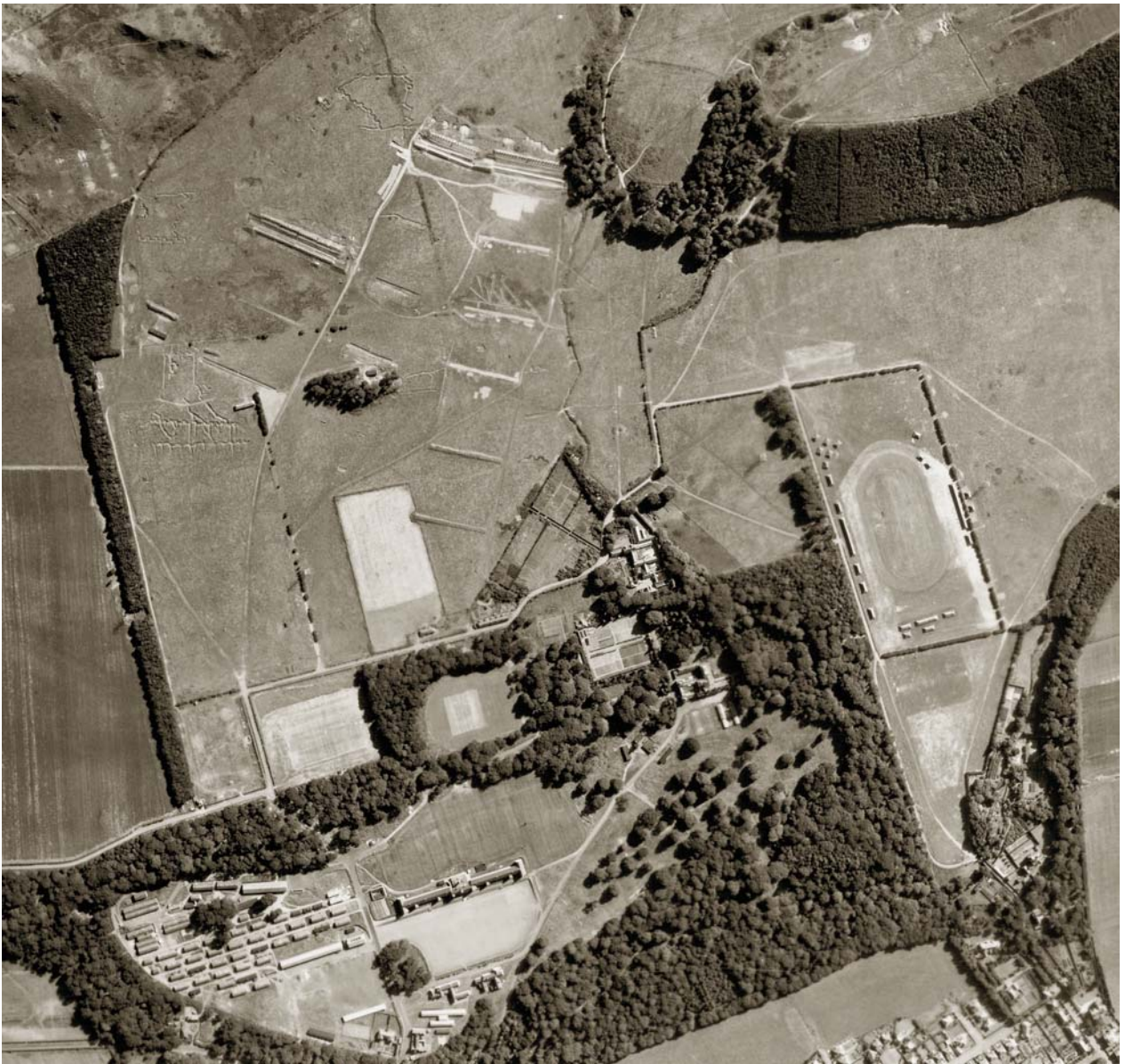
Illus 28. An RAF vertical aerial photograph (CPE/SCOT/UK 277, 5266), taken in 1947, centred on Dreghorn Castle, showing Dreghorn Mains farmsteading, the military small-arms ranges, practice-trench systems, sports facilities and barrack blocks (SC993232).
