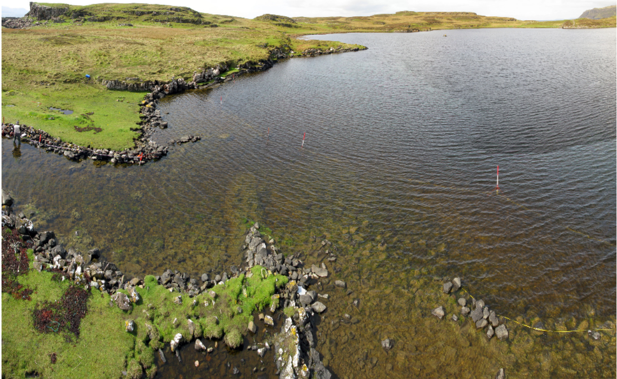
Figure 17. Canal entrance to loch (left); the line of the quay can be seen beyond marked by ranging rods. (Edward Martin)
