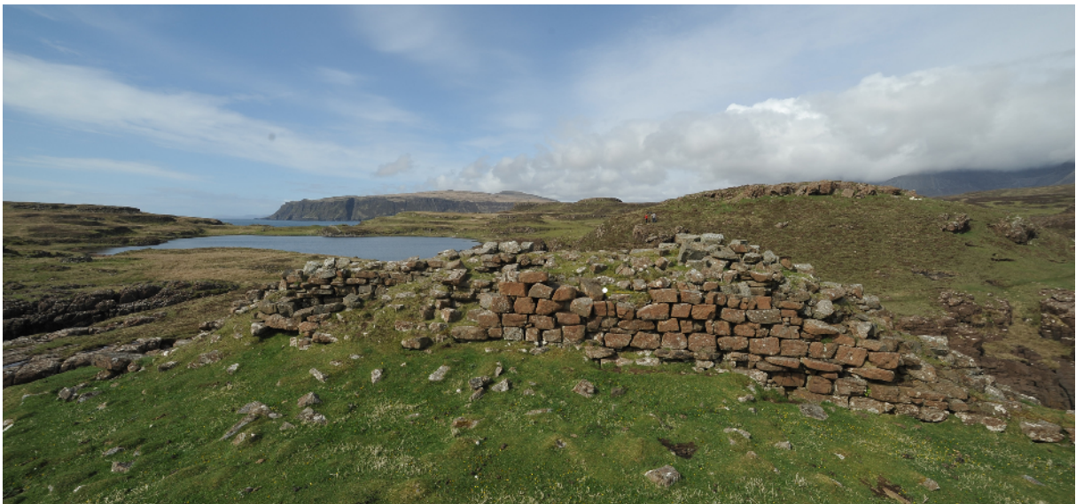
Figure 12. Dun wall from interior looking north-west. (Edward Martin)
