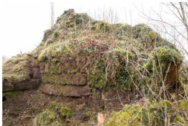
Fig 9 SE tower, showing the sloping plinth (see also Fig 22). DP151860
