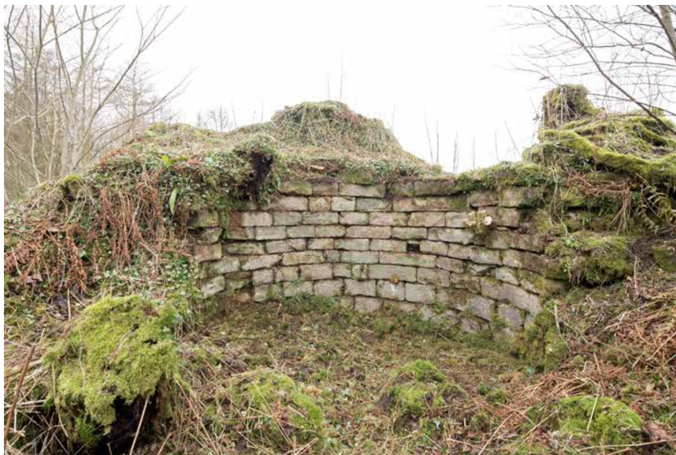
Fig 14 Basement of SSE tower. DP151827
