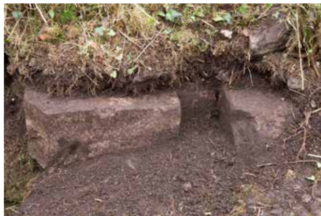
Fig 10 Portcullis slot on W side of entrance. DP151866
