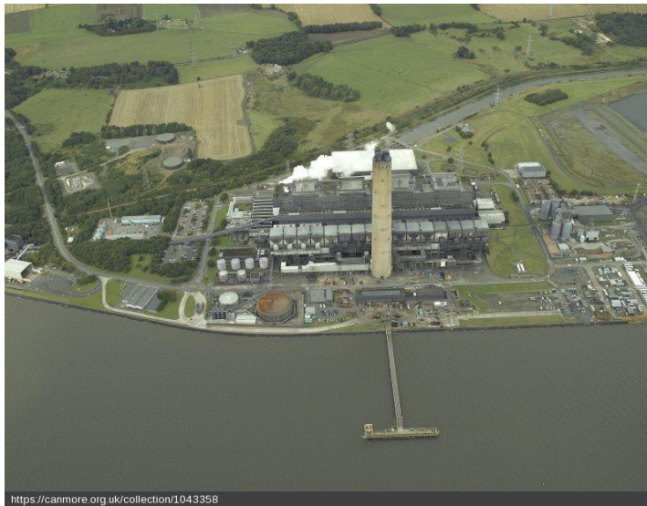
Longannet Electricity Generating Station from south [DP017135, 2006. Crown copyright: HES]
