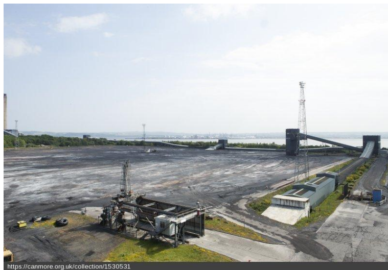
General view of coal yard from northwest. The power station is visible on the left. The conveyor on the right received coal from the vehicle coal discharge and the NCB buffer hopper that received its coal from the NCB Longannet Mine network discharge hopper [DP 237614, 2016. Crown copyright: HES]
