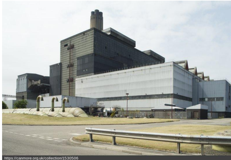
General view taken from the north west. From left to right, electrostatic precipitators, coal handling, boiler house and turbine house. [DP 237589, 2016. Crown copyright: HES]
