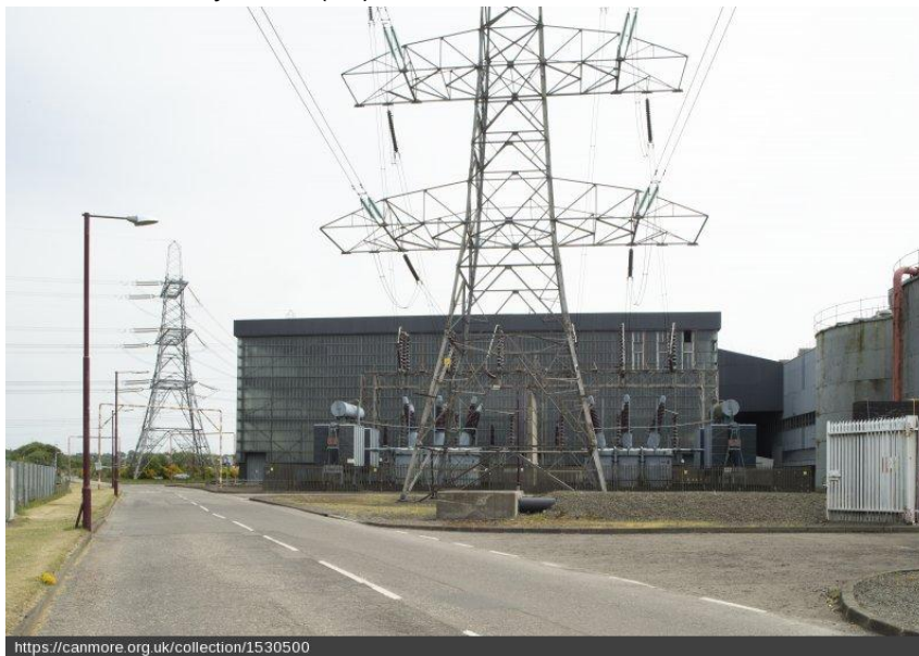
https://canmore.org.uk/collection/1530500 Switchhouse from north west [DP 237583, 2016. Crown copyright: HES]
