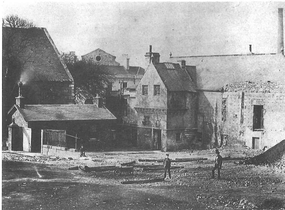
figure 32 Aberdeen Trades Hall, on the site of the Trinitarian Friary, may have incorporated former friary buildings
