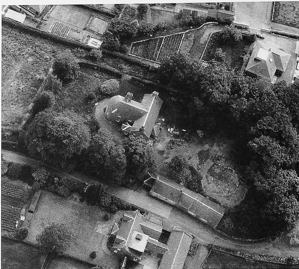
figure 5 Aerial view of Beech Hill House excavations 1989
