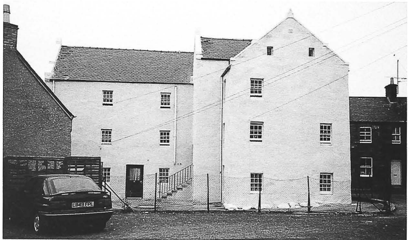
figure 11 Rear of Cumberland Barracks 1995
