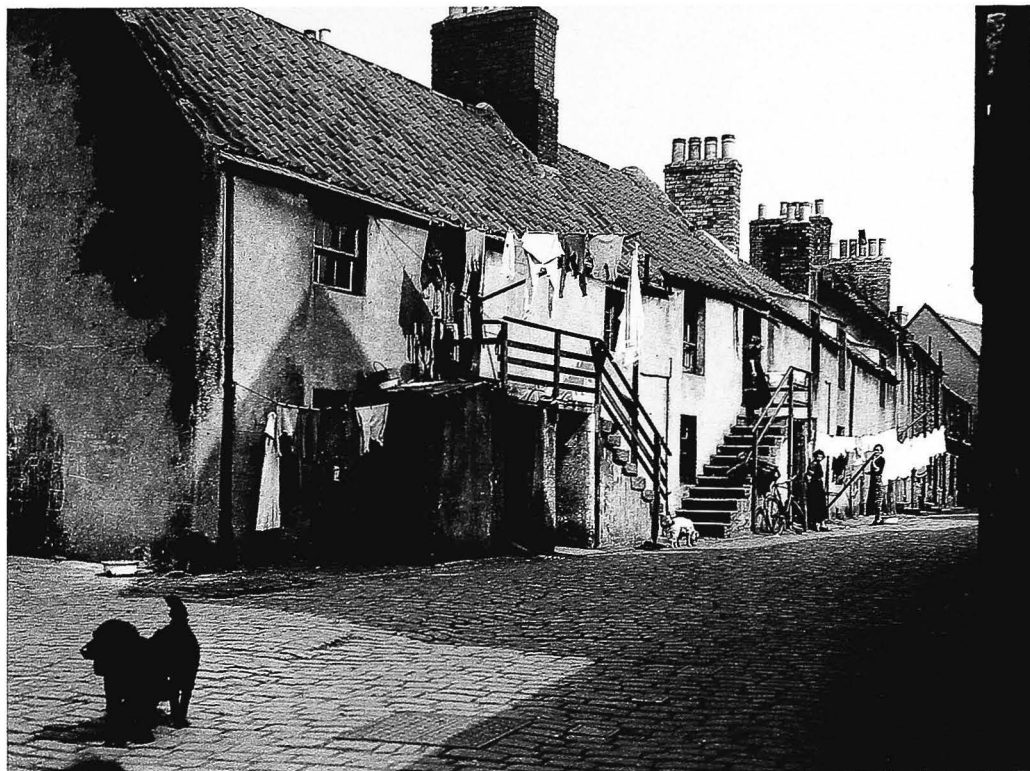
figure 17 North Wynd demolished c 1937
