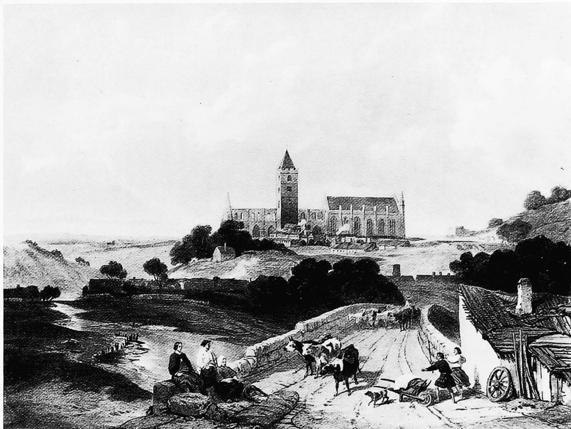
figure 8 Bridge over the Allan Water c 1855
