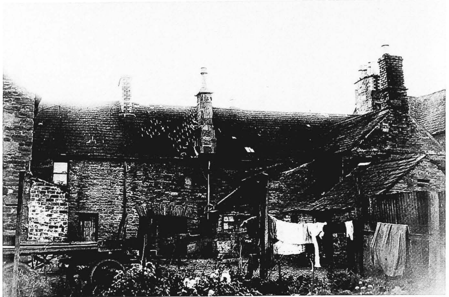
figure 23 Backlands of houses, East High Street
