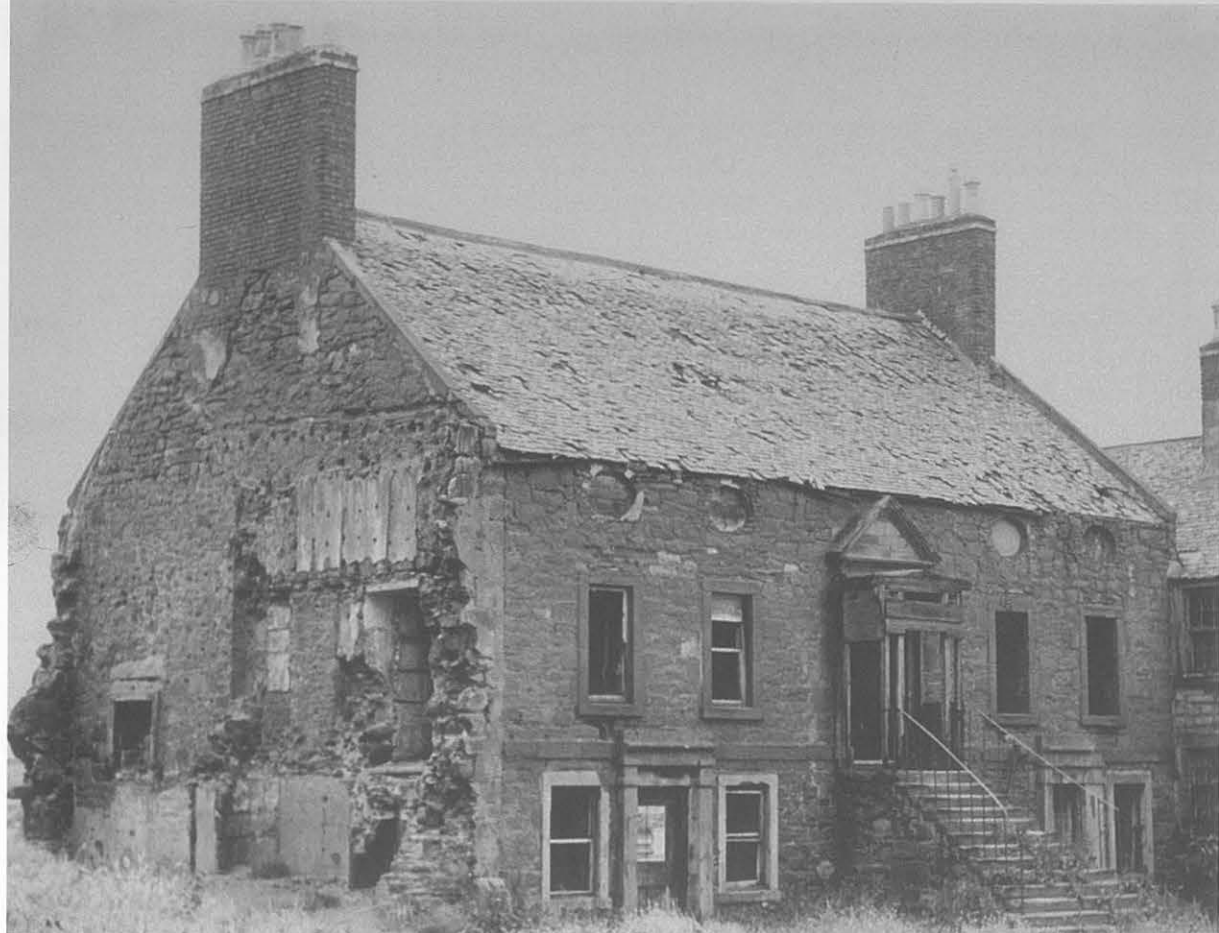
FIGURE 16 Dunbar Customs House, prior to demolition (By courtesy of Dr D Anderson and Dunbar and District History Society)
