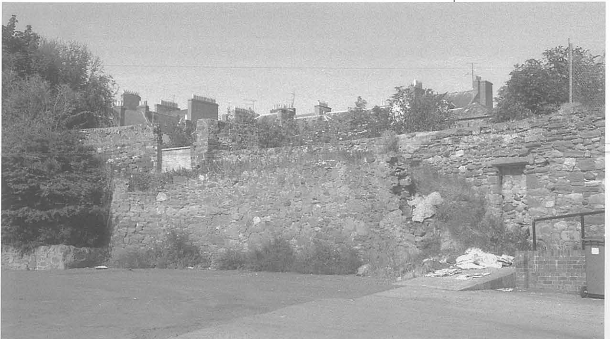
FIGURE 12 Friars' Walk and walls to the rear of burgage plots, 2002.
