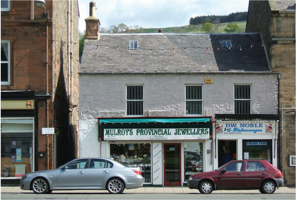
FIGURE 35 Early nineteenth-century houses in Bank Street (© Kirkdale Archaeology)
