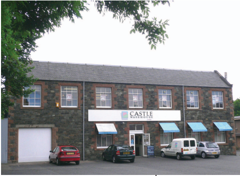
FIGURE 55 Langhaugh Mill, 2005 (© Crown Copyright Historic Scotland)
