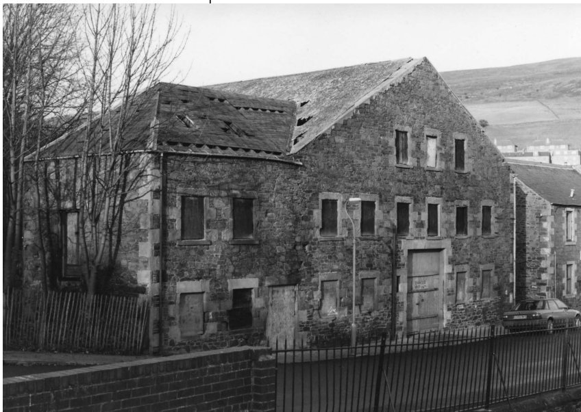
FIGURE 50 Deanbank Mill, 1990 (© Crown Copyright Historic Scotland)
