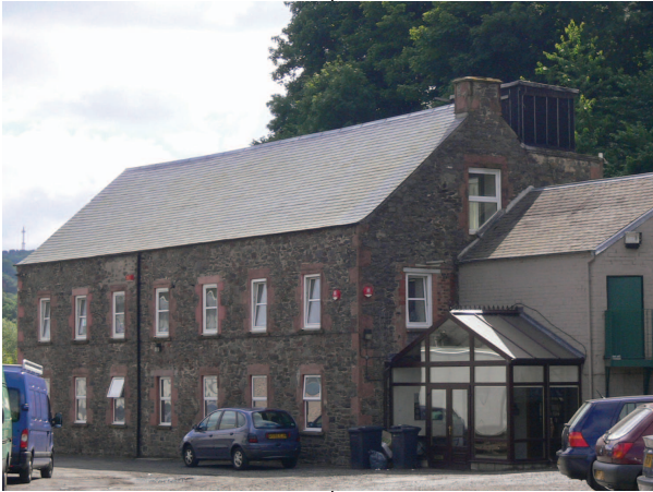
FIGURE 52 Galabank Mill, 2005 (© Crown Copyright Historic Scotland)
