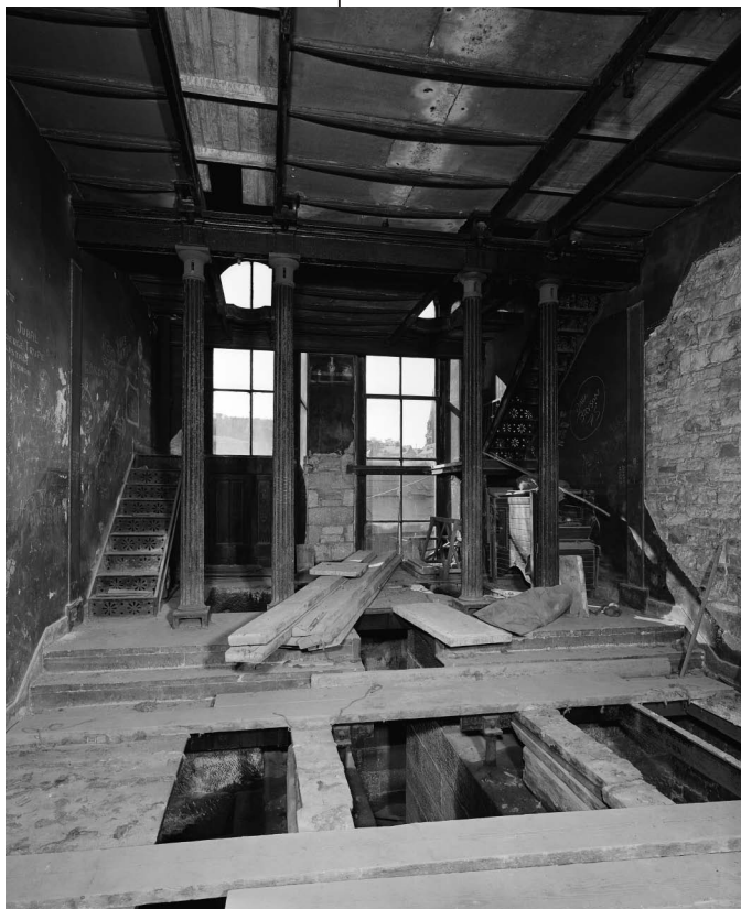
FIGURE 19 Mid or Valley Mill, interior of beam engine house, showing that this was a double engine, where two beams pivoted on an entablature carried by four columns. This arrangement is found only in the largest textile mills or in water pumping stations. Photographed before demolition in 1980 (By courtesy of RCAHMS; © Crown copyright RCAHMS)
