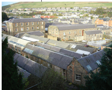
FIGURE 44 Botany Mill in 2005, showing the carding shed and four- storey weaving mill added in the 1870s (© Crown Copyright Historic Scotland)
