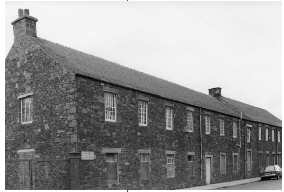
FIGURE 64 Waverley Mill/Waverley Ironworks, 1980 (© Crown Copyright Historic Scotland)
