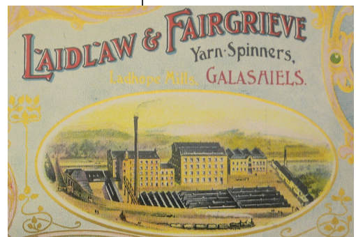
FIGURE 54 Ladhope Mill from Scotland's Industrial Souvenir II (1905) (Dundee Archive and Record Centre)
