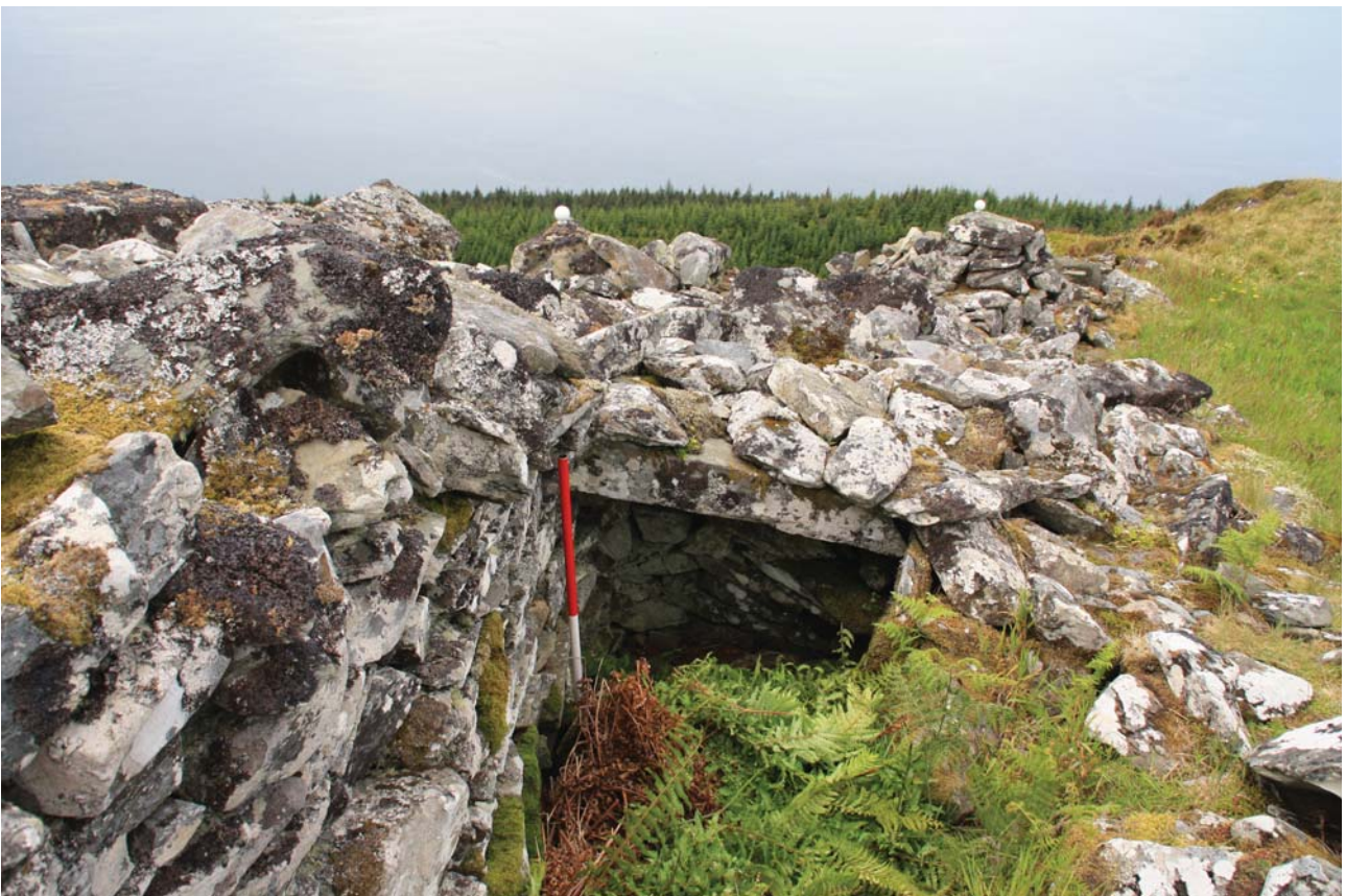
Plate 14: Partially intact corbelling at W end of cell, Point 5, from E
