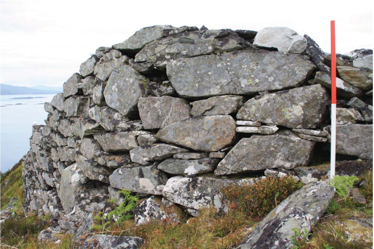
Plate 17: Outer wall face at Point 7, from S
