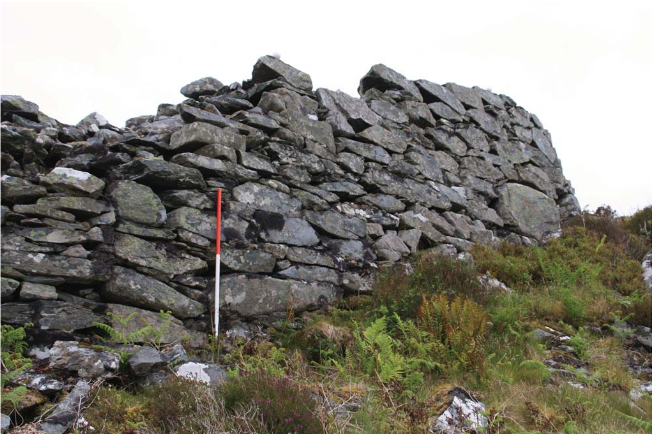
Plate 18: Outer wall face at Point 7, from S, showing straight joint
