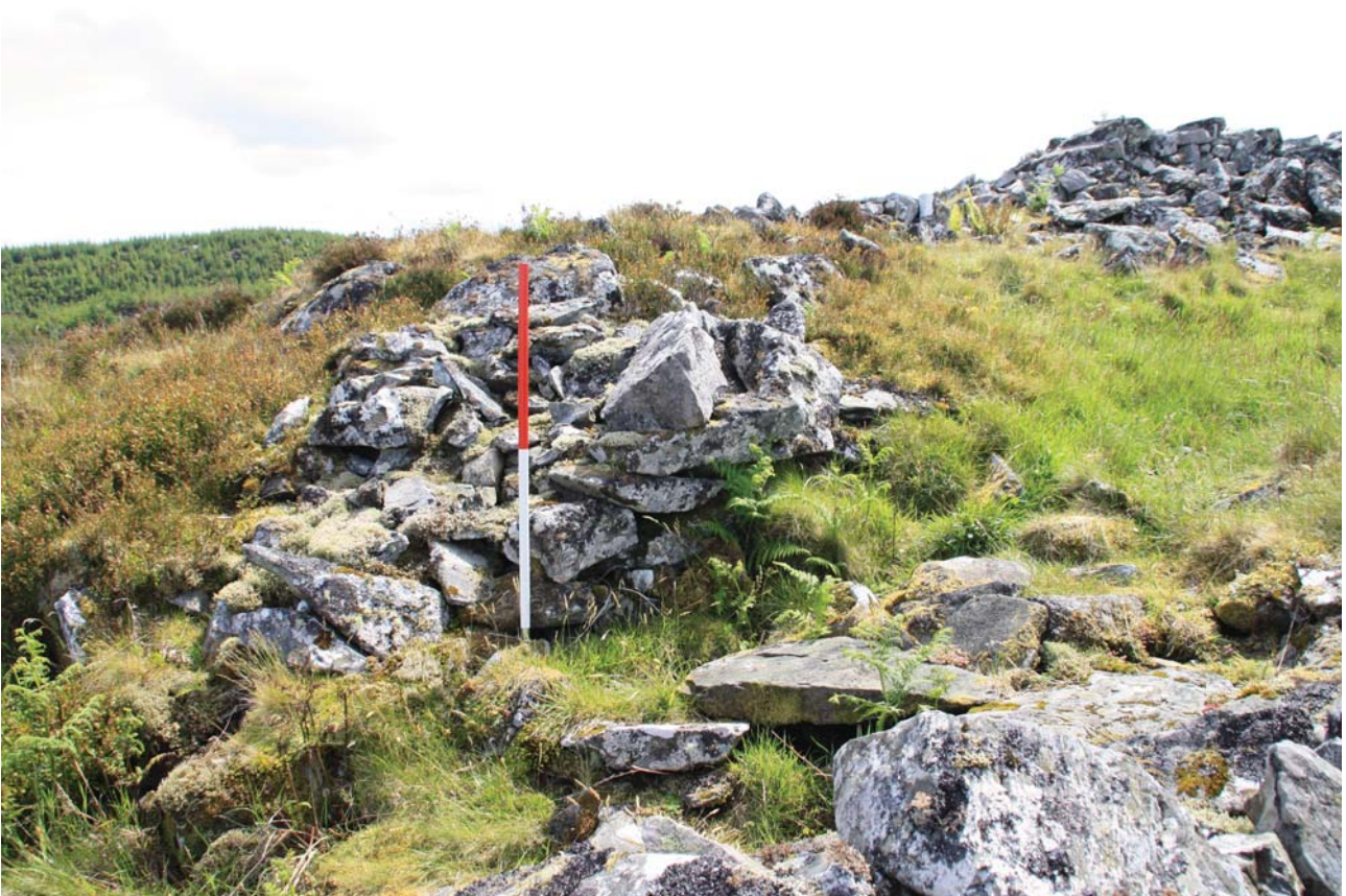
Plate 2: The E elevation of the entrance, from the NW
