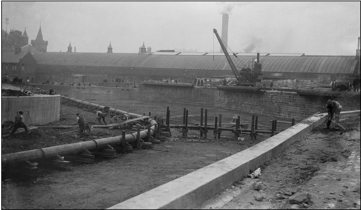
Figure 23: View of workmen blocking up and infilling Lochrin Basin , c.1906 (copied 2009) (Francis M Chrystal Collection, SC1130869 ©Crown copyright HES)
