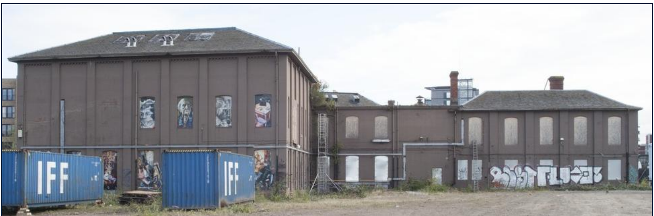
Figure 29: View of former North British Rubber Company, Fountainbridge/Gilmore Park, from south, 2014 (DP202947 ©Crown copyright HES)
