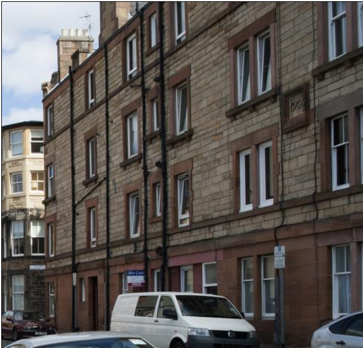
Figure 180: View of Nos 49-63 Watson Crescent, from west, showing red sandstone dressings and datestone '1906', 2014 (DP203088 ©Crown copyright HES)
