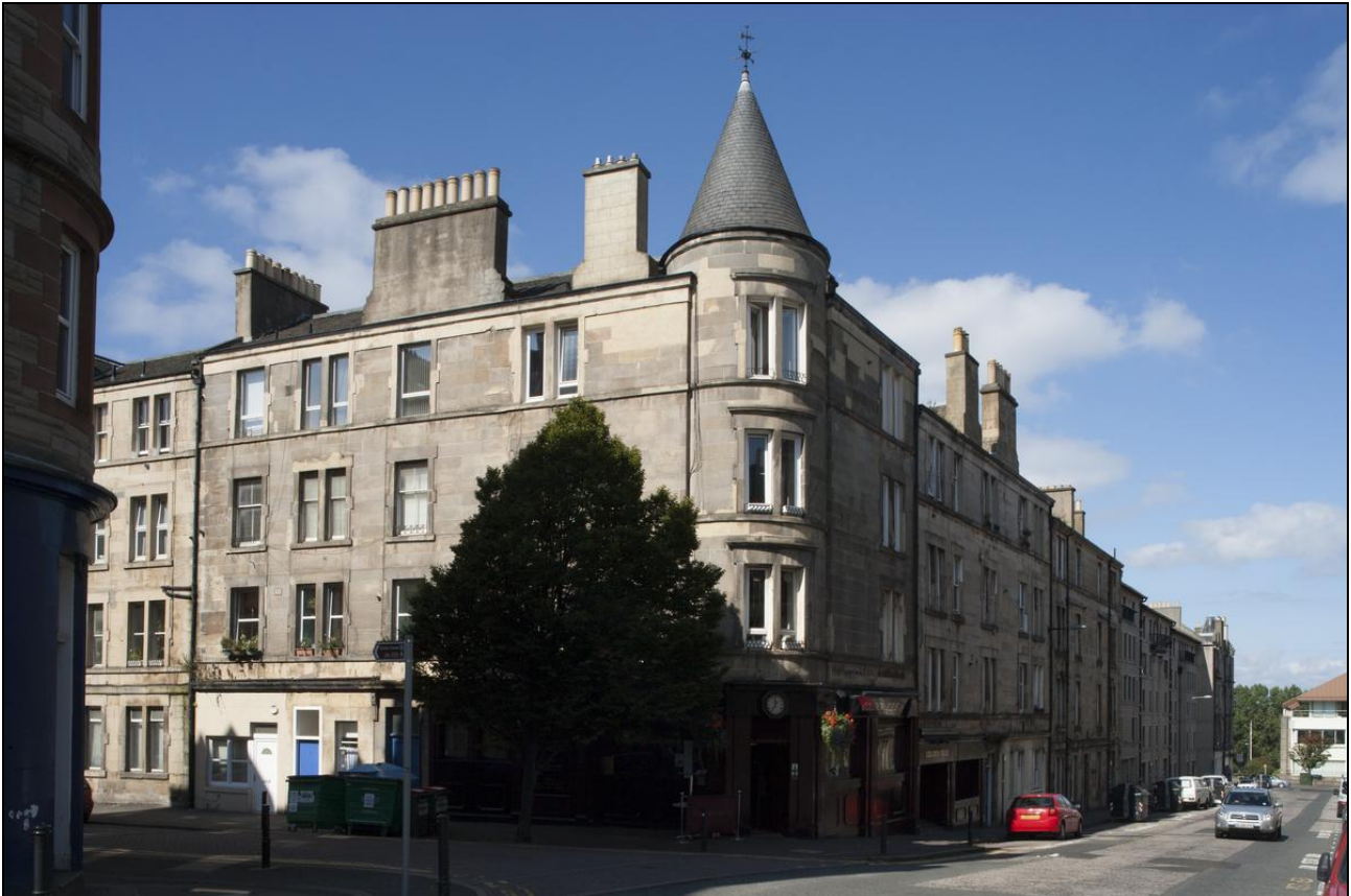
Figure 157: View of corner block at 2 Watson Crescent (left) and 30 Yeaman Place (right), from south-east, 2014 (DP199635 ©Crown copyright HES)
