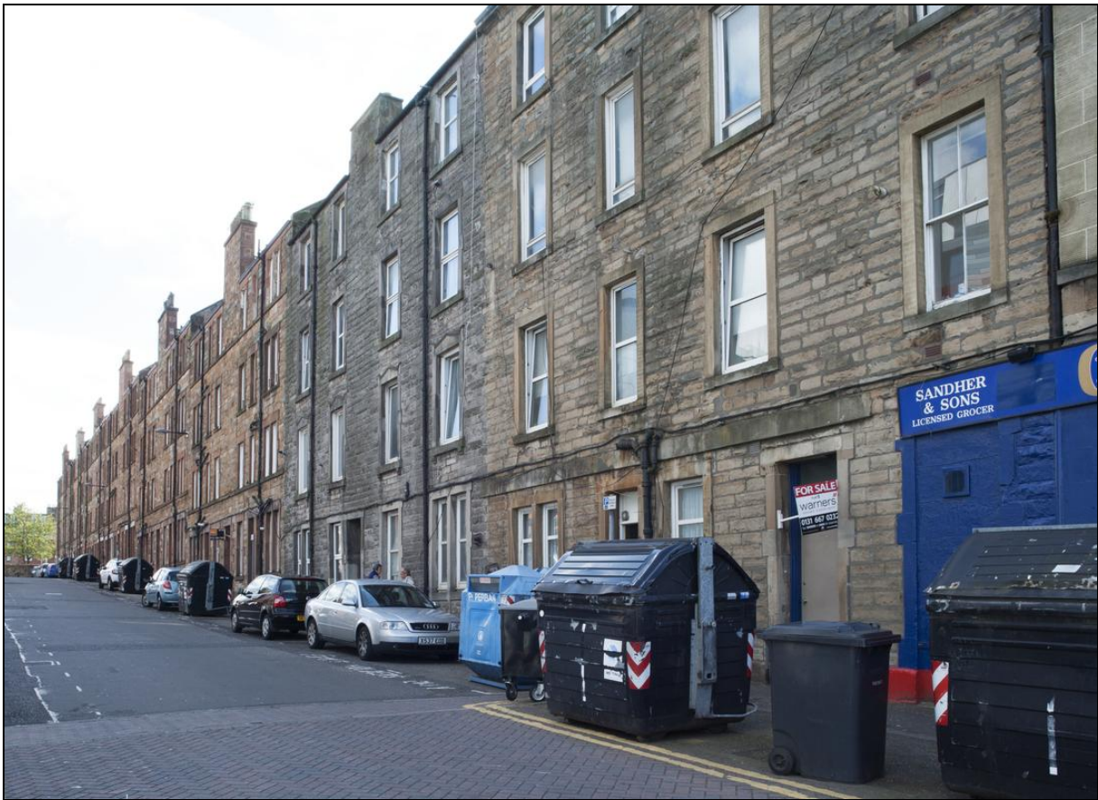
Figure 149: View of western side of Gibson Terrace , from north, showing 1870s tenements to the right, 2014 (DP203159 ©Crown copyright HES)
