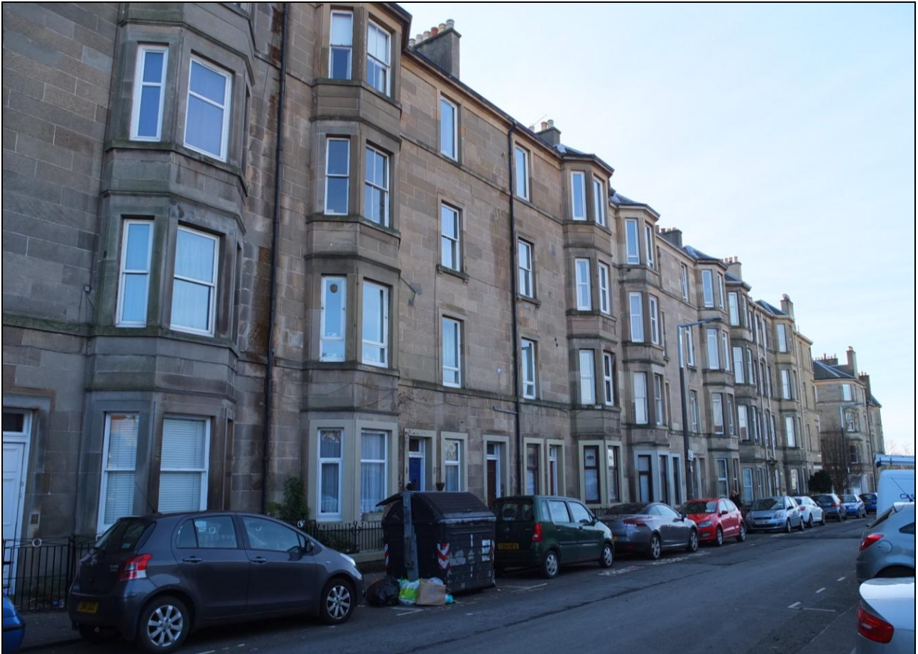
Figure 152: View of bay-windowed section of tenements on Dundee Terrace , from north-east, 2016 (DP232776 ©Copyright HES)
