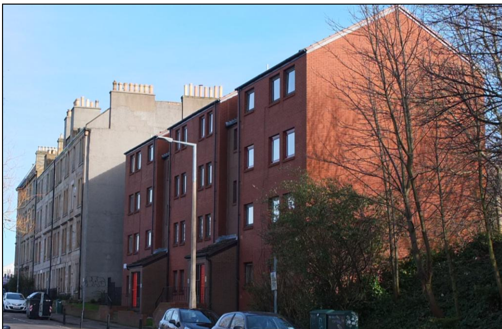
Figure 154: View of red brick development at west end of Dundee Terrace, from south-west, 2016 (DP232779 ©Copyright HES)
