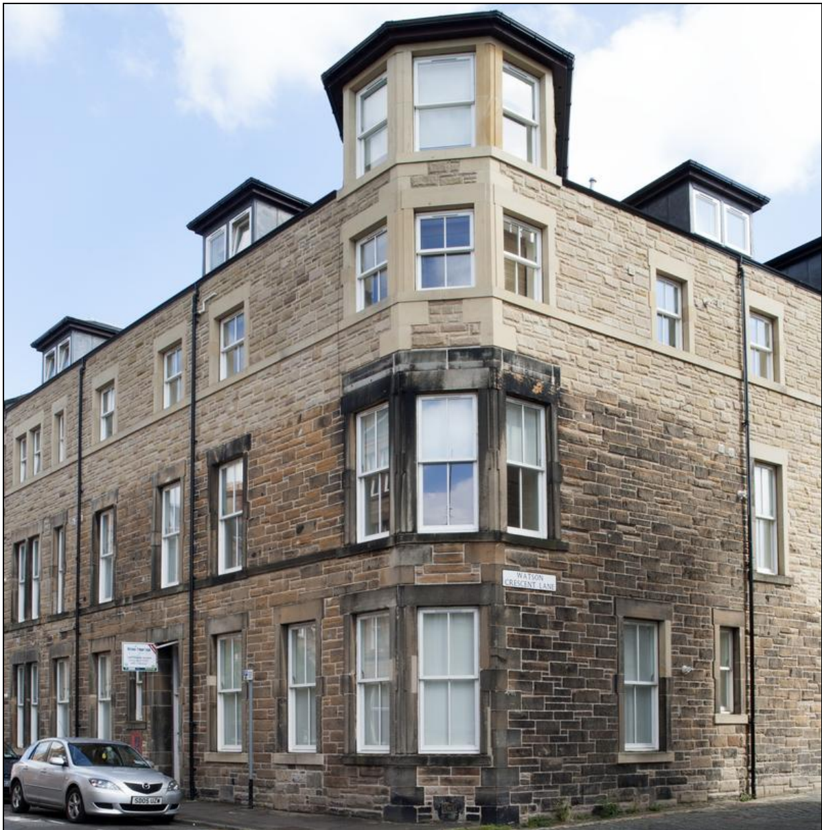
Figure 177: View of corner of 43 Watson Crescent/Watson Crescent Lane, from west, 2014 (DP203028 ©Crown copyright HES)
