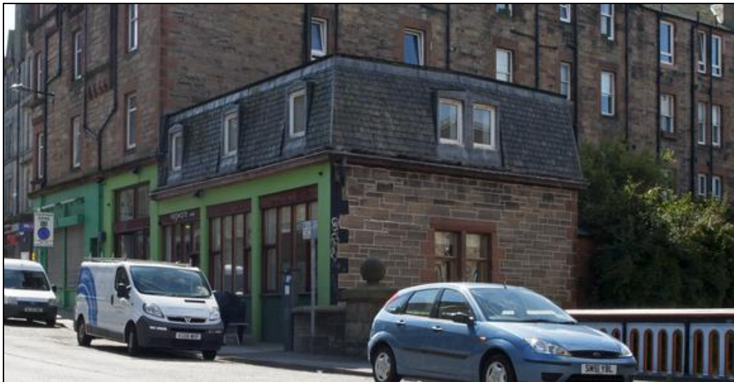
Figure 160: View of altered block at 43-45 Polwarth Crescent on south-western corner of Walker Bridge over Union Canal, from north-east, 2014 (DP202997 ©Crown copyright HES)
