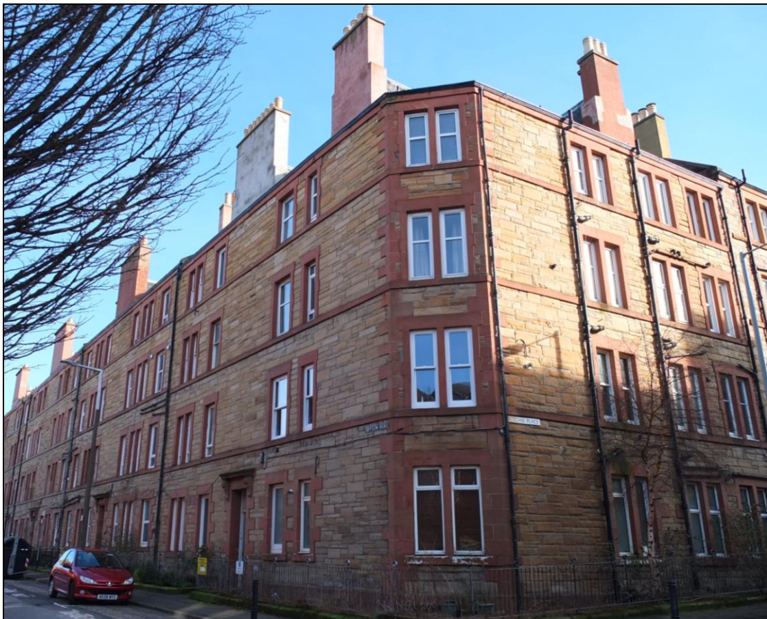
Figure 197: View of corner Bryson Road (left) and Ritchie Place (right), from west, 2016 (DP232769 ©Copyright HES)
