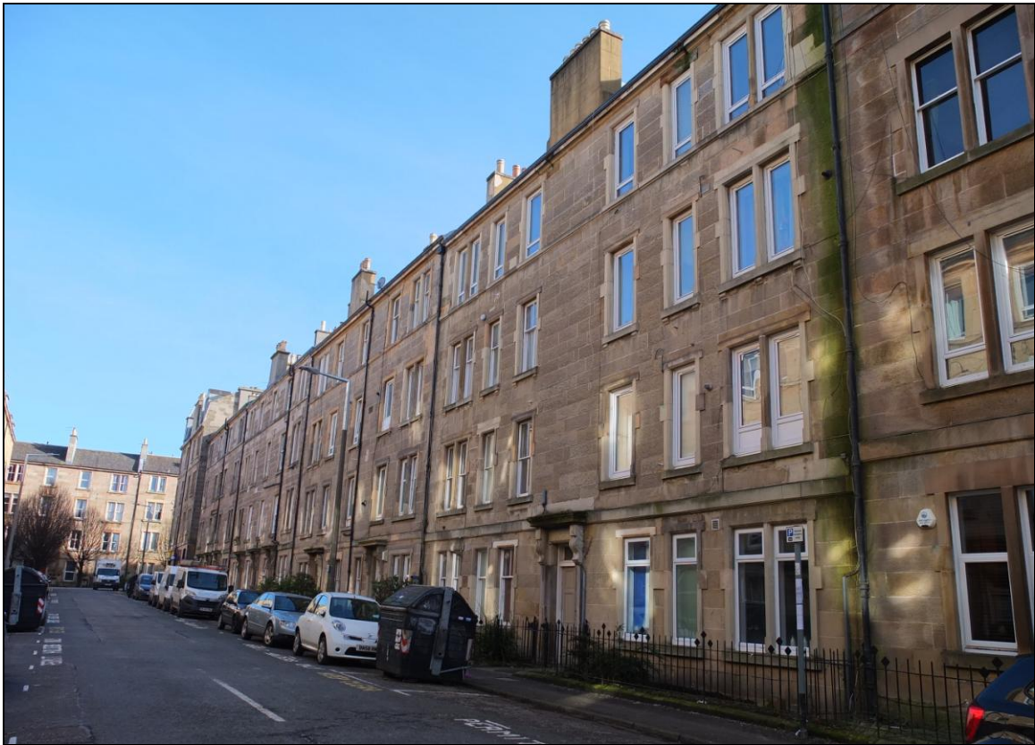
Figure 185: View of tenements on Bryson Road , from west, 2016 (DP232771 ©Copyright HES)
