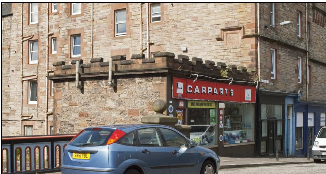
Figure 159: View of crenellated single-storeyed block at 36-38 Yeaman Place on north-western corner of Walker Bridge over Union Canal, from south-east, 2014 (DP202867 ©Crown copyright HES)
