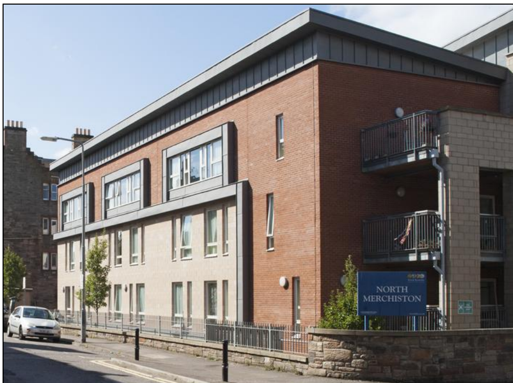
Figure 184: View of Watson Crescent elevation of North Merchiston Care Home, from east, 2014 (DP203093 ©Crown copyright HES)
