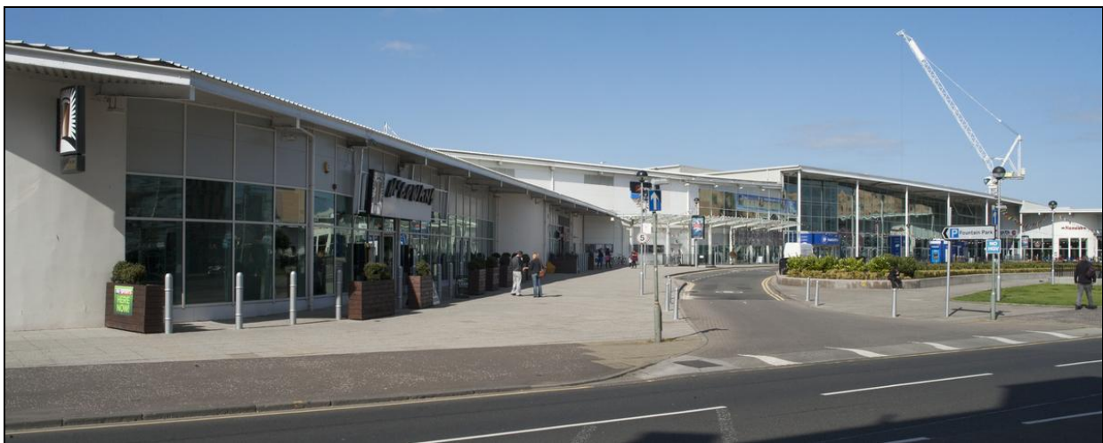
Figure 83: View of Fountain Park Leisure Complex, from south-west, 2014 (DP202973 ©Crown copyright HES)
