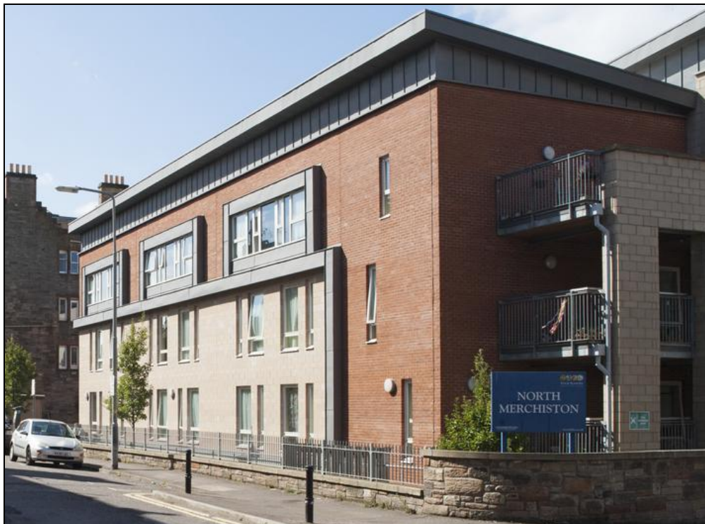
Figure 184: View of Watson Crescent elevation of North Merchiston Care Home, from east, 2014 (DP203093 ©Crown copyright HES)
