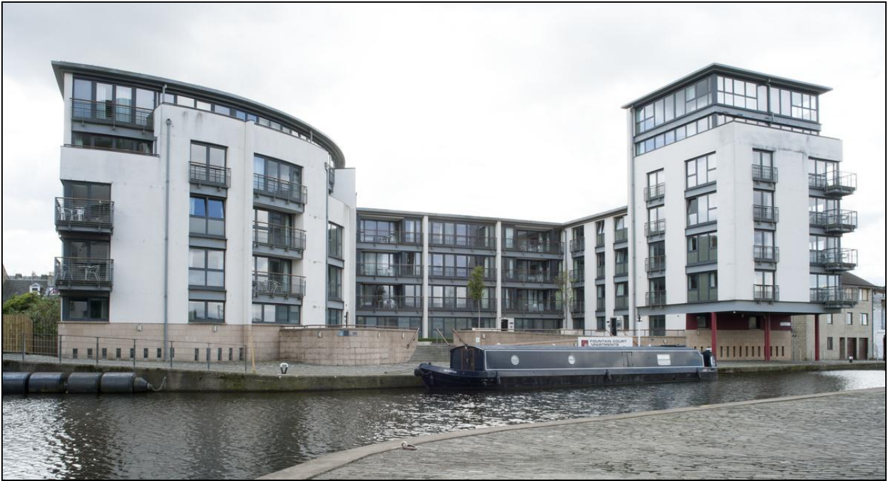
Figure 36: View of flats built at entrance to former Lochrin Basin, Lower Gilmore Place, from north-west, 2014 (DP195068 ©Crown copyright HES)
