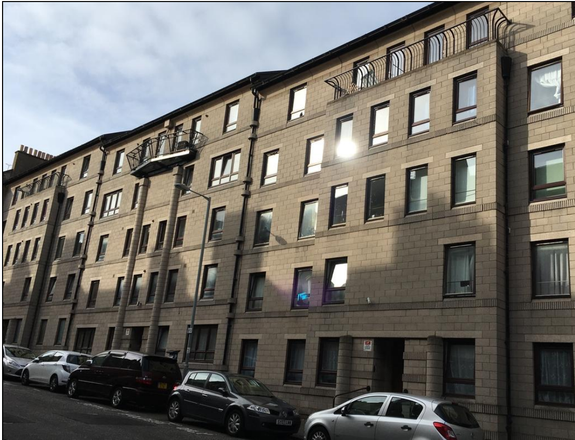
Figure 158: View of 10-16 Yeaman Place, from south-east, 2017 (DP260086 © HES)
