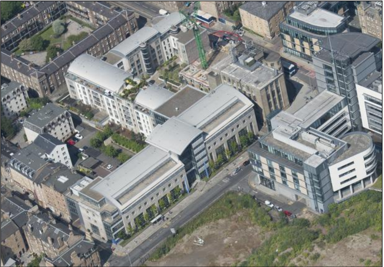
Figure 94: Aerial view showing Citymark offices and flats on Fountainbridge, 2014 (DP193076 ©Crown copyright HES)
