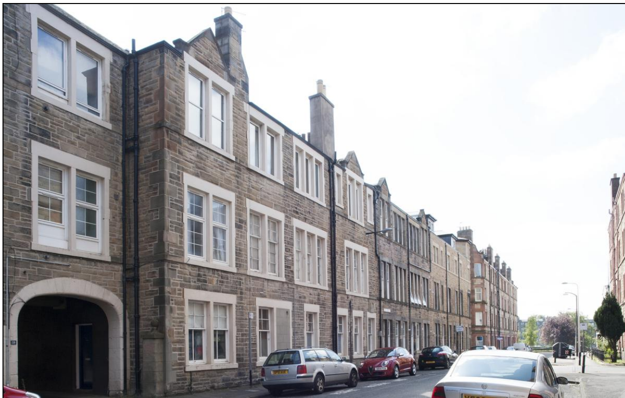
Figure 174: View of 39-43 Watson Crescent , from east, 2014 (DP203081 ©Crown copyright HES)
