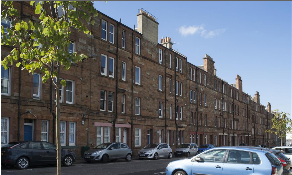
Figure 150: View of western side of Gibson Terrace, from south-east, showing 1890s tenements to the left, 2014 (DP203162 ©Crown copyright HES)
