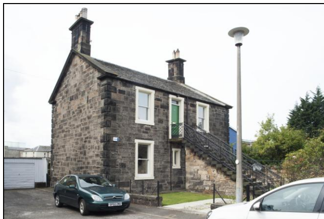
Figure 112: View of 35-6 Rosebank Cottages , from north-east, 2014 (DP203784 ©Crown copyright HES)
