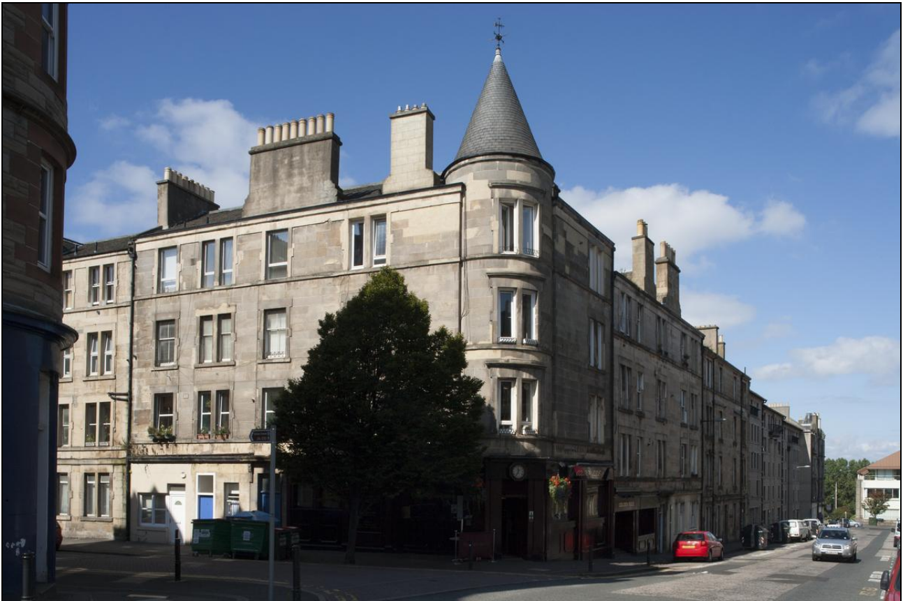
Figure 157: View of corner block at 2 Watson Crescent (left) and 30 Yeaman Place (right), from south-east, 2014 (DP199635 ©Crown copyright HES)
