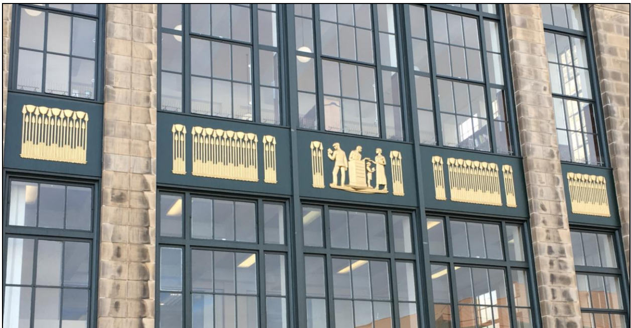
Figure 148: Detail of painted bronze-plated cast-iron panels on Dundee Street elevation of Fountainbridge Public Library, 2017 (DP260083 ©Crown copyright HES)
