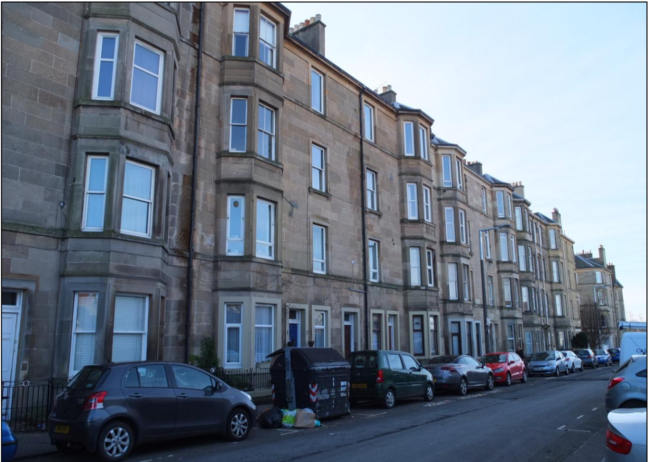
Figure 152: View of bay-windowed section of tenements on Dundee Terrace , from north-east, 2016 (DP232776 ©Copyright HES)
