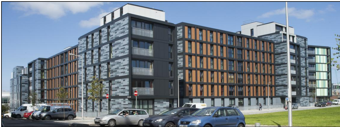
Figure 65: View of Napier University's student residences on eastern side of Gibson Terrace , from south-west, 2014 (DP203164 ©Crown copyright HES)
