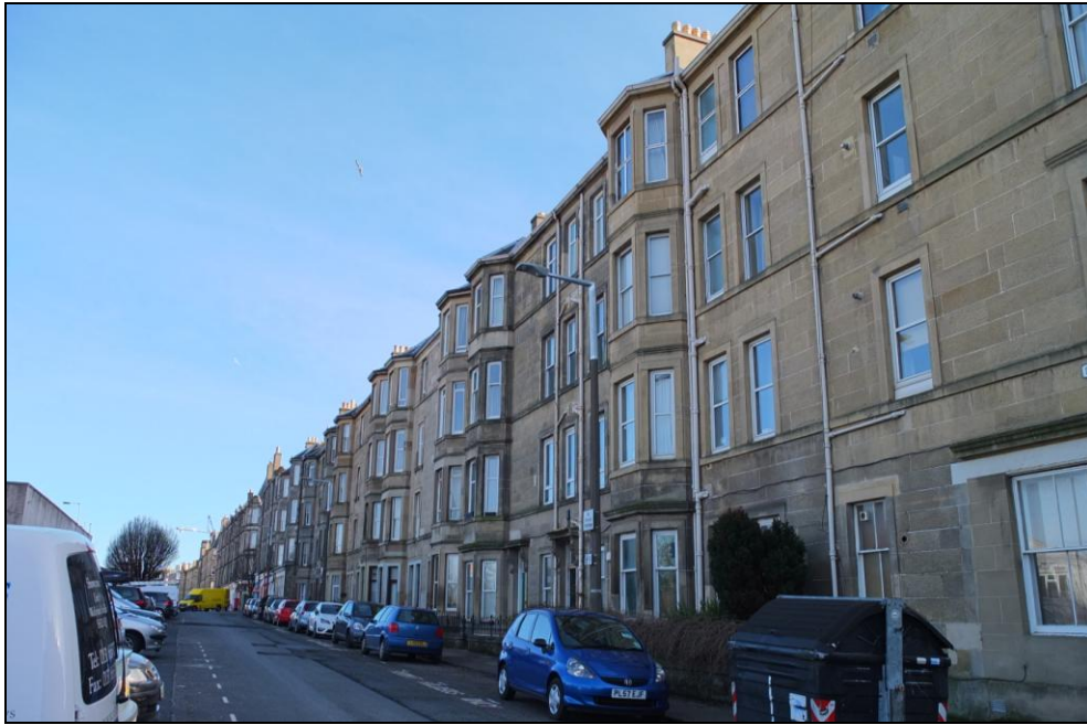
Figure 153: View of some of plain-fronted tenements on Dundee Terrace, from west, 2016 (DP232777 ©Copyright HES)
