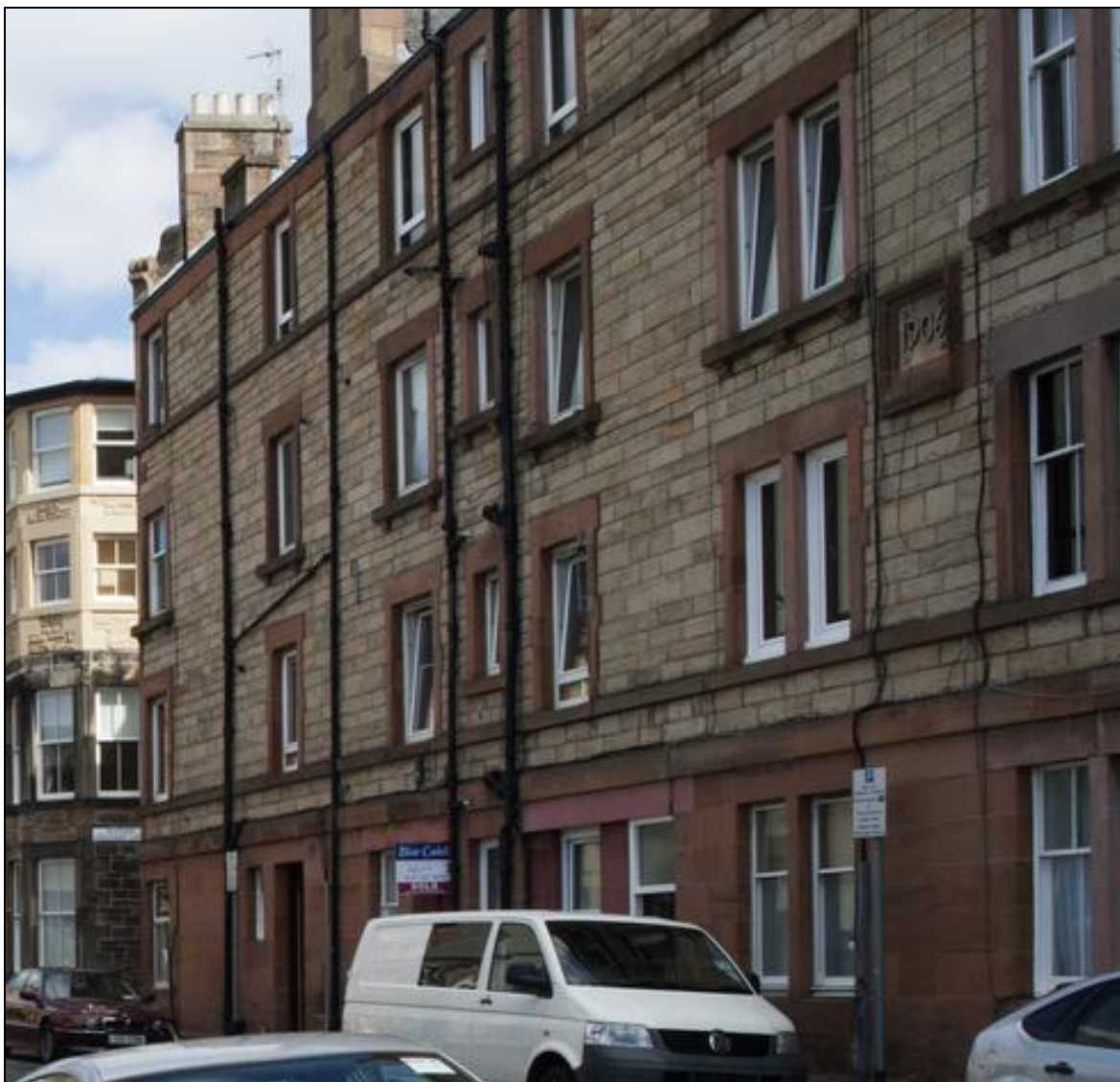
Figure 180: View of Nos 49-63 Watson Crescent, from west, showing red sandstone dressings and datestone '1906', 2014 (DP203088 ©Crown copyright HES)
