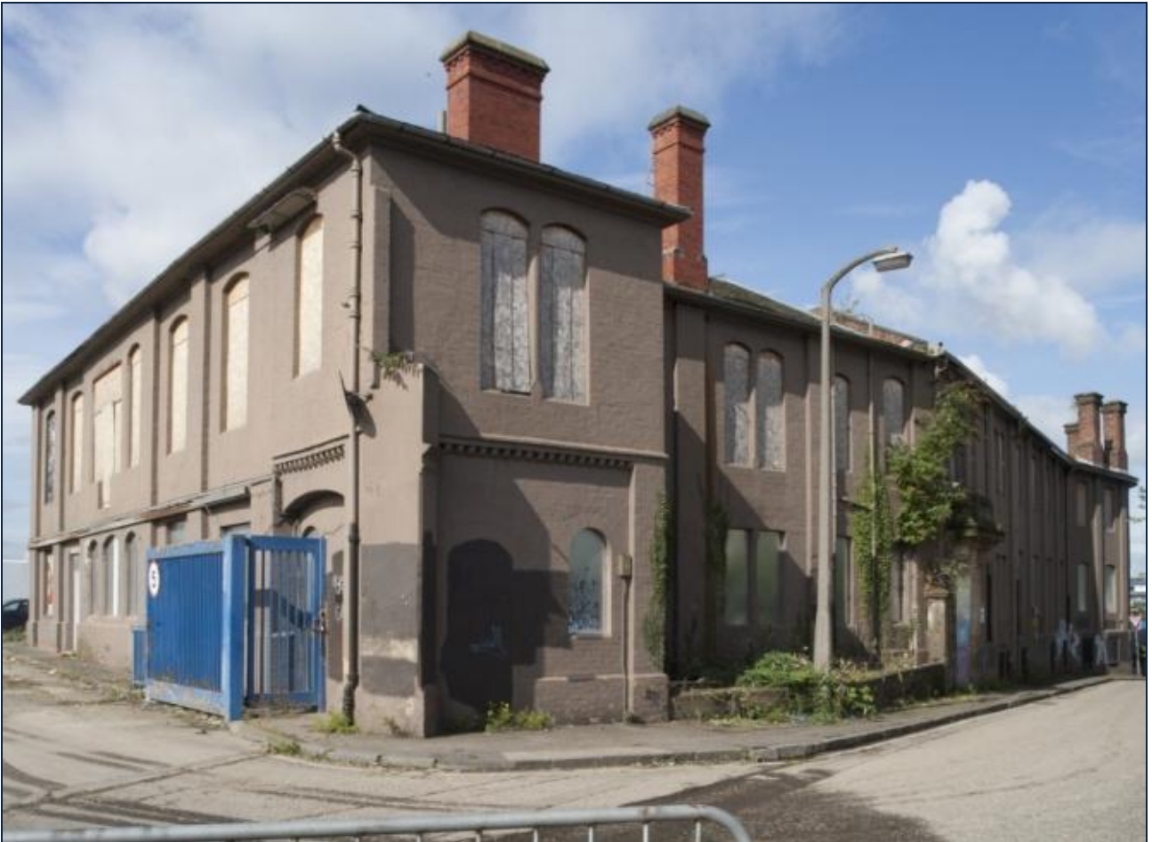
Figures 28: View of former North British Rubber Company , Fountainbridge/Gilmore Park, from south-east, 2014 (DP202952 ©Crown copyright HES)
