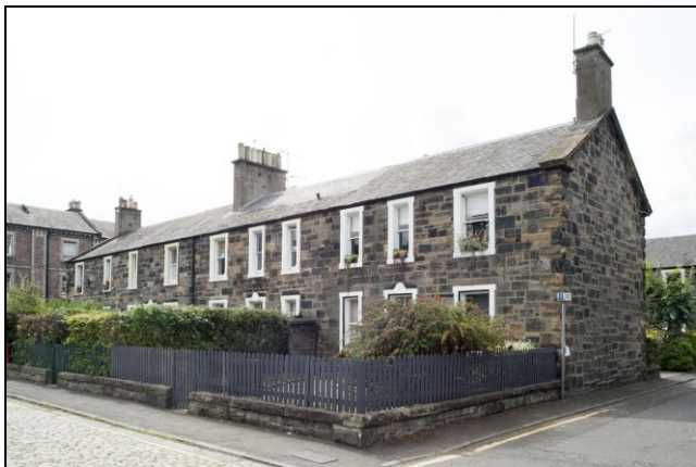
Figure 109: View of 1-8 Rosebank Cottages , from north-east, 2014 (DP203792 ©Crown copyright HES)
