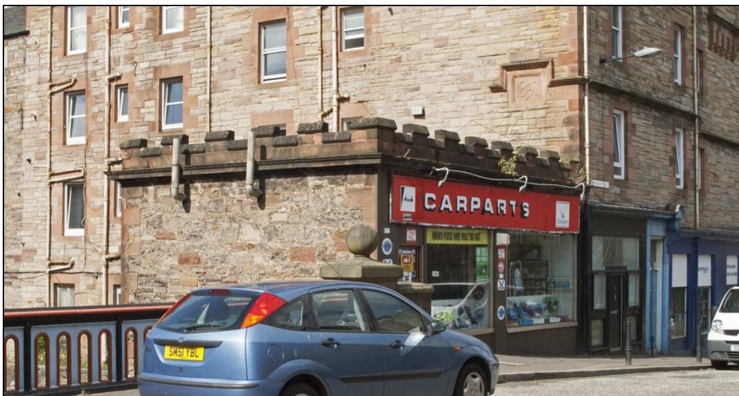
Figure 159: View of crenellated single-storeyed block at 36-38 Yeaman Place on north-western corner of Walker Bridge over Union Canal, from south-east, 2014 (DP202867 ©Crown copyright HES)
