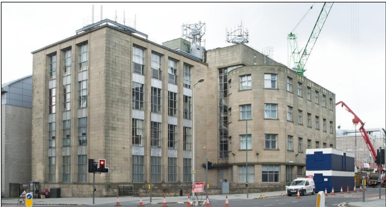
Figure 101: View of Telephone Exchange, 116 Fountainbridge , from south-east, 2014 (DP203620 ©Crown copyright HES)
