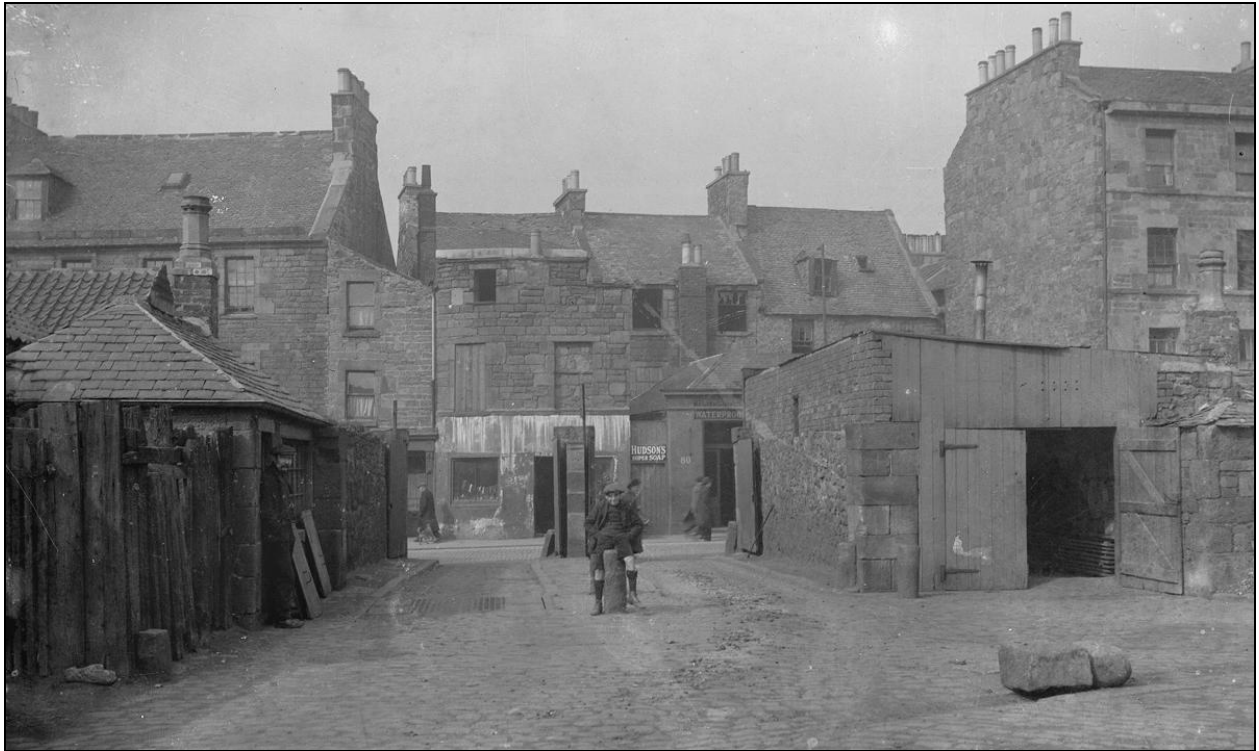
Figure 80: View of entrance to Port Hamilton with Simple Street in background, c.1900 (copied 2009) (SC410027 ©Crown copyright HES)
