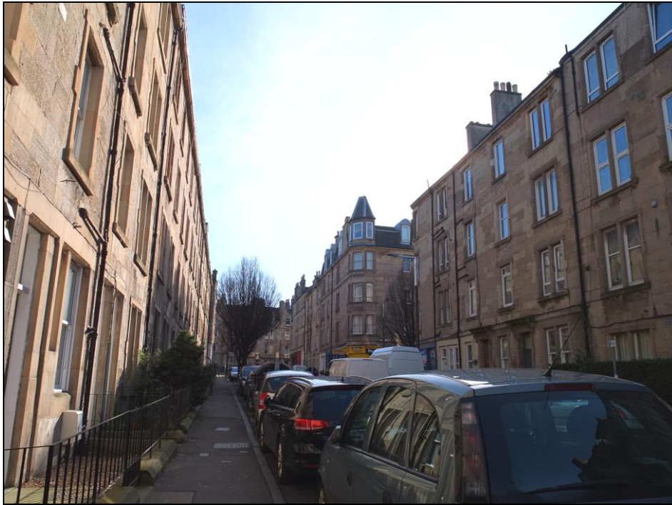
Figure 189: View of tenements in Fowler Terrace, from north, 2016 (DP232796 ©Copyright HES)
