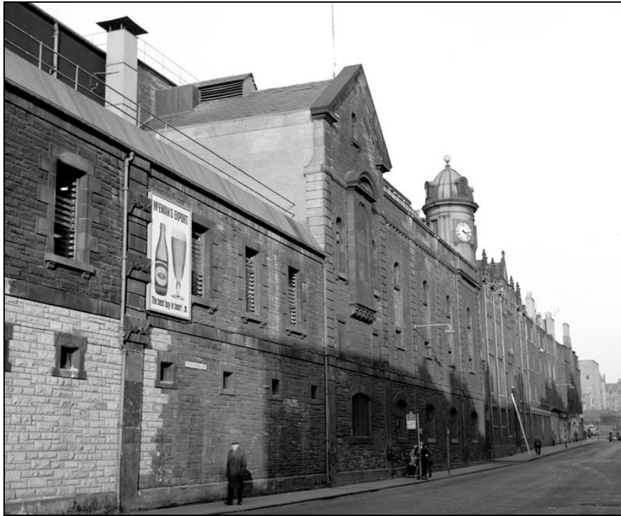
Figure 56: View of original Fountain Brewery buildings on north side of Fountainbridge, 1967 (copied 2000) (John R Hume Collection, SC590232 ©Crown Copyright HES)
