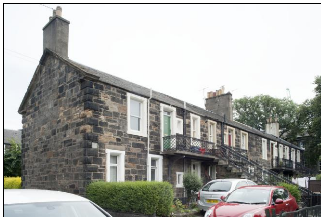
Figure 110: View of 17-24 Rosebank Cottages , from north-west, 2014 (DP203788 ©Crown copyright HES)
