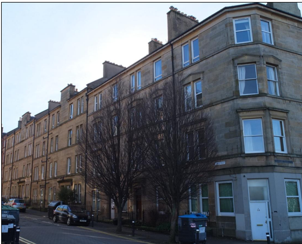
Figure 192: View of Tay Street , from north-east, 2016 (DP234218 ©Copyright HES)
