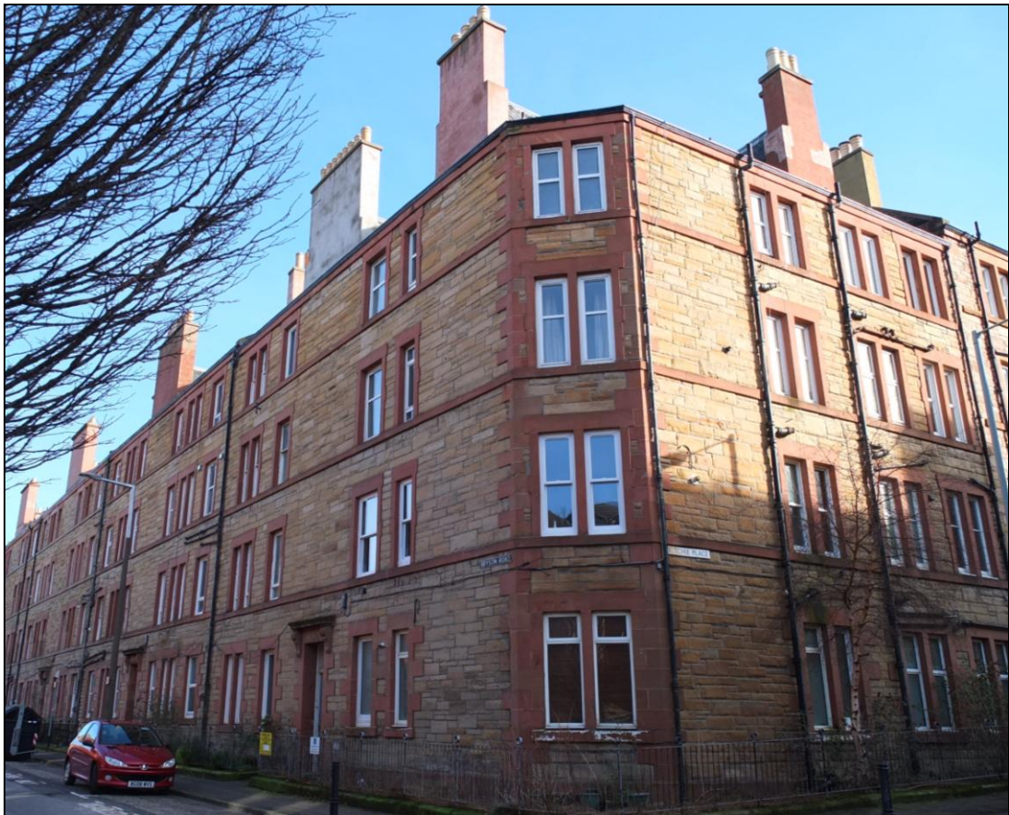
Figure 197: View of corner Bryson Road (left) and Ritchie Place (right), from west, 2016 (DP232769 ©Copyright HES)
