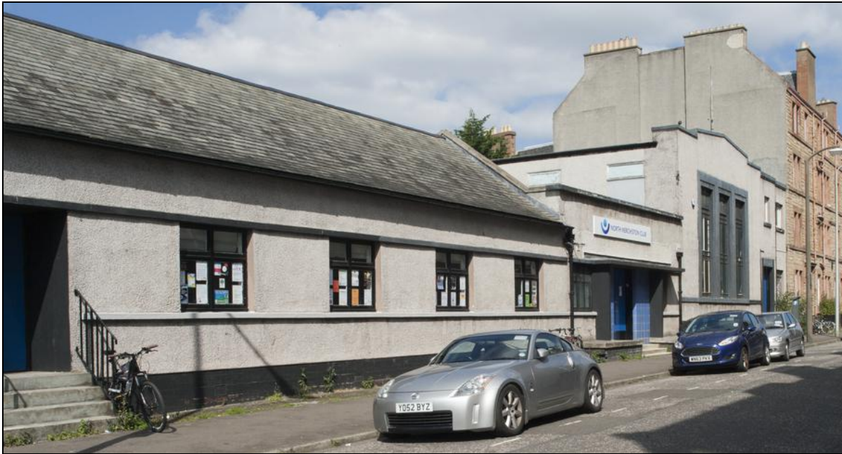
Figure 178: View of North Merchiston Club hall at west end of Watson Crescent, from south-west, 2014 (DP203087 ©Crown copyright HES)
