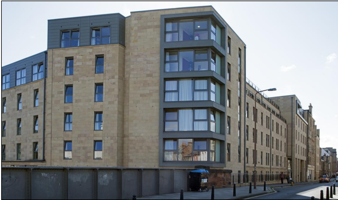
Figure 132: View of Grove Student Residences, 69 Grove Street , from north, 2014 (DP203702 ©Crown copyright HES)
