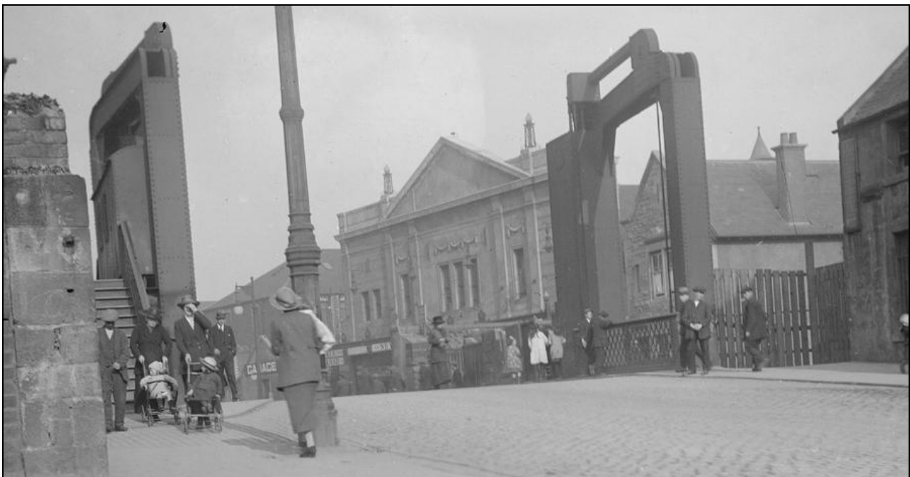
Figure 62: View of Fountainbridge elevation of Coliseum, 125 Fountainbridge , former iron foundry, 1906-30 (copied 2009) (Francis M Chrystal Collection, SC1131124 ©Crown copyright HES)
