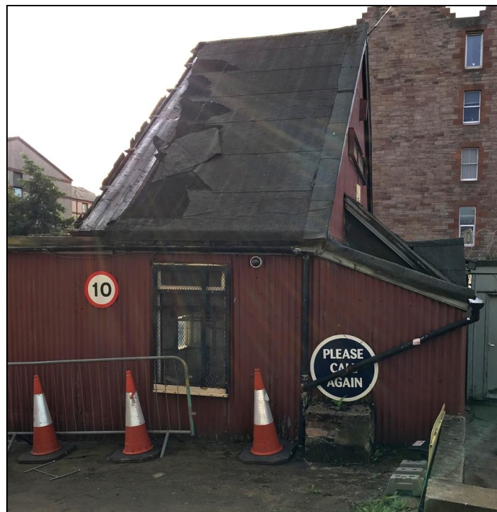
Figure 165: View of scrap merchants yard on Yeaman Place, from south, 2017 (DP260090 © HES)
