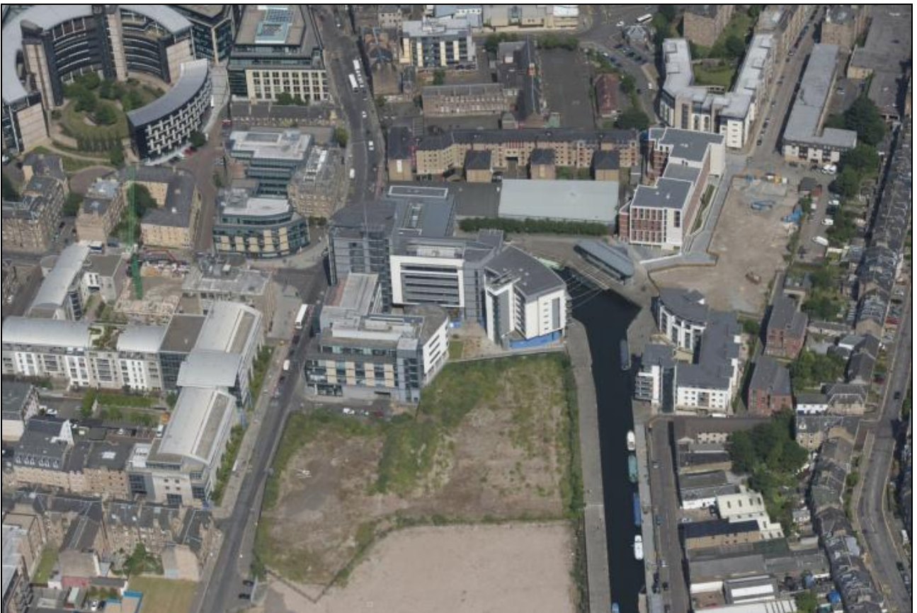
Figure 31: Aerial view of Union Canal, Lochrin Basin and Edinburgh Quay , from east-north-east, 2014 (DP193073 ©Crown copyright HES)
