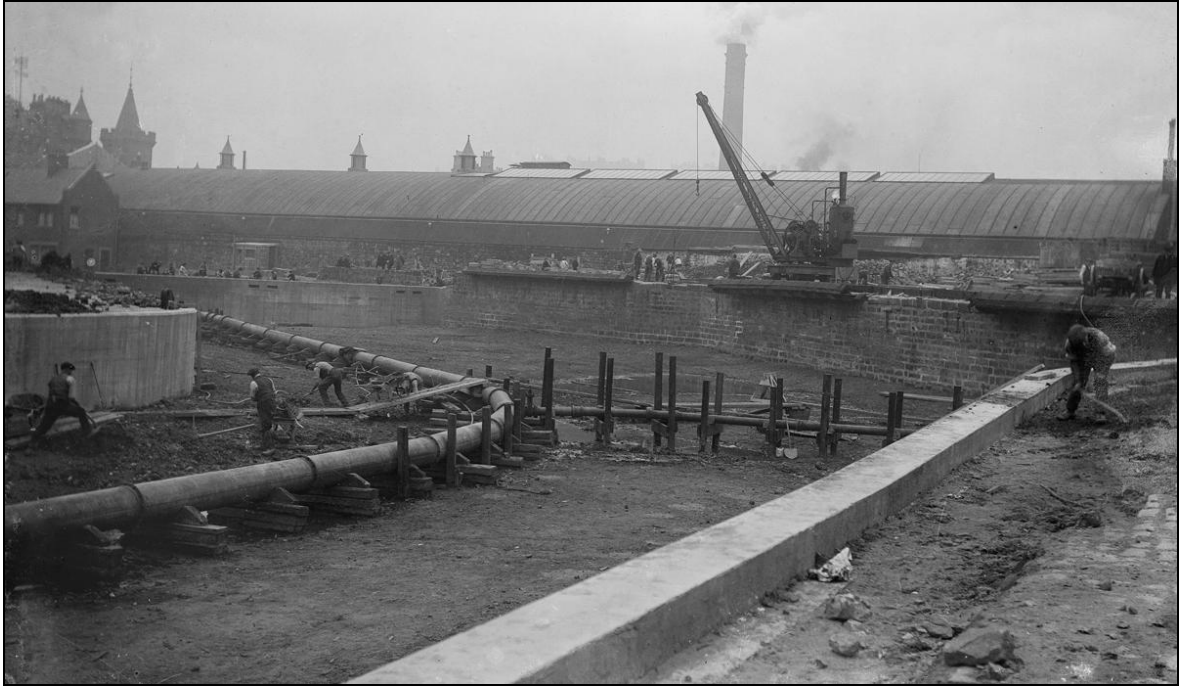
Figure 23: View of workmen blocking up and infilling Lochrin Basin , c.1906 (copied 2009) (Francis M Chrystal Collection, SC1130869 ©Crown copyright HES)
