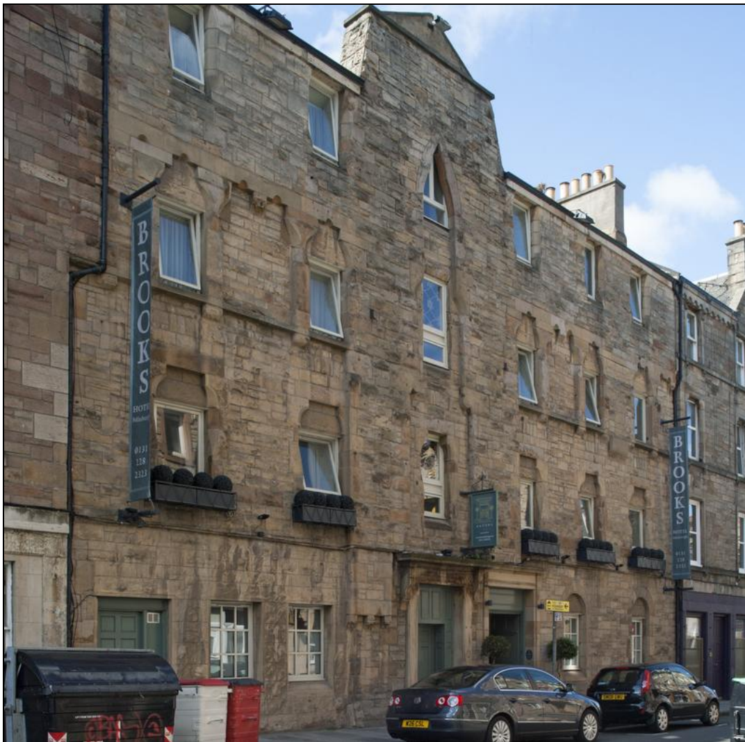
Figure 124: View of 70-76 Grove Street , from south-east, 2014 (DP204093 ©Crown copyright HES)
