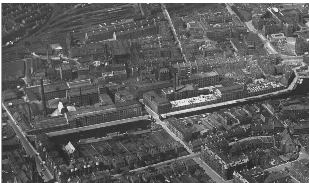
Figure 73: Aerial view showing Castle Mills alongside the Union Canal, with the southern block under reconstruction, 1929 (copied 2014) (Aerofilms Collection, SC1452001 ©Crown copyright HES)
