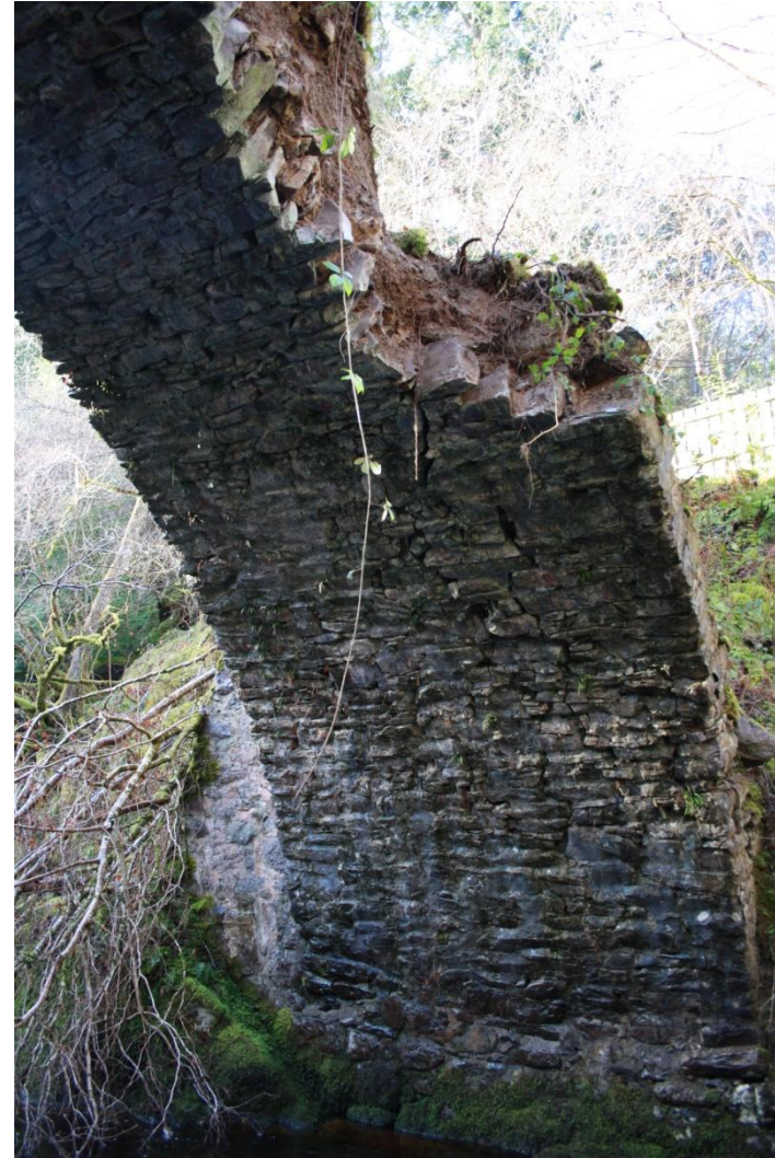
Plate 6: View of the arch from the NW.
