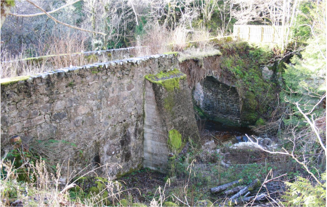
Plate 1: General view of the bridge from the NW.
