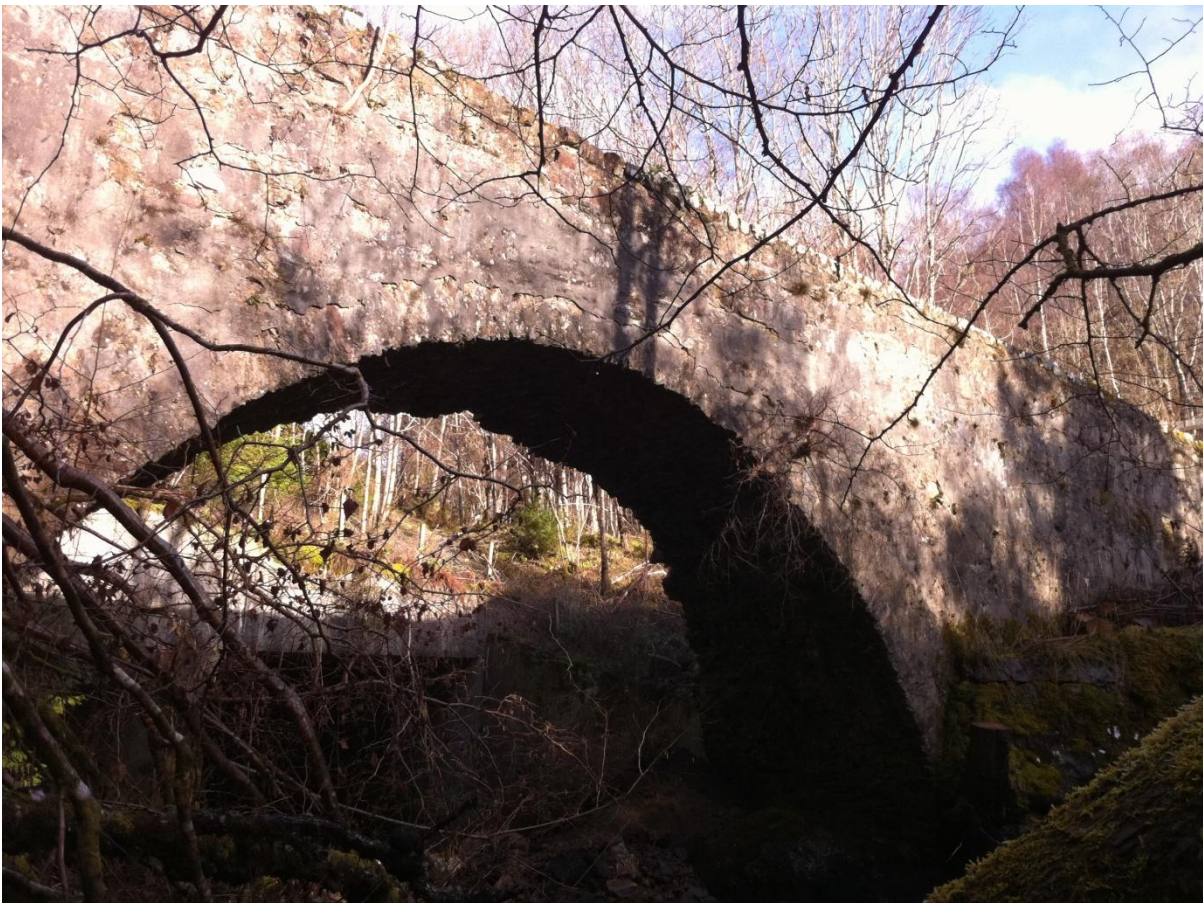
Plate 8: General view of the arch from the SE.
