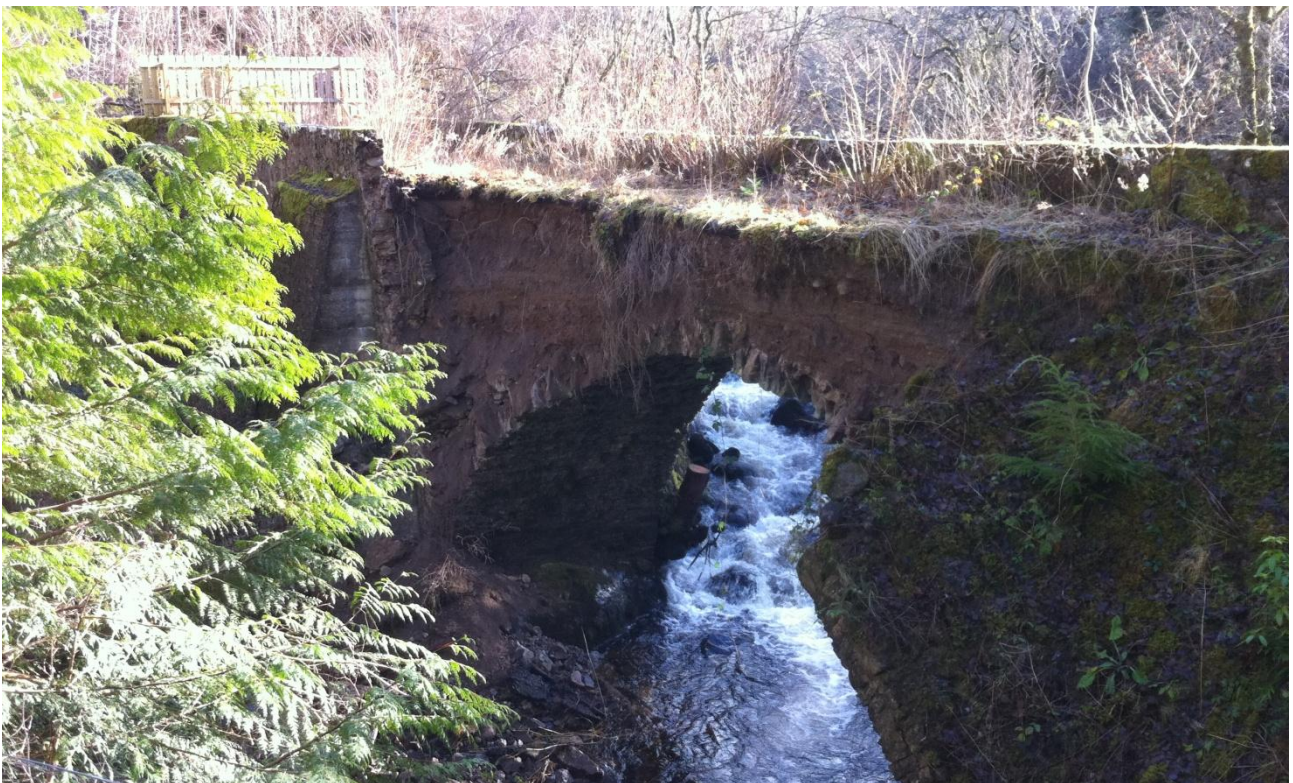
Plate 2: General view of the bridge from the SW.
