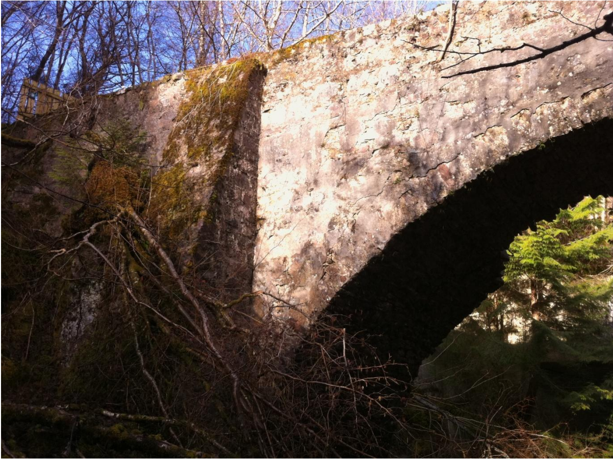
Plate 9: View of the SE buttress from the NE.
