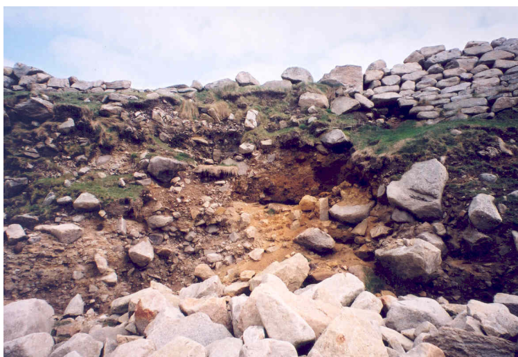
In 2003 the overhang has collapsed with further loss of vegetation
