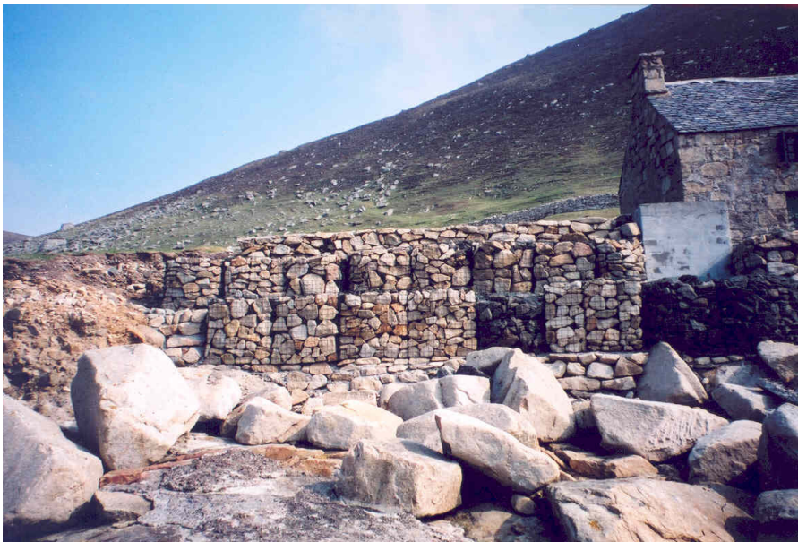
Coastal erosion Section C – 2003 (STK03 3/9) The repaired gabion baskets
