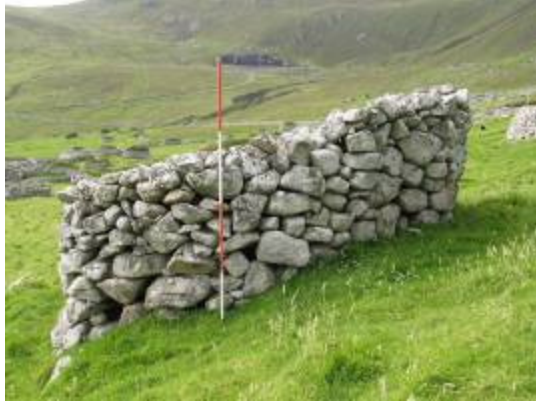
Planticrue (P-03) located within head dyke
