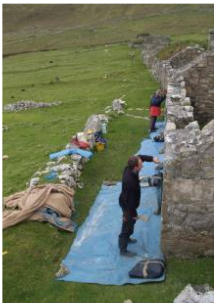
Lime pointing the façade of House 12
