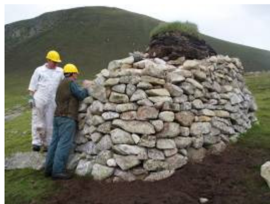
Cleit 168 being repaired by drystane dyker and Work Party member
