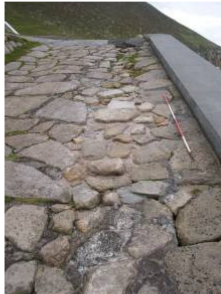
Jetty slipway after repair
