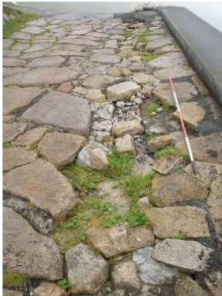
Jetty slipway before repair
