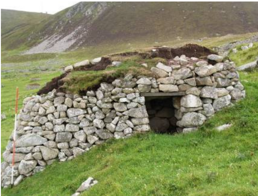
Heavy erosion of turf on cleit 15
