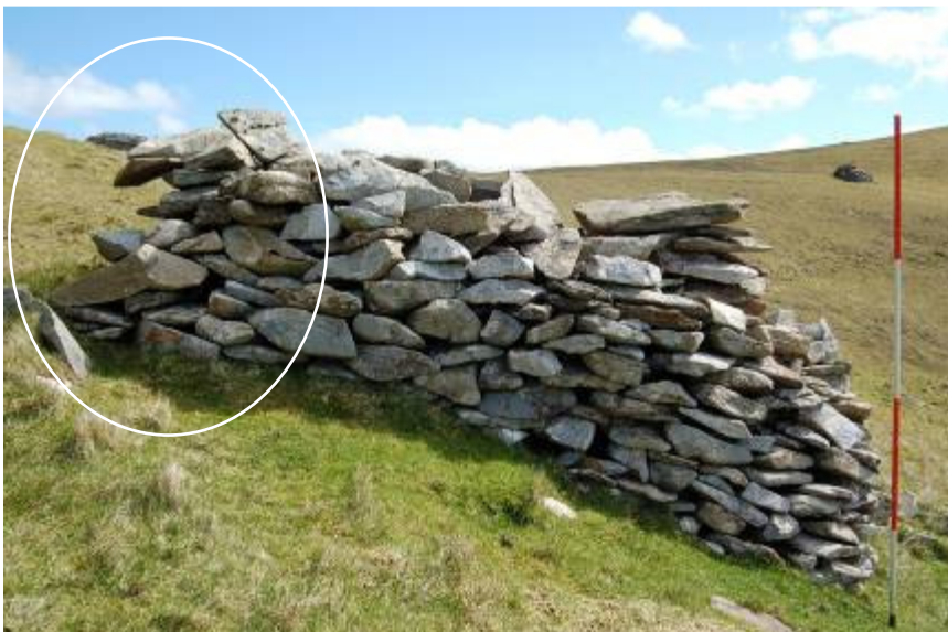
Major collapse to Cleit 486. Stones have fallen at the left-hand side of the photo.
