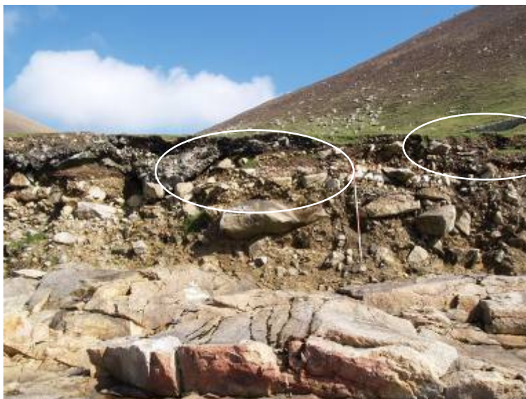
Same section in 2007 showing two areas of erosion caused by sheets of water running off the hills
