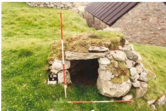
Figure 12 Cleit 26, with collapsed roof above compared with 1996
