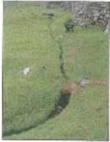
Clearing street drain
