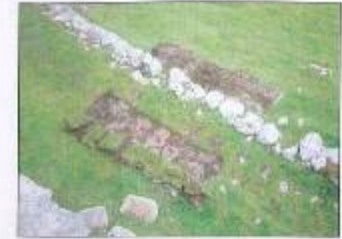
Reparatory work by D14.7
