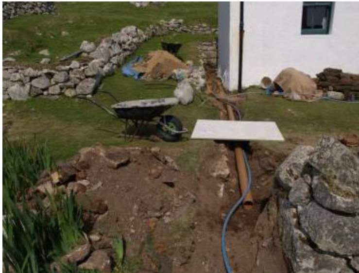
Figure 15a - Factor's House drainage – inserting Pipe 1, facing north-east
