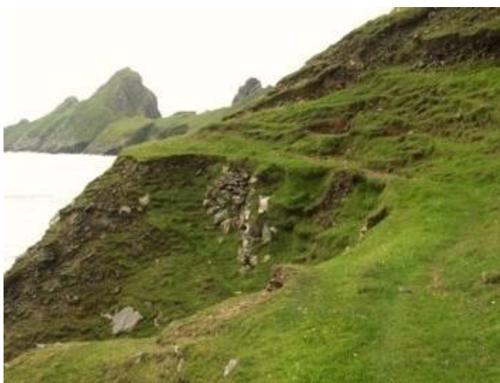
Figure 10 – Revetted track to Ruaival
