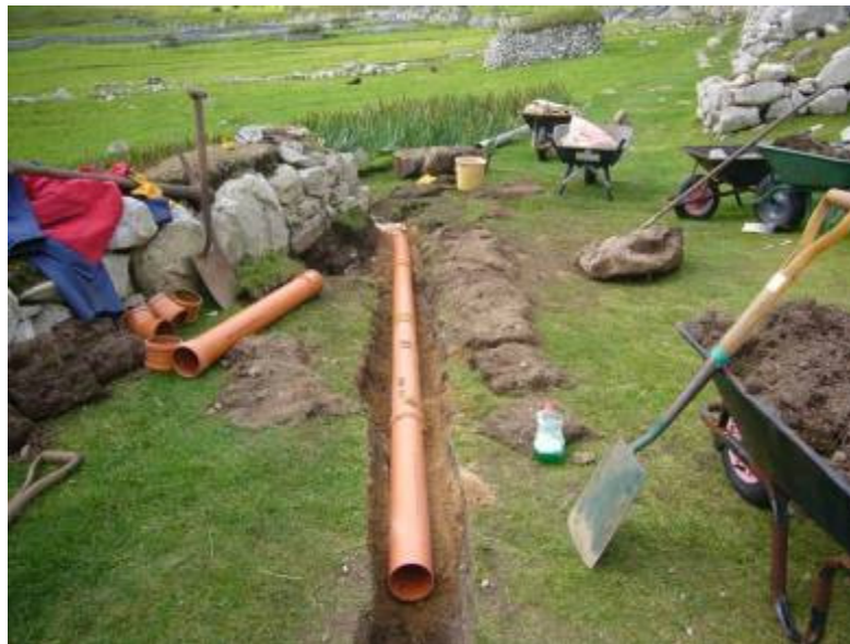
Figure 15b - Factor's House drainage – inserting Pipe 2, facing west
