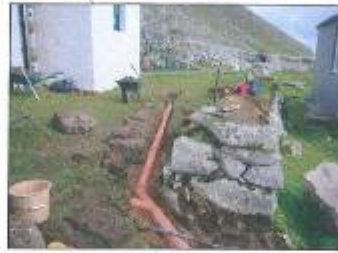
Upgrading and improving drain at the factory house
