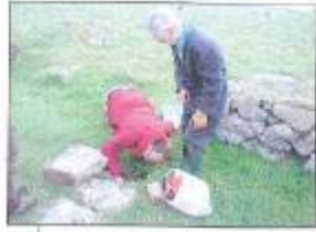
Clearing the gully drain at 1115
