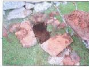
Clearing the fire drain at 1162 house B
