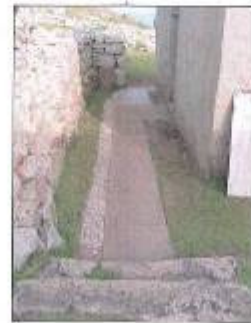
A new ditch of the church
