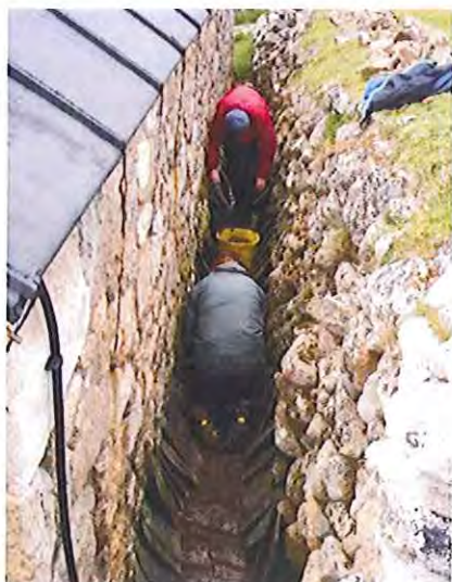
Clearing out the soak-away along the rear of House 6 and the completed task
