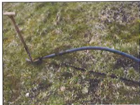
Cutting the visible cable within the Head Dyke, and revealing the cable up towards the hill-top radars
