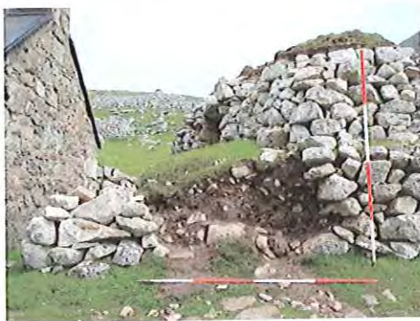
Repairing the revetment wall by the streets between House 2 and cleit 28
