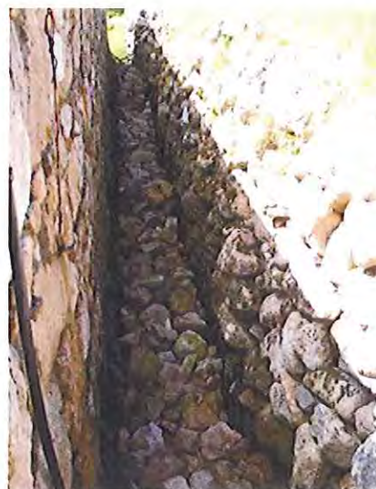
Clearing out the soak-away along the rear of House 6 and the completed task
