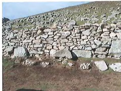
Repairing the Head Dyke behind the MacKenzie Slabs, before and after
