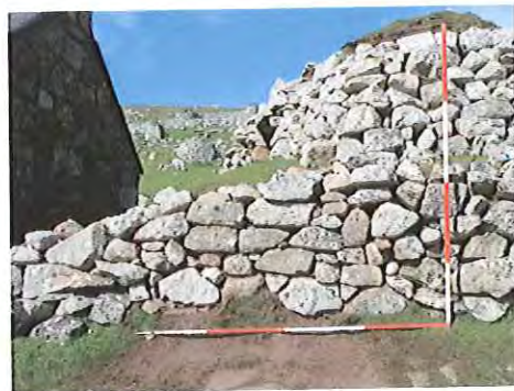
Repairing the revetment wall by the streets between House 2 and cleit 28
