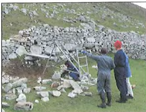
The repair work to the Head Dyke near cleits 4 and 5, during and after
