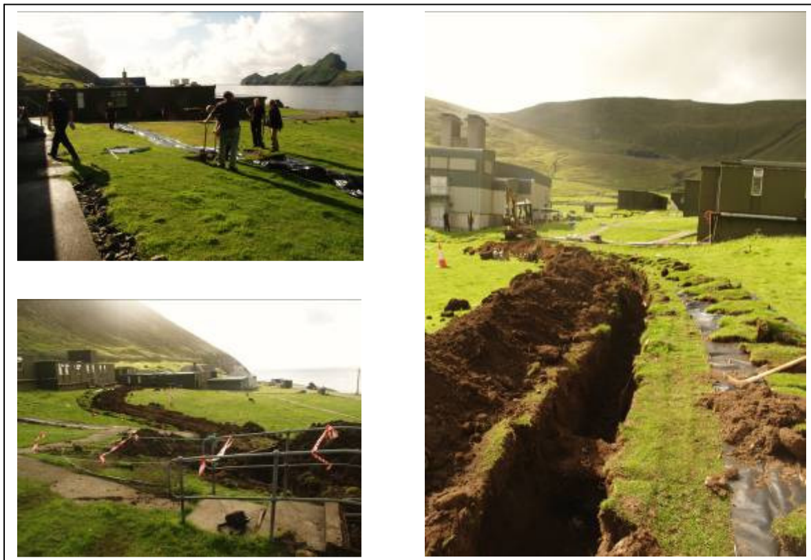
Figure 8: The trench being excavated
