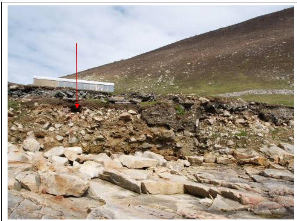
Figure 2b: Photograph CEP 15, area C with missing stone, 2010
