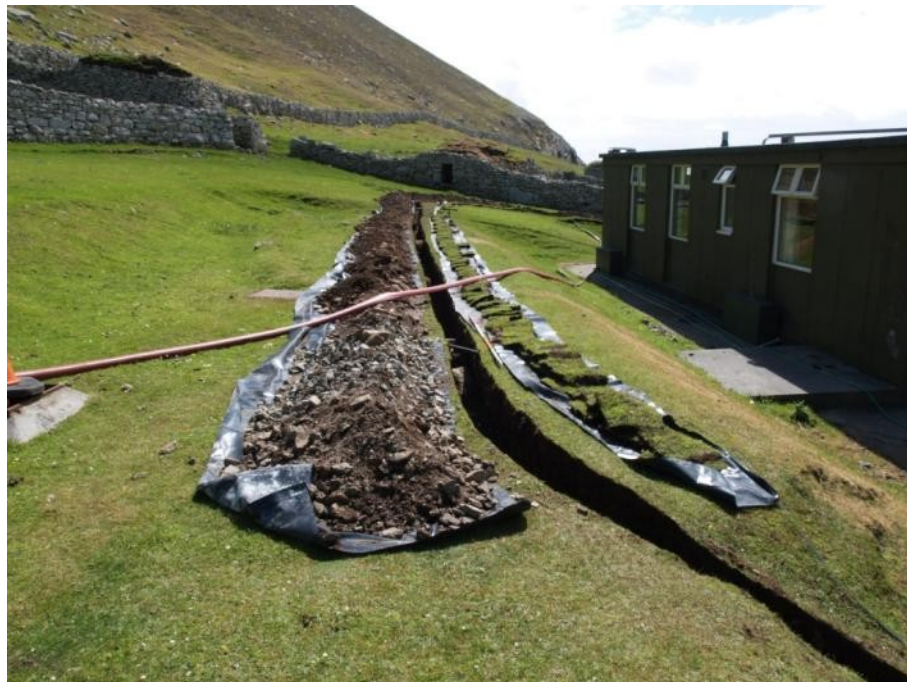
Figure 18. The pipe trench after excavation, looking south east
