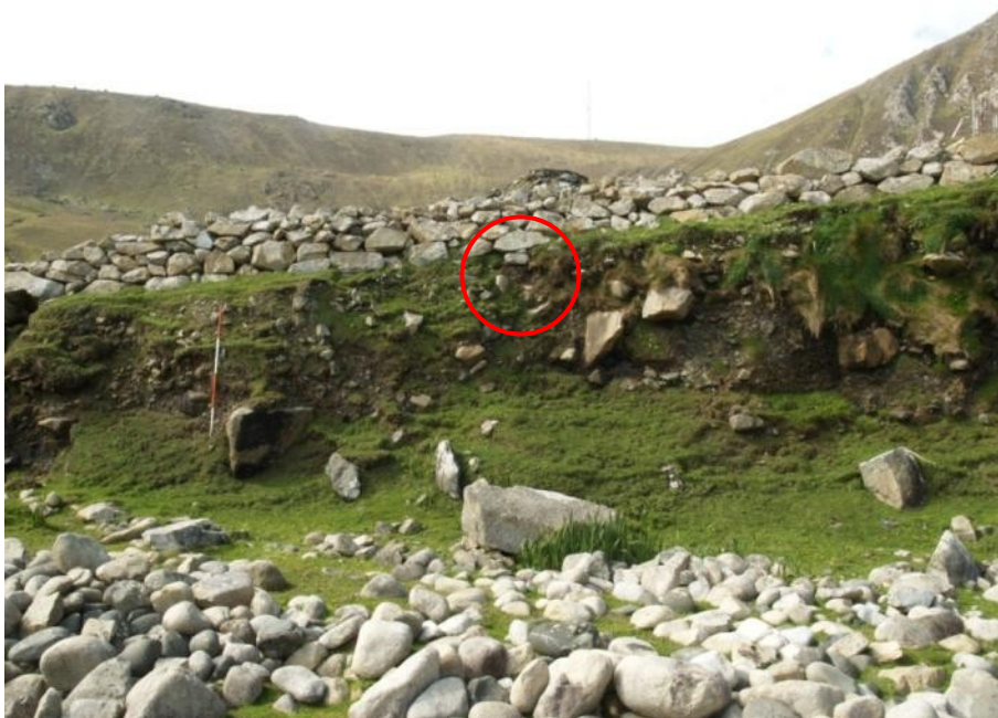
Figure 9. A stone near the base of the Sea Dyke in Section H has been lost between 2011 (top) and 2012 (bottom)
