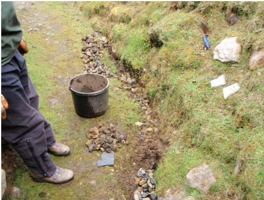
Figure 2. Clearing out the drain by the Munitions Store
