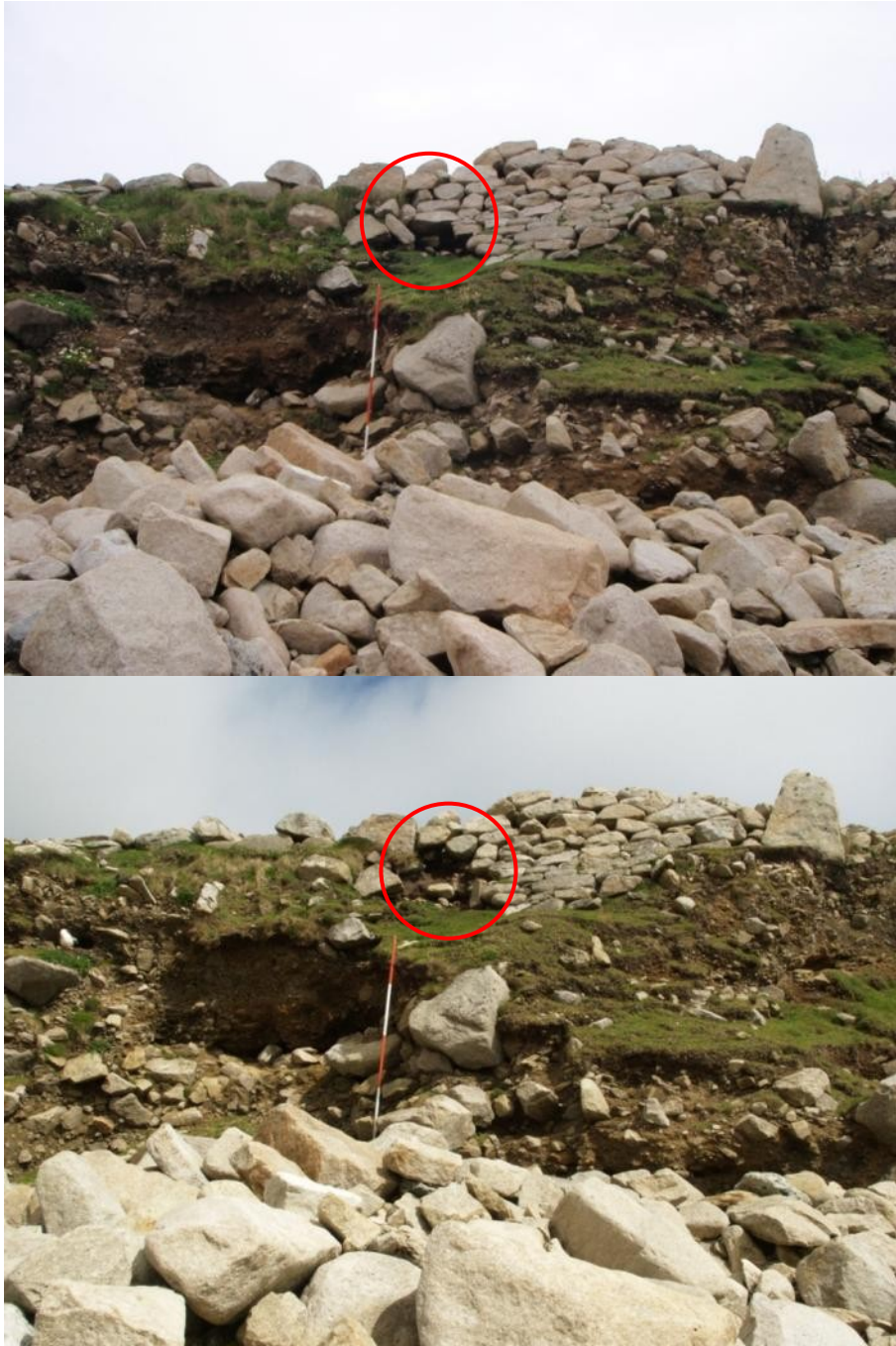
Figure 8. Part of the Sea Dyke in Section E has been lost between 2011 (top) and 2012 (bottom)
