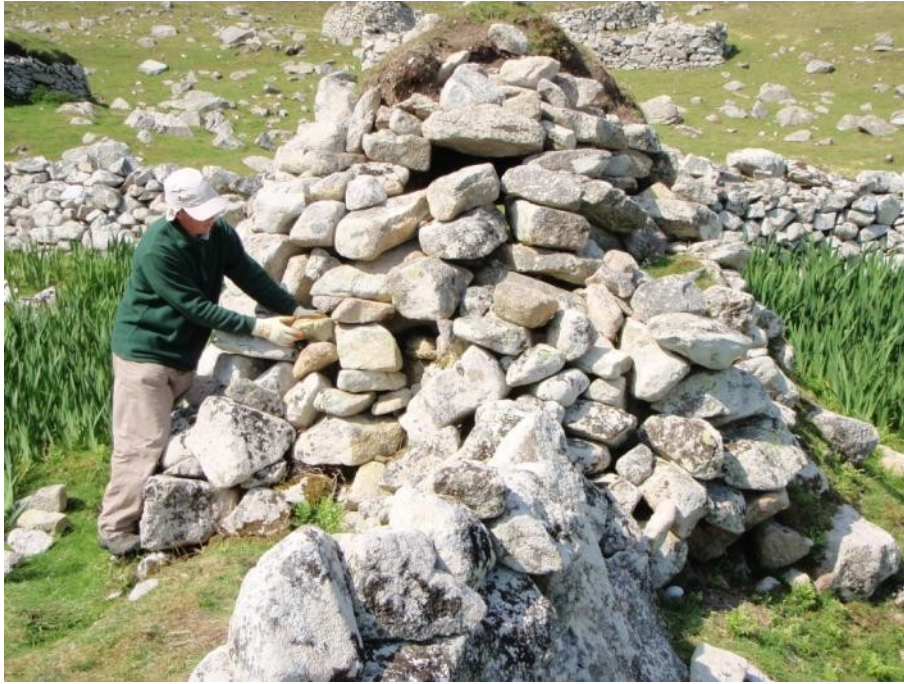
Figure 1. Repairing a cleit wall
