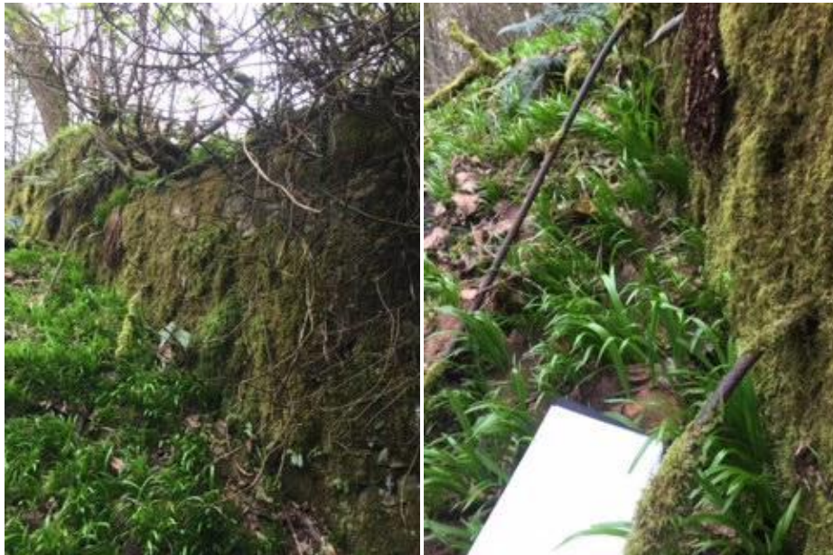
Illus 19: Retaining wall for the upper terrace; illus 20: Winding mechanisms for glasshouses.
