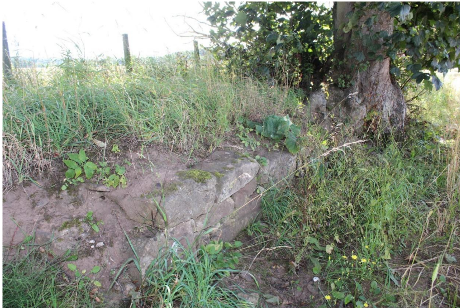
Illus 32: Dressed stone dyke along the Riverside Pleasure Walk.
