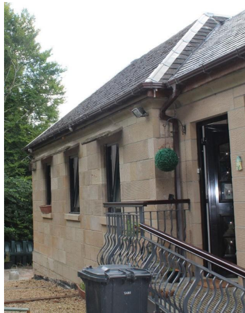
Illus 25: The rebuilt East Lodge; the central window replaced the front door of the original building.
