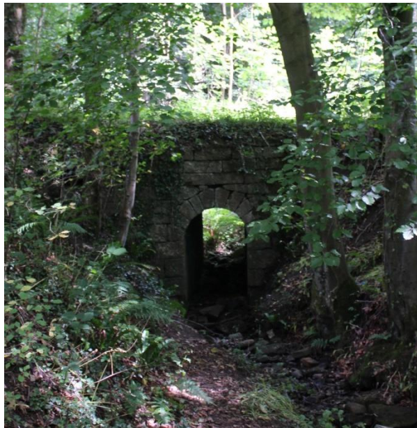
Illus 27: A stone bridge and culvert taking East Drive over a burn in Highmainshead Woods.
