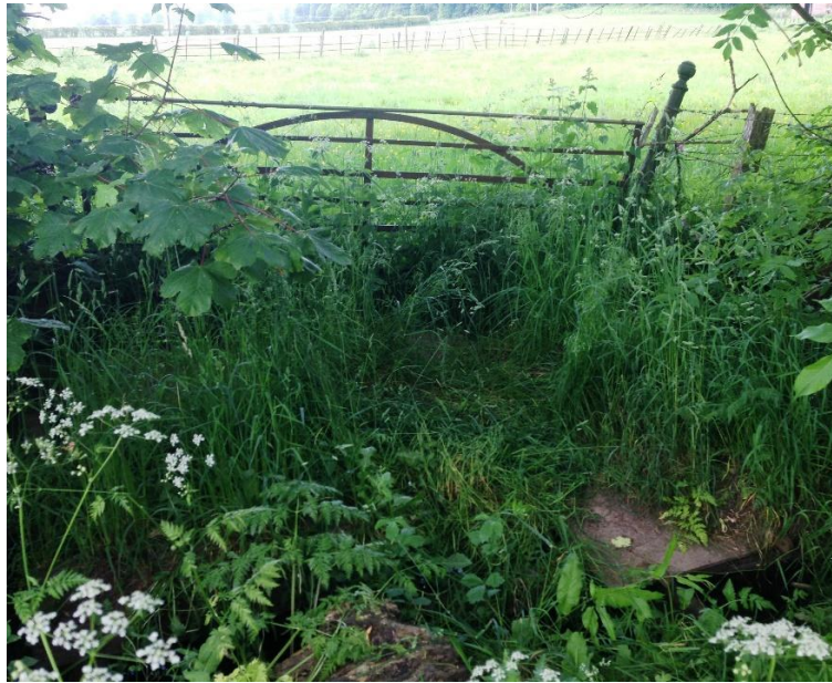
Illus 18: The remains of an iron gate and bridge over a burn between the gardens in front of the Estate Offices and the former walled garden.
