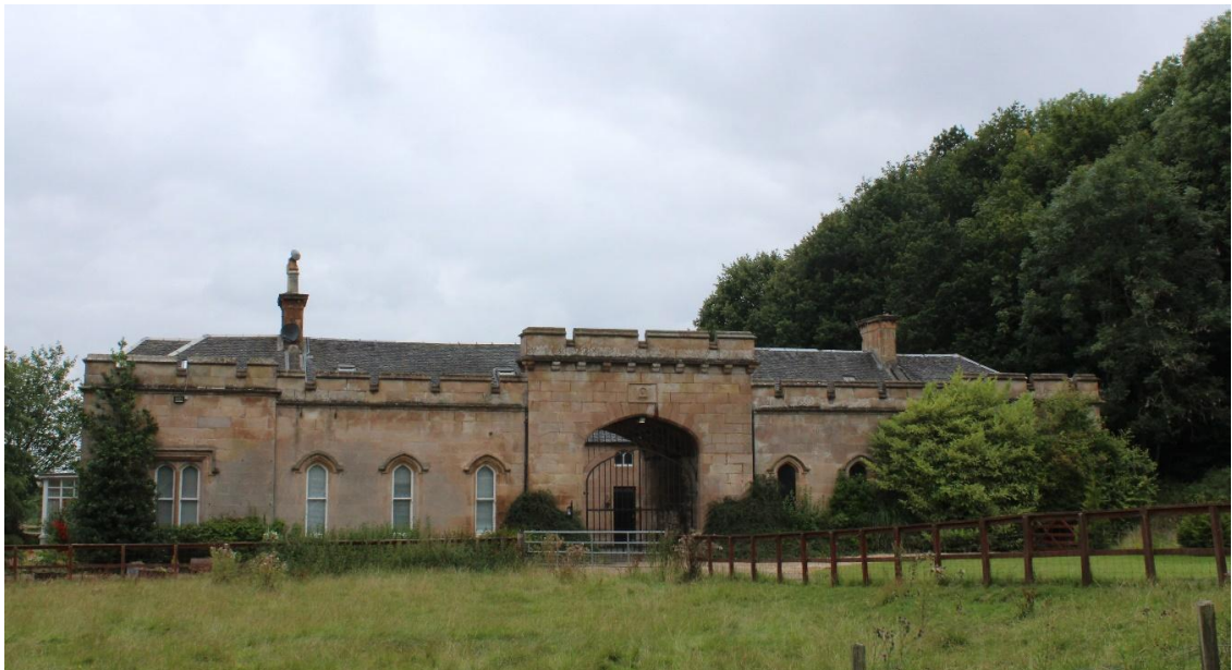
Illus 21: The east elevation of the Offices & Stables.
