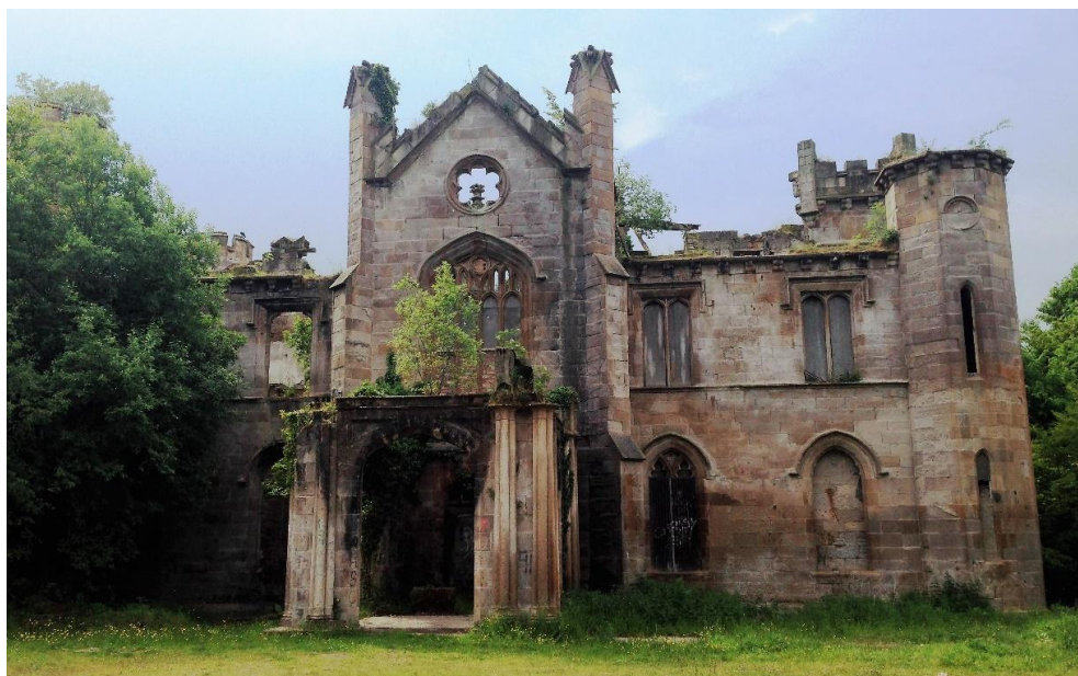
Illus 33: The north elevation of Cambusnethan House and the porte-cochère .
