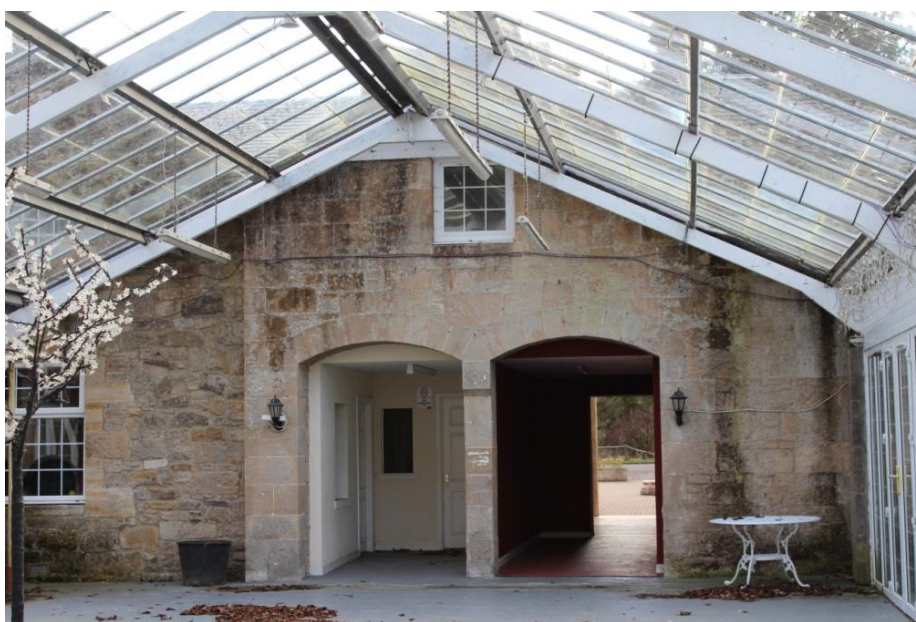
Illus 16: Interior of the Courtyard Stables, showing north-facing wall with reconstructed archways under the modern glass and steel canopy.
