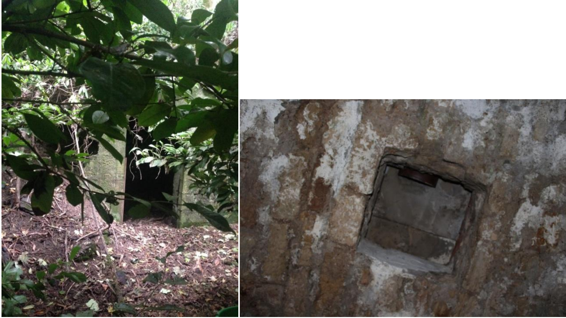
Illus 32: The Gasometer's exterior and interior roof (from the north and below).
