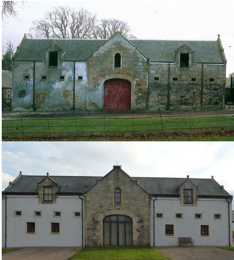
Illus 16: The stable block in the Home Farm Complex, before and after conversion.
