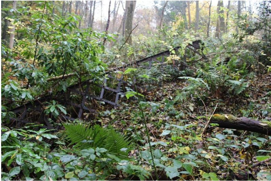
Illus 17: Collapsed remains of iron bridge in the Ram's Gill ravine.
