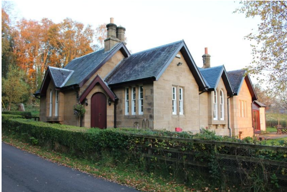
Illus 24: Early lodge along the North-east Drive.
