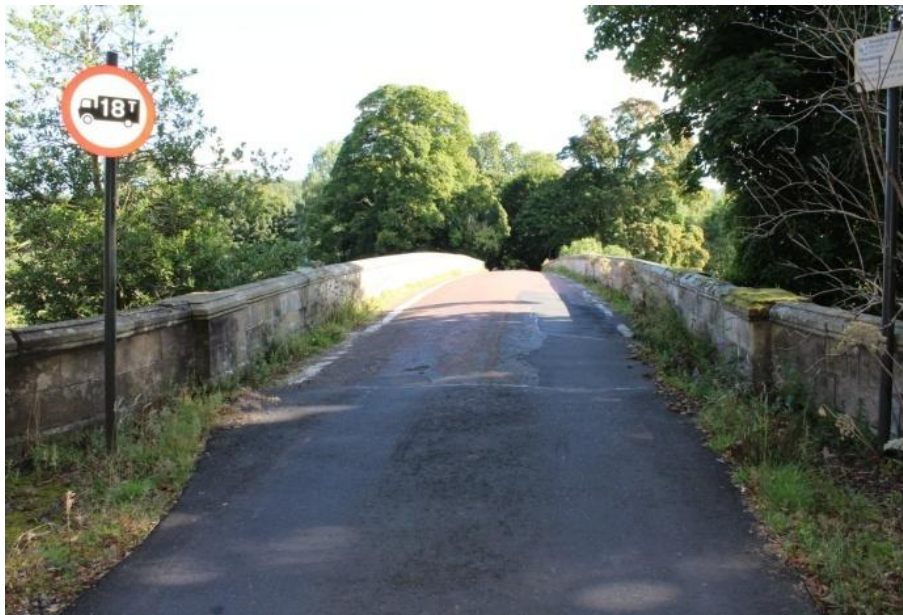
Illus 27: Mauldslie Bridge.
