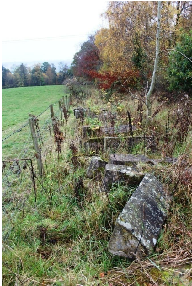
Illus 19: Dismantled remains of former gate structure near Mauldslie Kennels.
