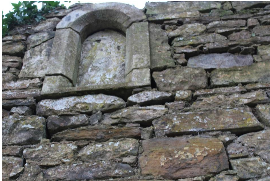
Illus 41: Burnetholm Cottage - decorative stonework detail of window on the south facing facade.
