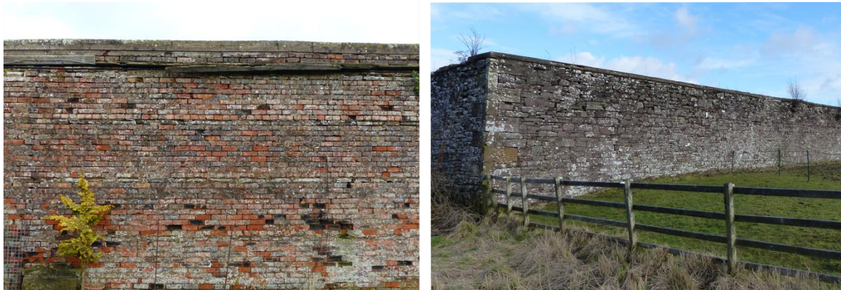
Illus 34: Typical interior brickwork (left image) and external stonework (right image) of the Walled Garden.
