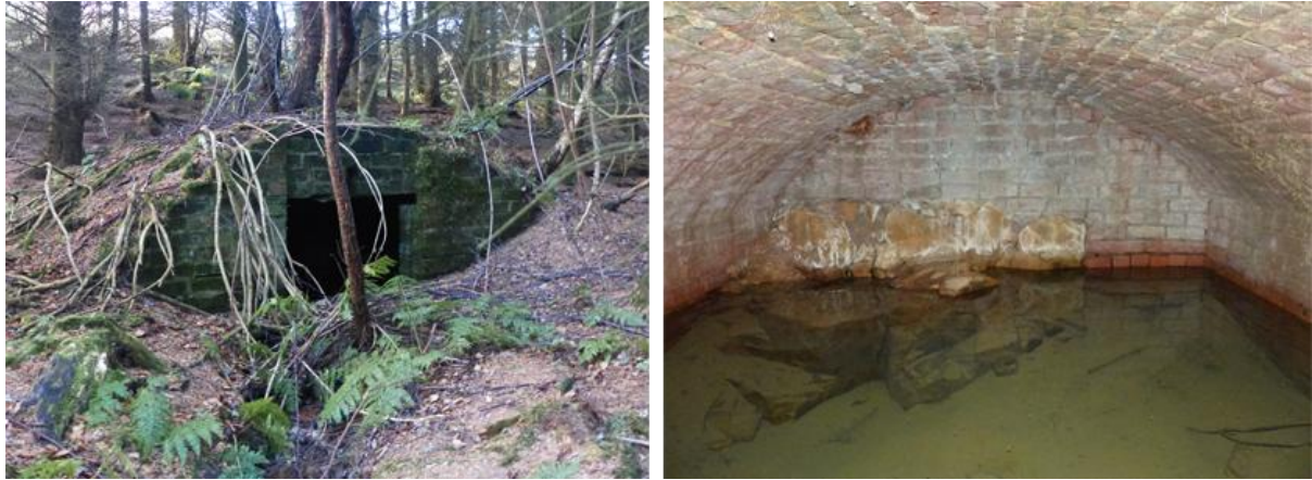
Illus 54: Water Tank 2: Left: Exterior view; Right: Interior
