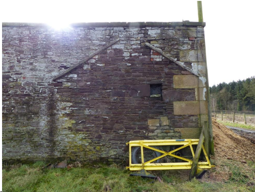
Illus 38: Outline of the small building at the west end of the north side of the Walled Garden's north wall.
