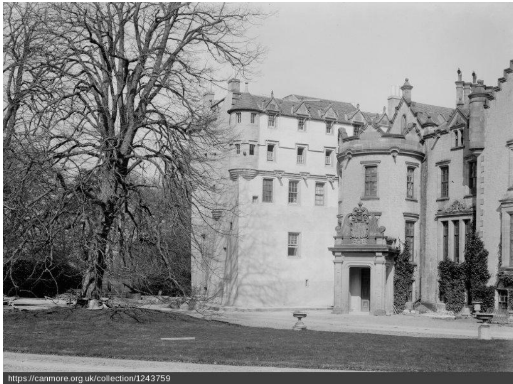
Illus 17: Stonebyres House looking north-east towards the front entrance, c 1890. (from Canmore https://canmore.org.uk/collection/1243759 ).
