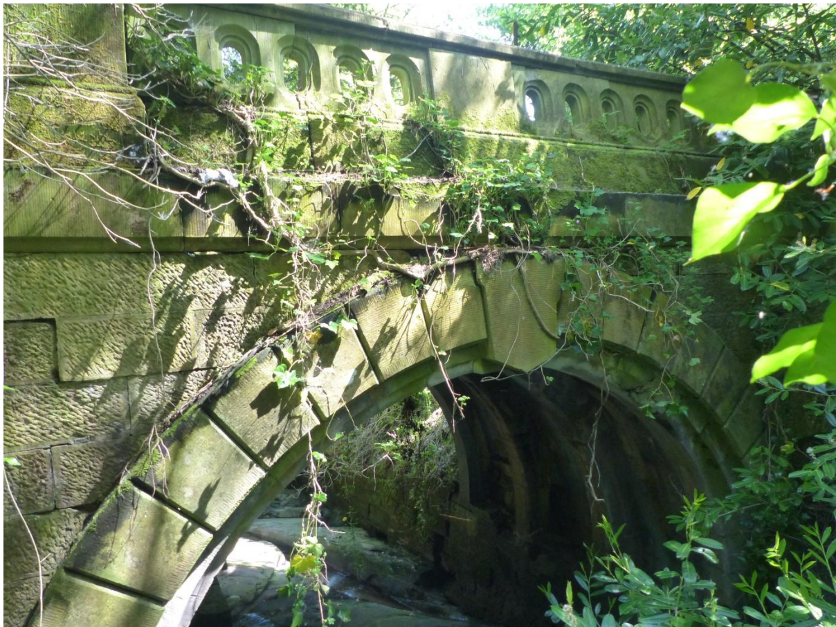
Illustration 29: The upstream face of the bridge across Stonebyres Burn (looking north-east).
