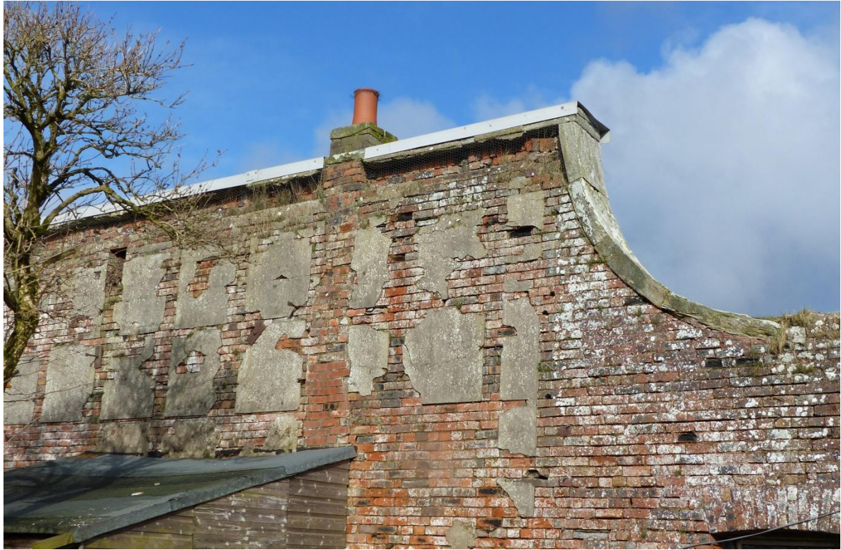
Illus 37: Details of the south-facing interior wall of Stonebyres walled garden.
