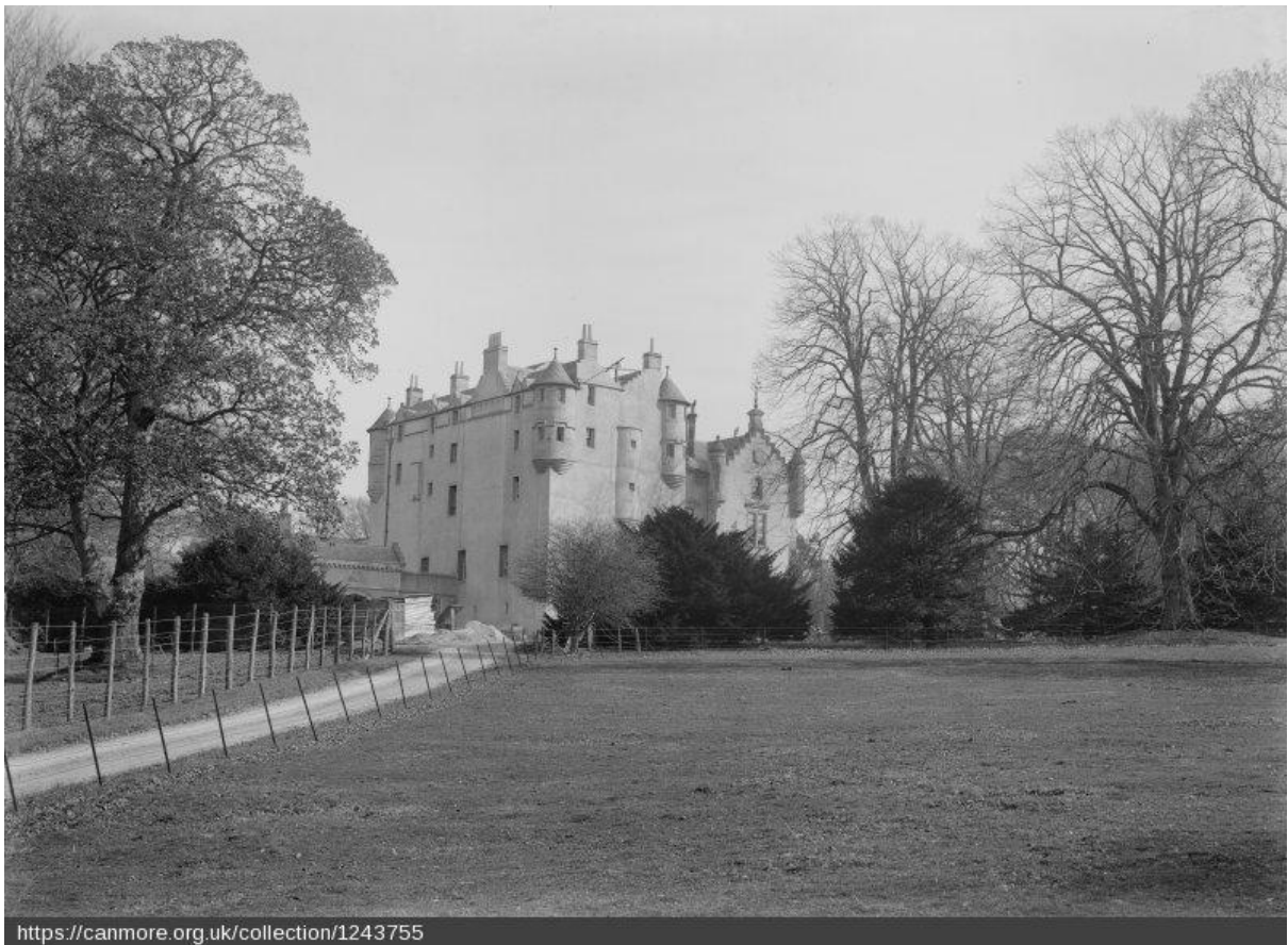
Illus 20: View of Stonebyres House looking SSE, c 1890. (Canmore, https://canmore.org.uk/collection/1243755 ).
