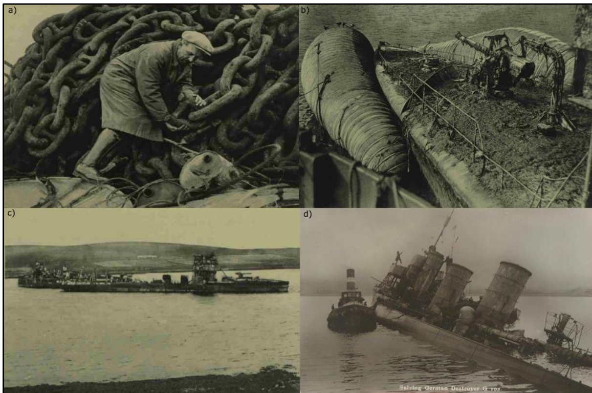
Plate 1 a) The chain that snapped in the first lifting attempt on V70 in July 1924 (Illustrated London News) b) Salvage operations on S131 by ScapaFlow Salvage & Shipbreaking Company (Illustrated London News) c) Salvaged destroyer lying in Cox & Danks 'boneyard' at Mill Bay, Hoy (Illustrated London News) d) Postcard showing salvage operations on G102 by Cox & Danks (courtesy Kevin Heath)
