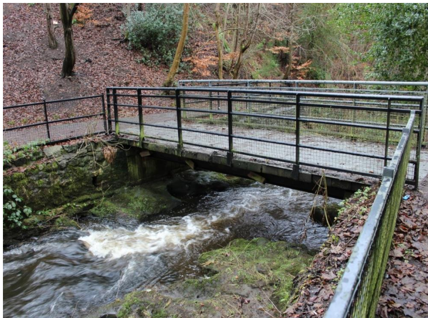
Illus 14: Footbridge at the upper waterfall near the south-west entrance.
