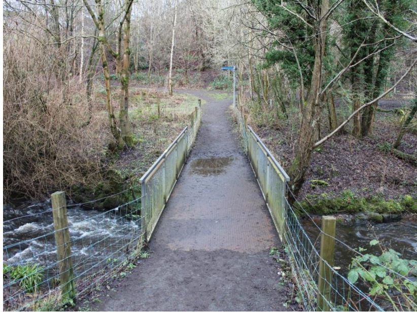
Illus 19: Footbridge towards the north end of glen.
