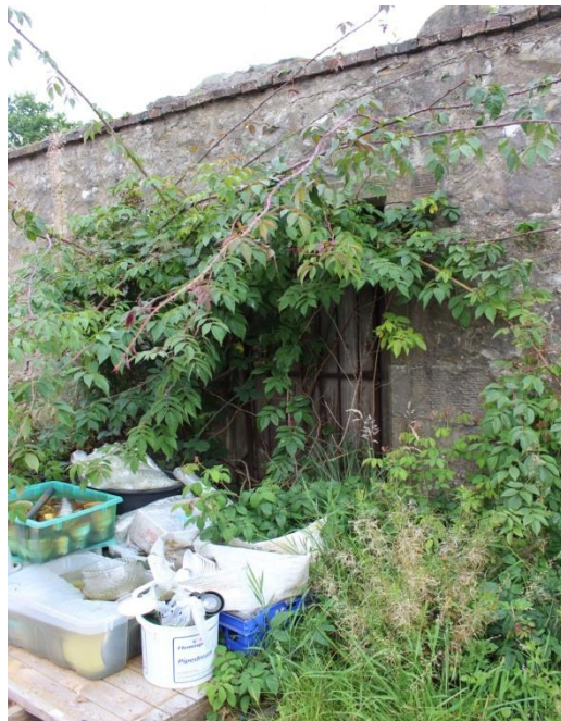
Illus 19: Overgrown door into walled garden.
