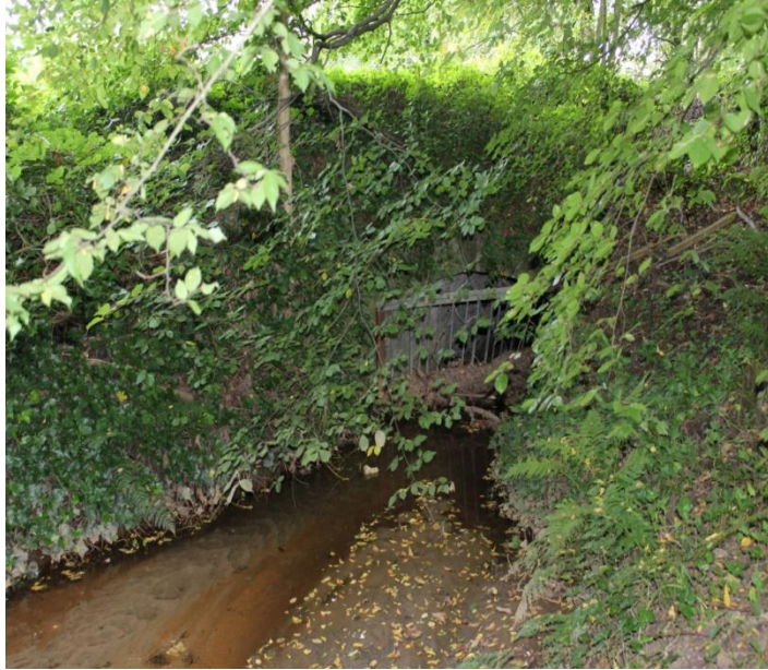
Illus 20: Arched bridge over burn.
