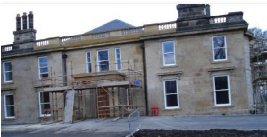
Illus 19: Larbert House under renovation.
