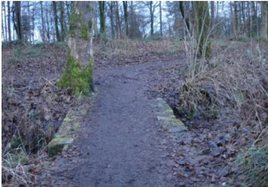
Illus 20: Footbridge over the ditch that leads towards the Walled Garden.
